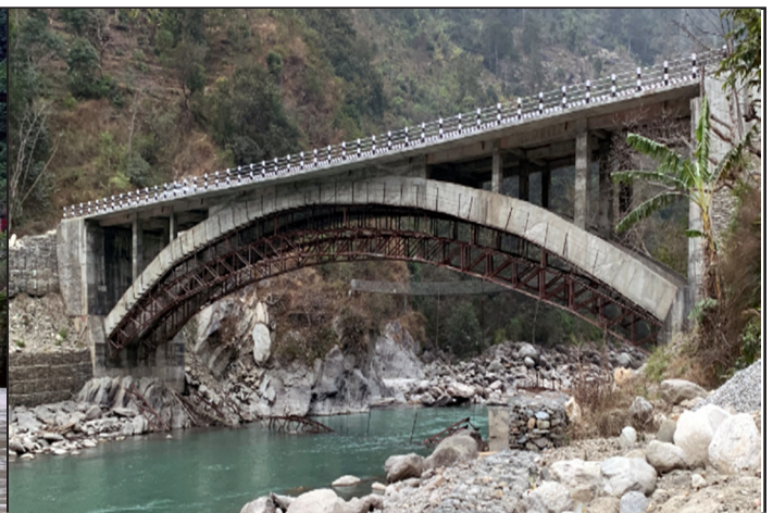
Arch bridge over Tamakoshi River at Gumu, Dolakha (60m span)
