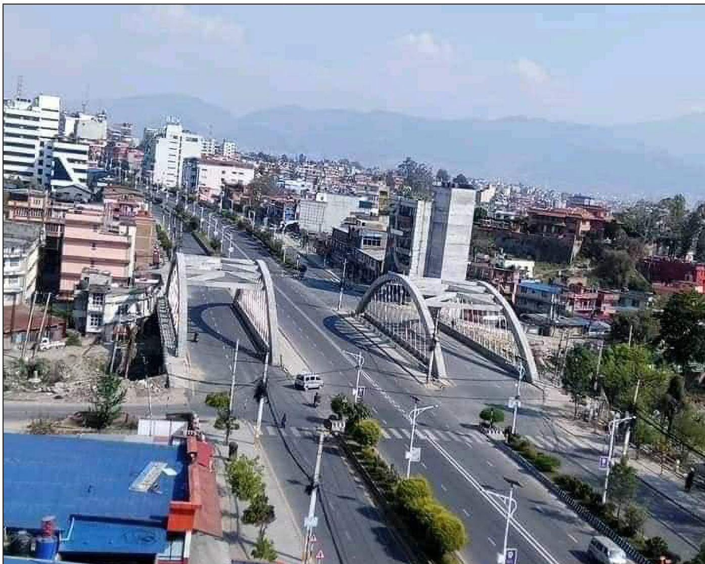
Dhobikhola Network Arch Bridge, Kathmandu (50m span)
