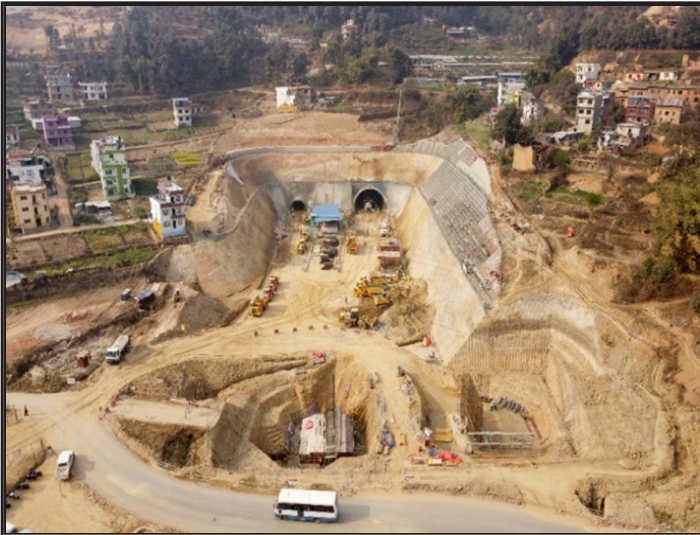
(a) Main Tunnel, East
