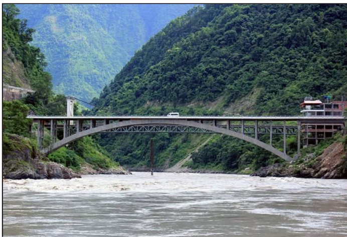
Mugling Arch Bridge (120m + 2 * 20m)
