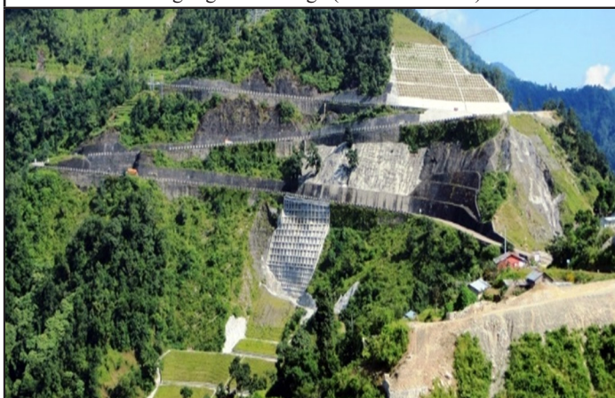
Slope Stabilization work at BP highway
