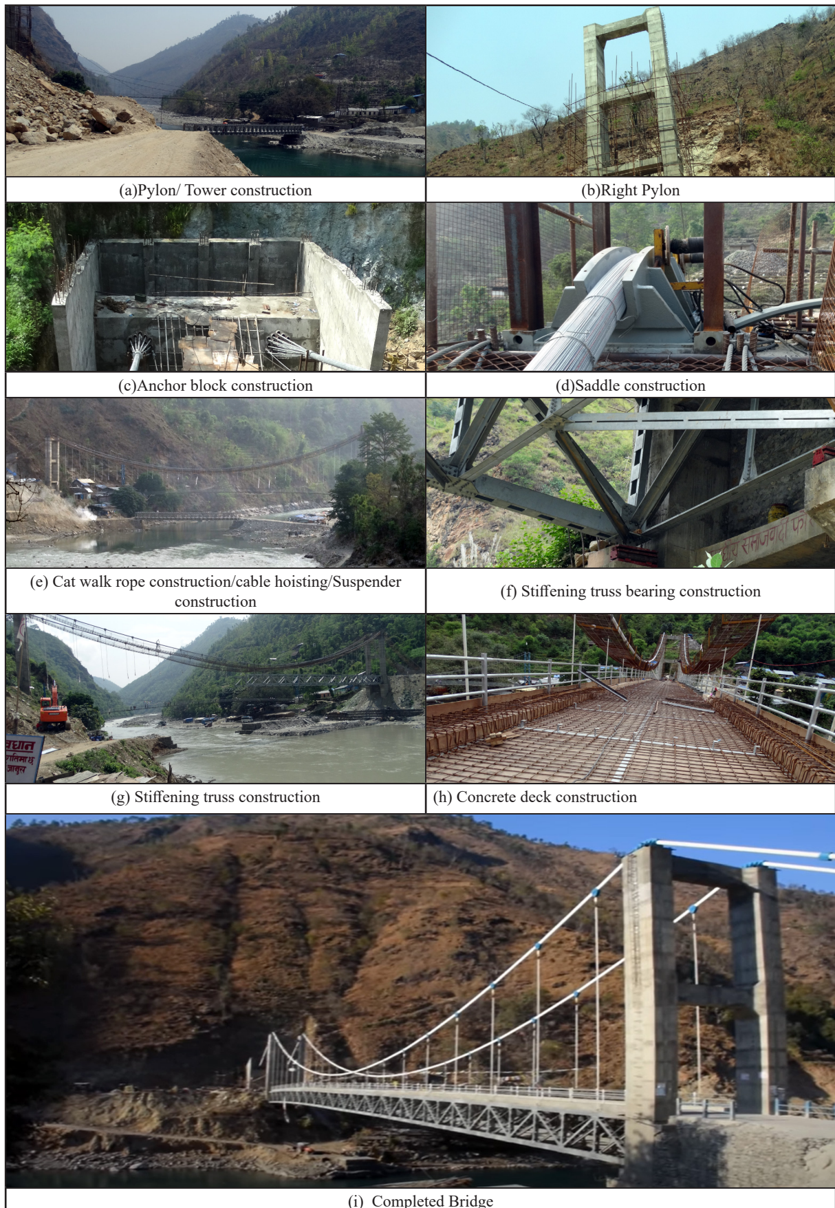
Fig.4- Bridge Construction Sequence
