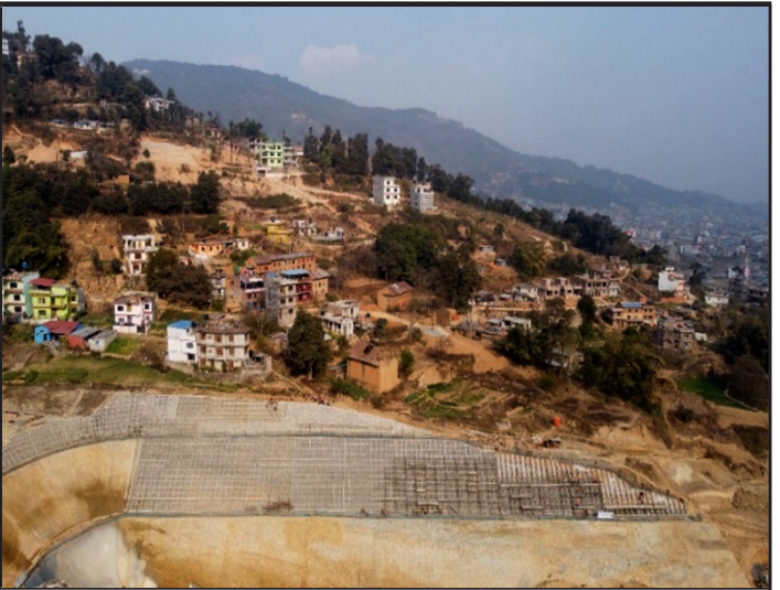
(b) Crib Wall, East
