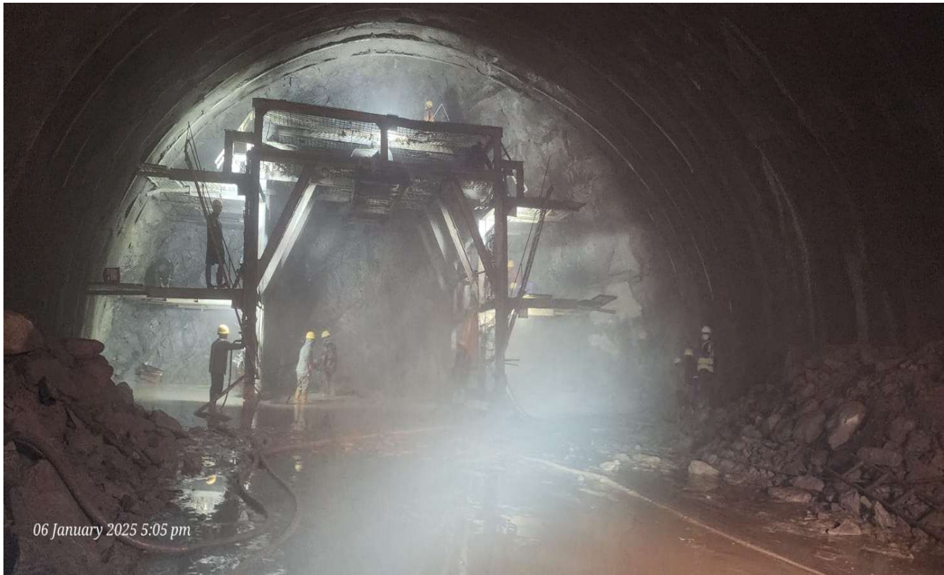
Fig: During Drilling of hole to load explosive material for Blasting
