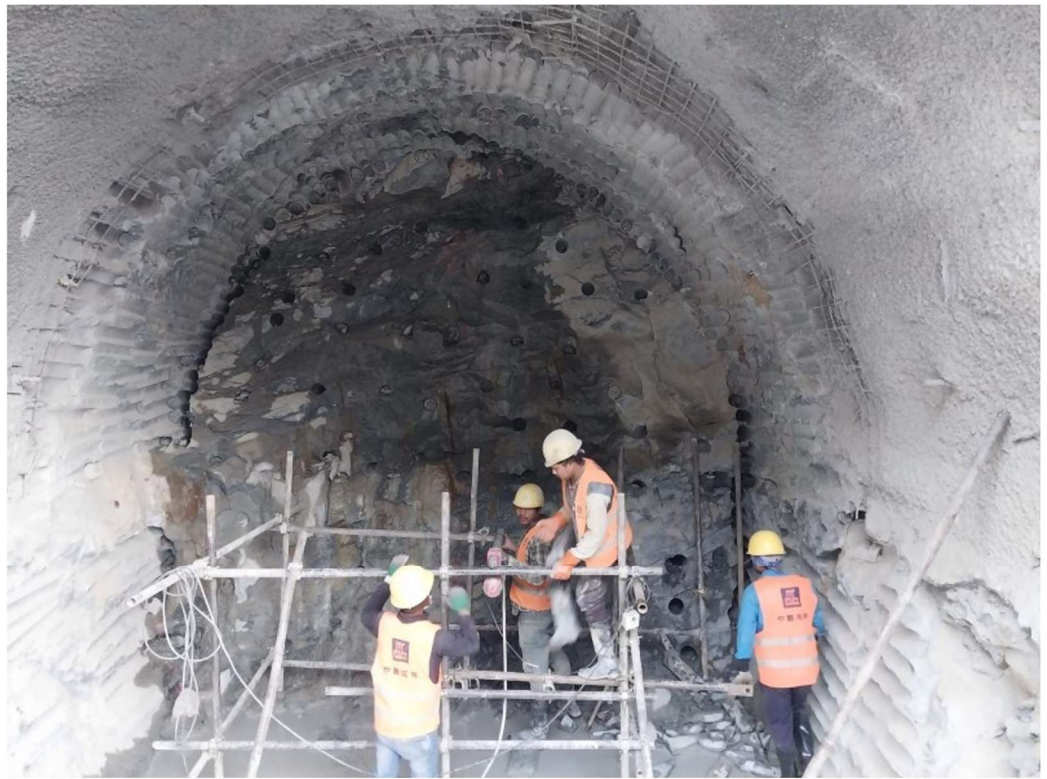
Fig: During core cutting for excavation of Rock in Bypass 2 Tunnel
