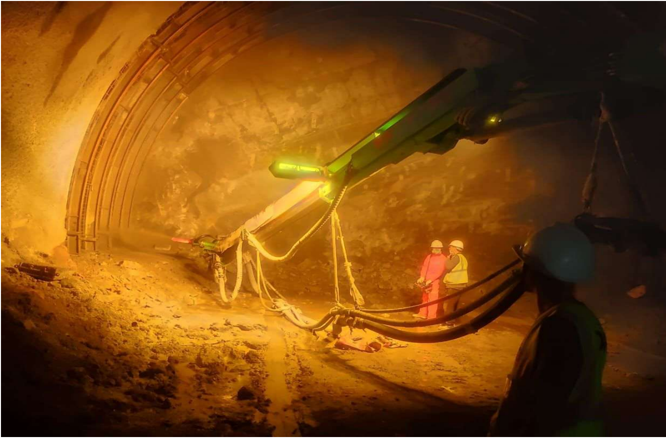
Fig: Shotcreting Works at North Portal
