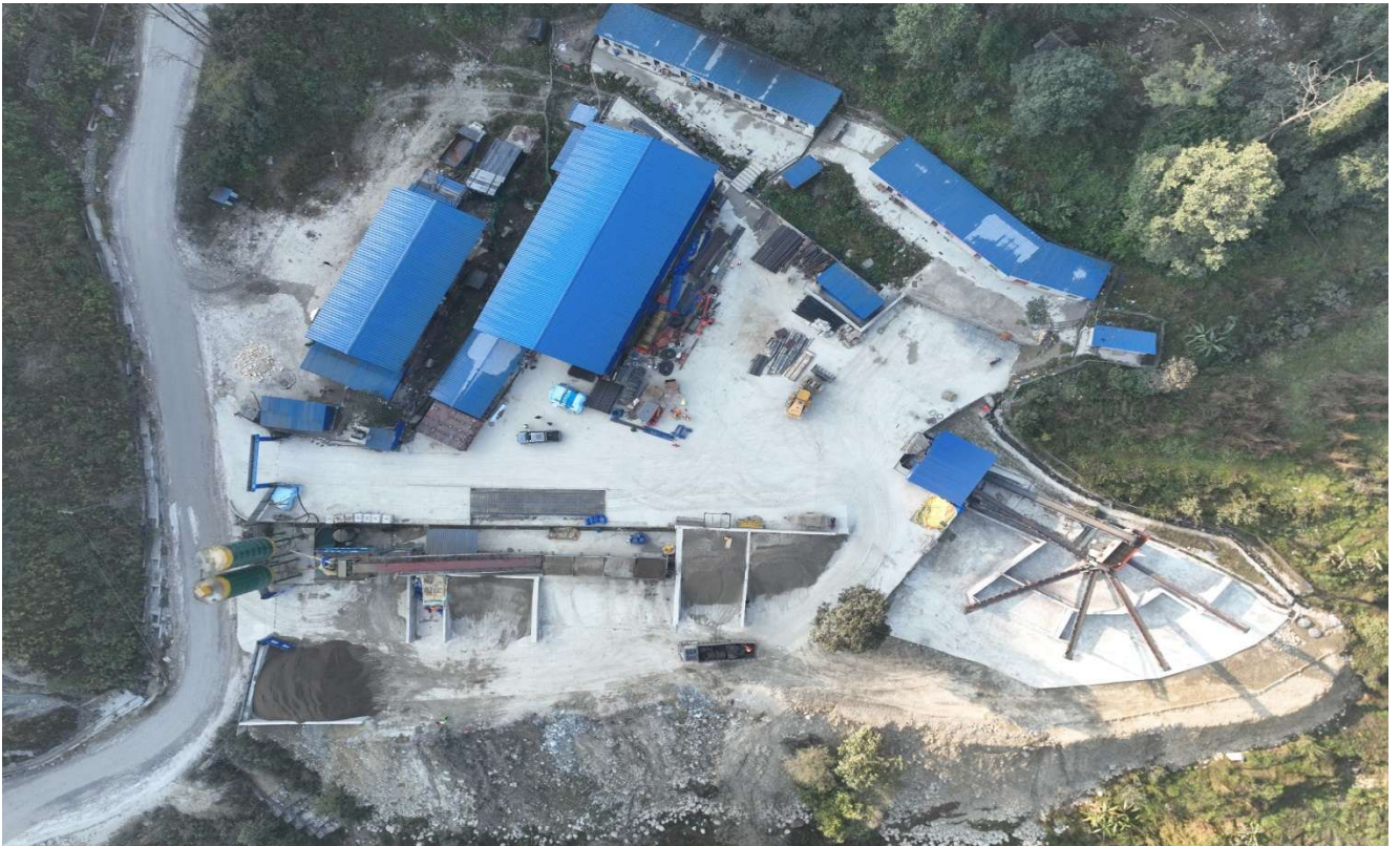
Fig: Workshop Area/ Crusher Plant /Batching Plant
