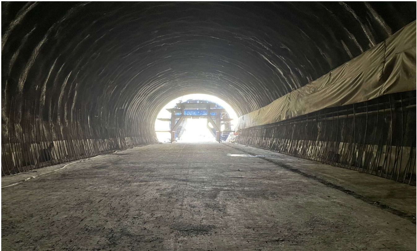
Fig: Main Tunnel after construction of Invert
