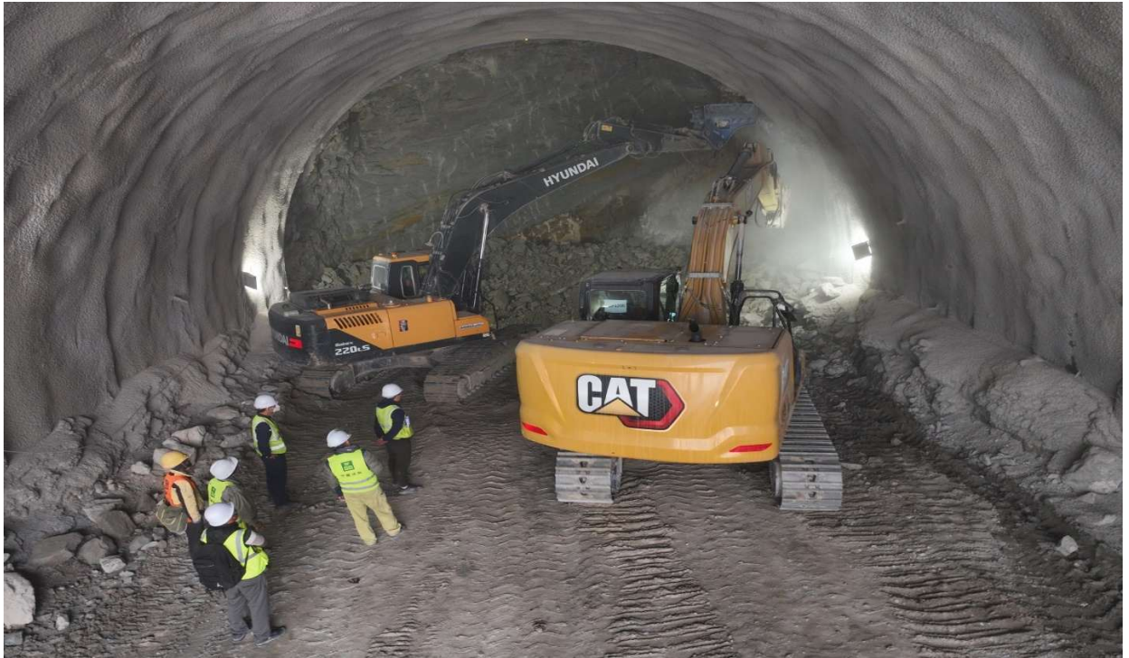
Fig: During Mechanical Excavation Works in Main Tunnel From South Portal Area
