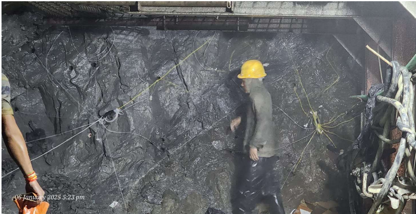
Fig: During preparation for Blasting Works
