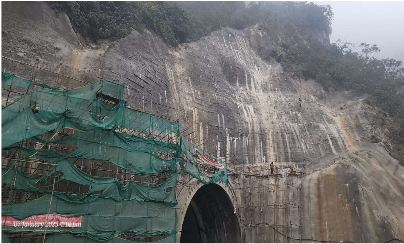
Fig: South Portal Area after slope stabilization
