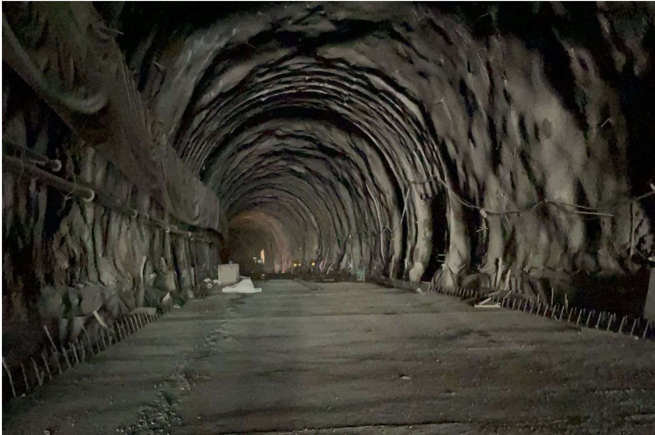
Fig: Main Tunnel after construction of Invert
