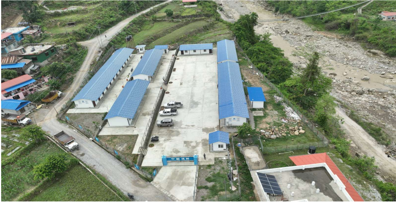
fig: Contractor's Site Camp and Lab
