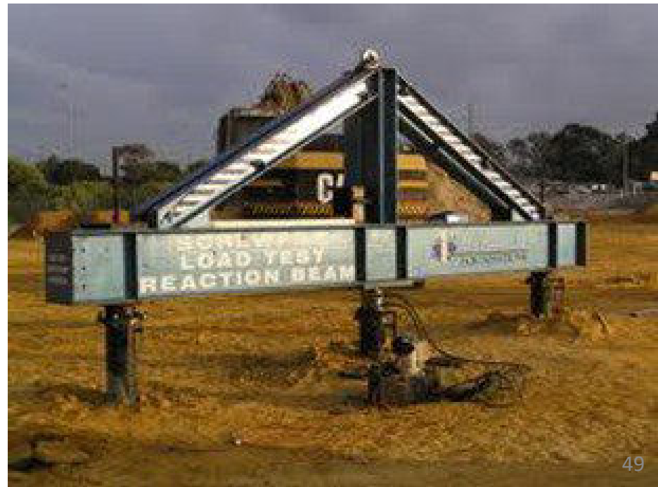
Fig: Vertical load test on piles
