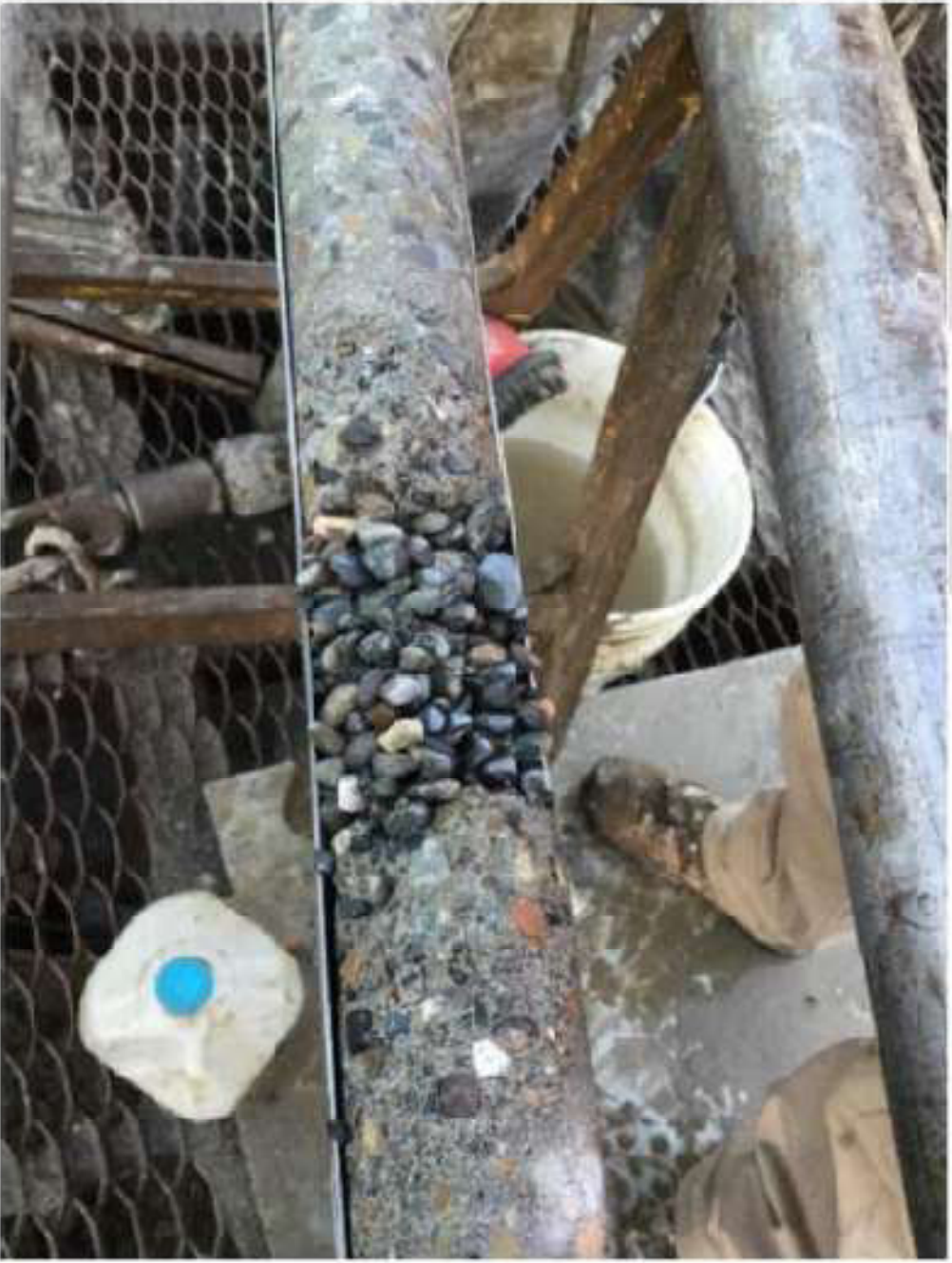
Coring results in a defective drilled shaft.
