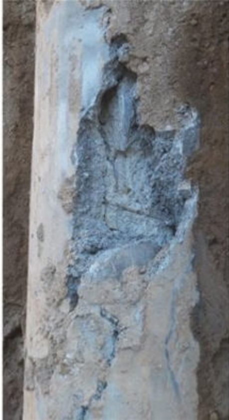
Cracked Pile
