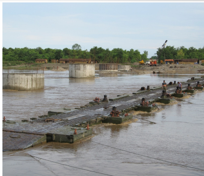
CONSTRUCTION OF WELL FOUNDATION 3, 4 , 5 AND 6
