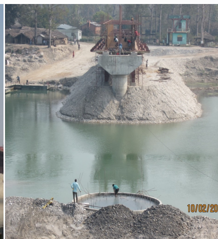
COMPLETION OF WELL SINKING
