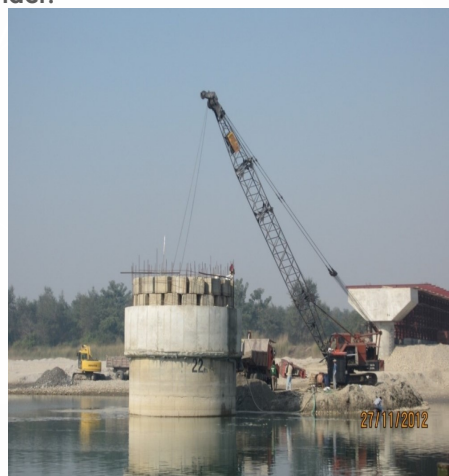
WELL BEFORE PUMPING IN
