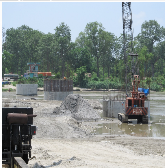
CONSTRUCTION OF WELL FOUNDATION 3, 4 , 5 AND 6
