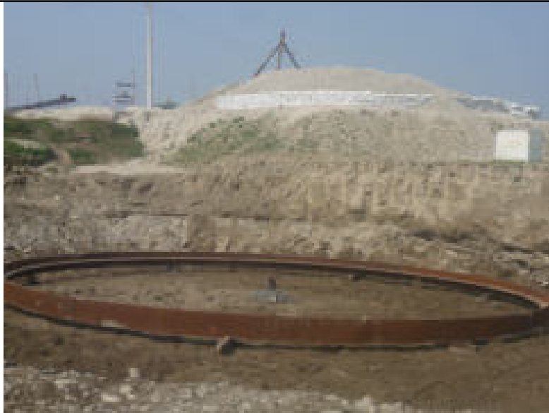
PLACING OF CUTTING EDGE
