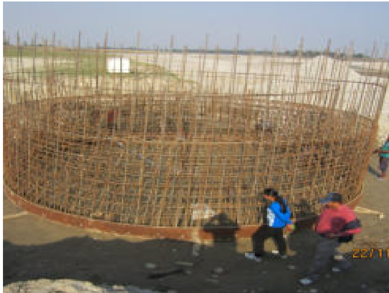
PLACING REINF. ON CUTTING EDGE
