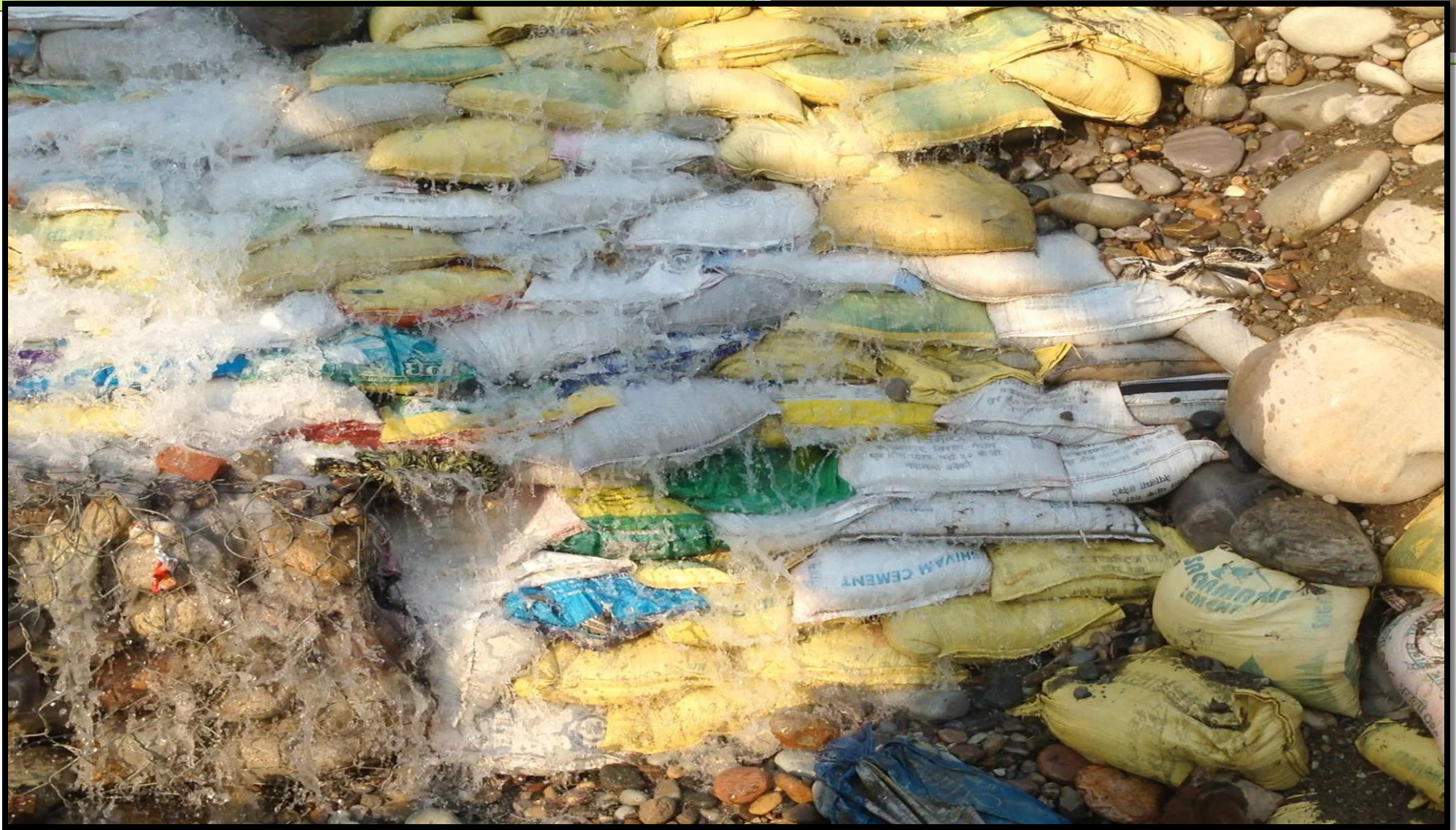
BHERI BRIDGE, RIMNA
