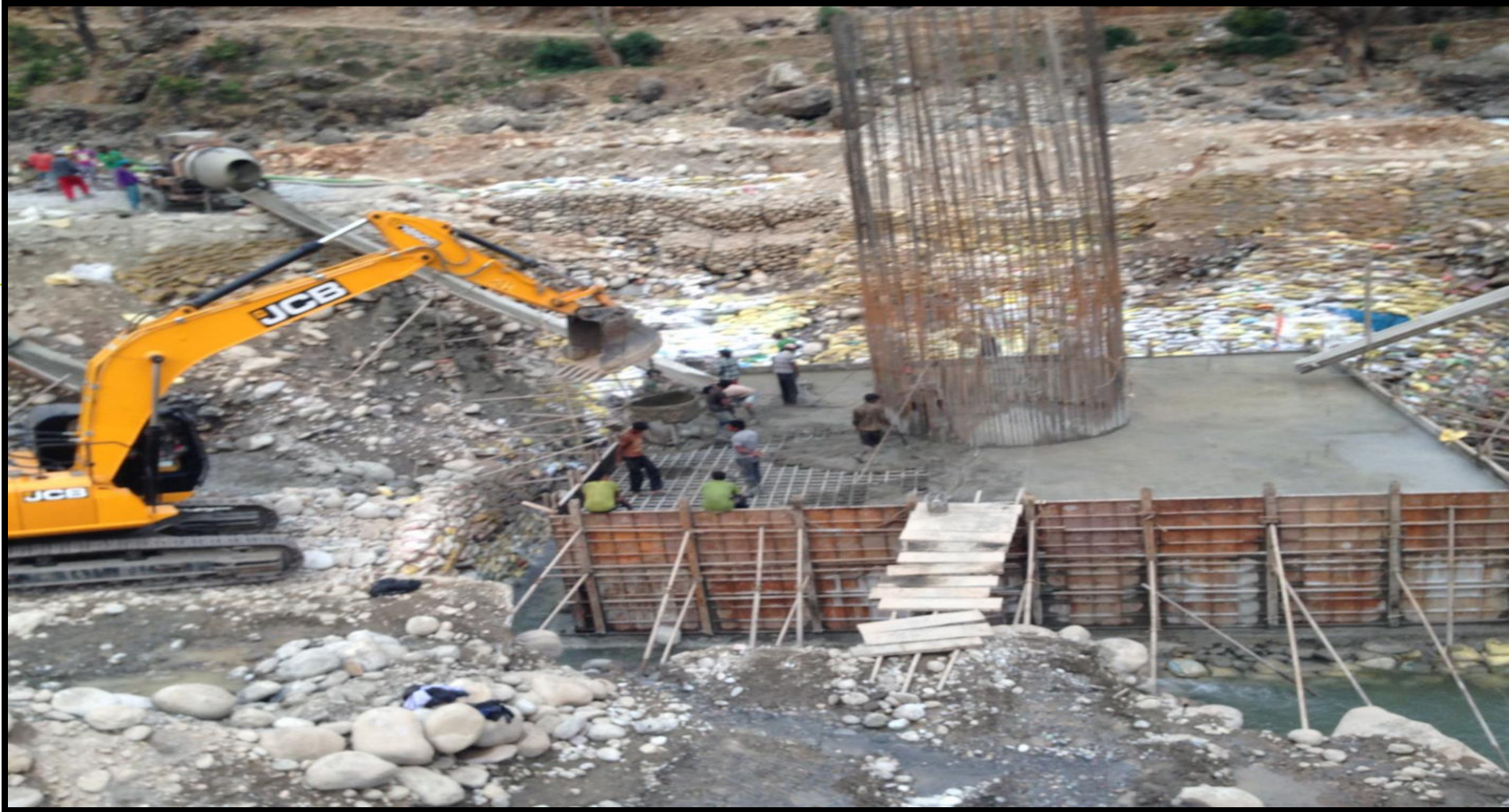
Concreting on Pier Footing
