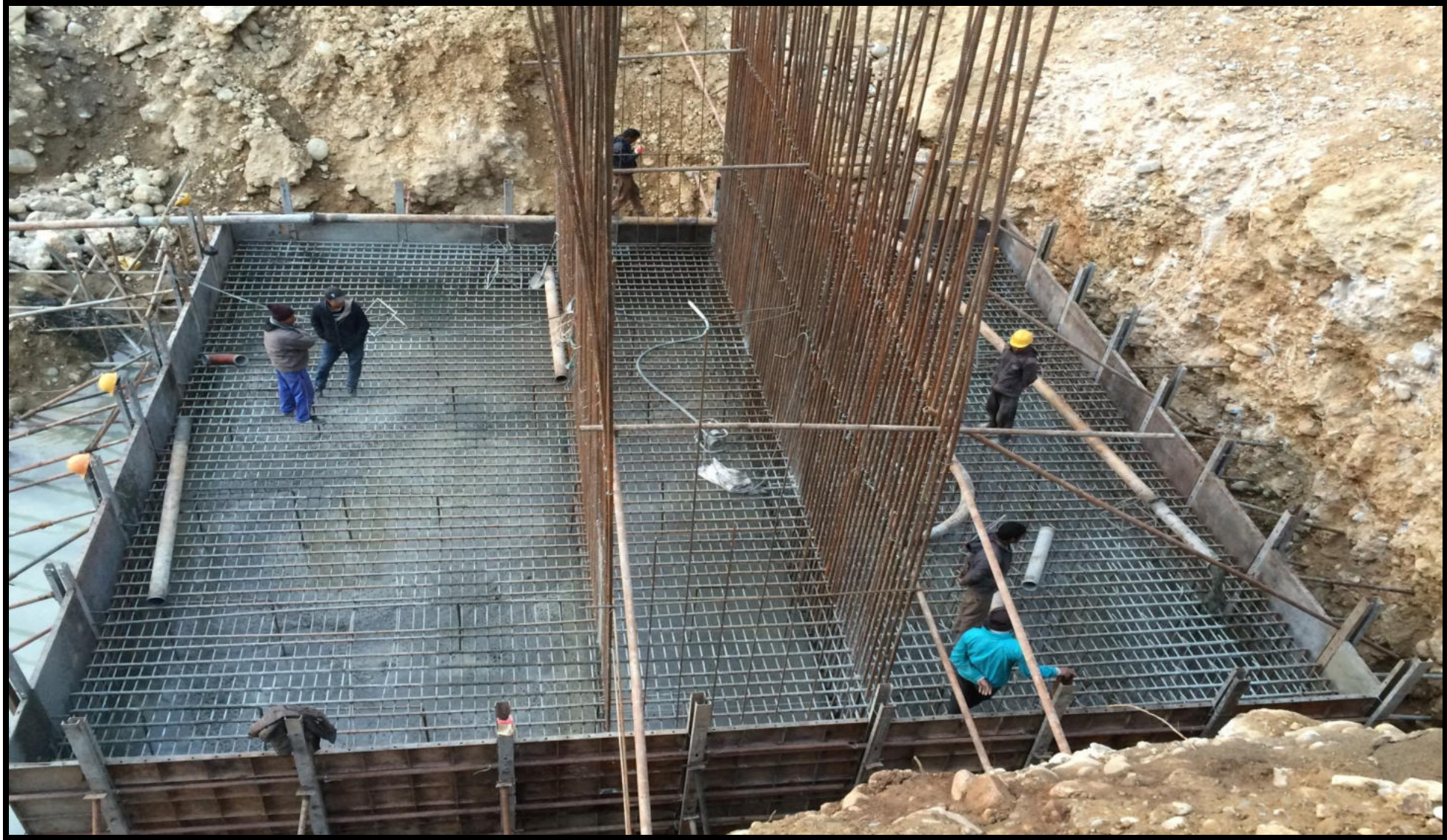
BHERI BRIDGE, RIMNA
