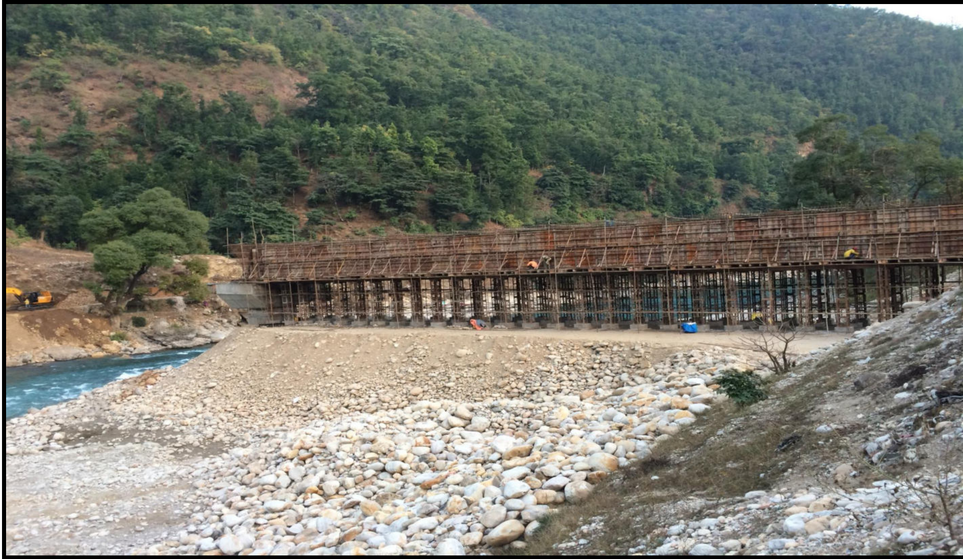
CONSTRUCTION OF RIGHT SPAN SUPERSTRUCTURE
