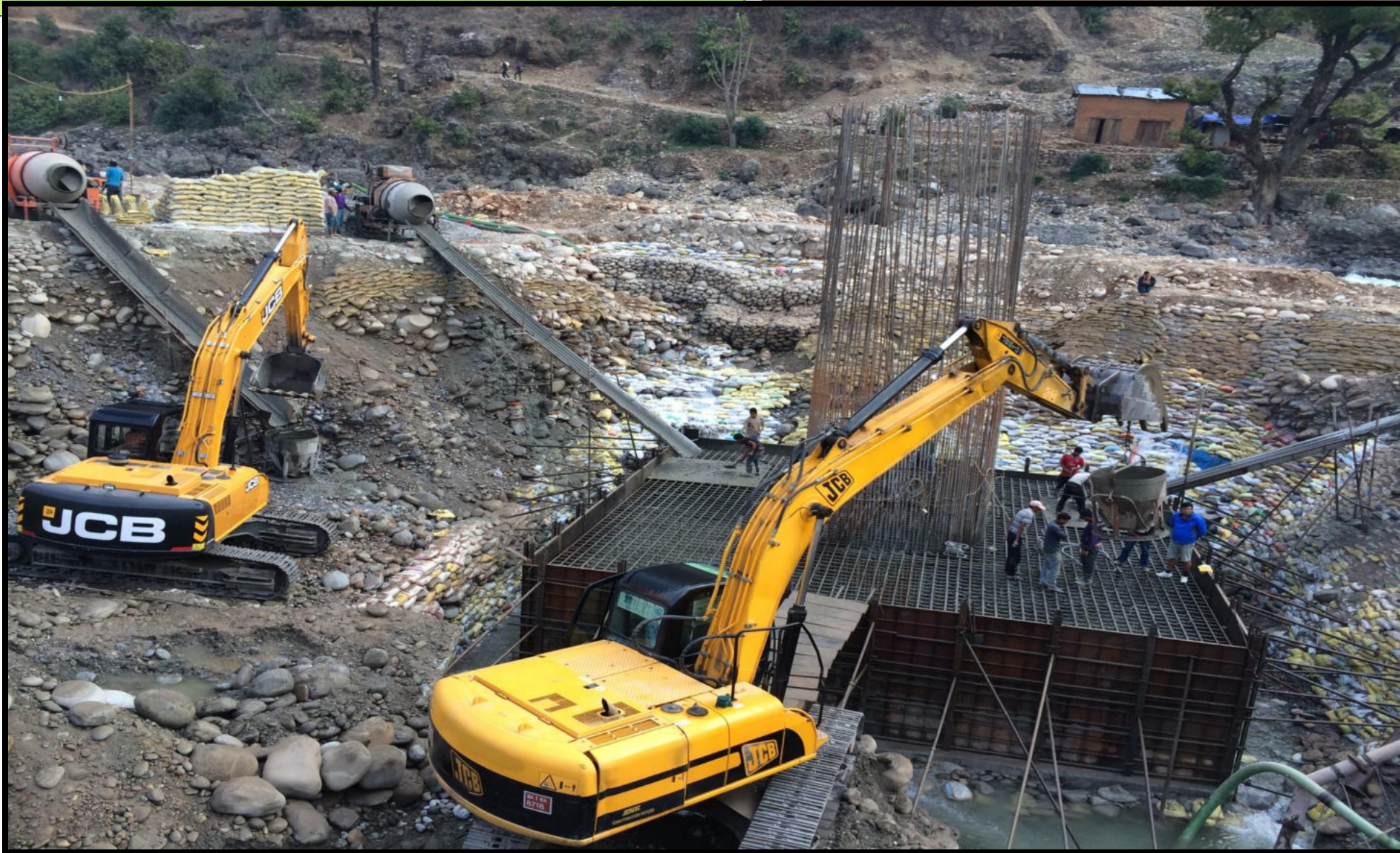
BHERI BRIDGE, RIMNA
