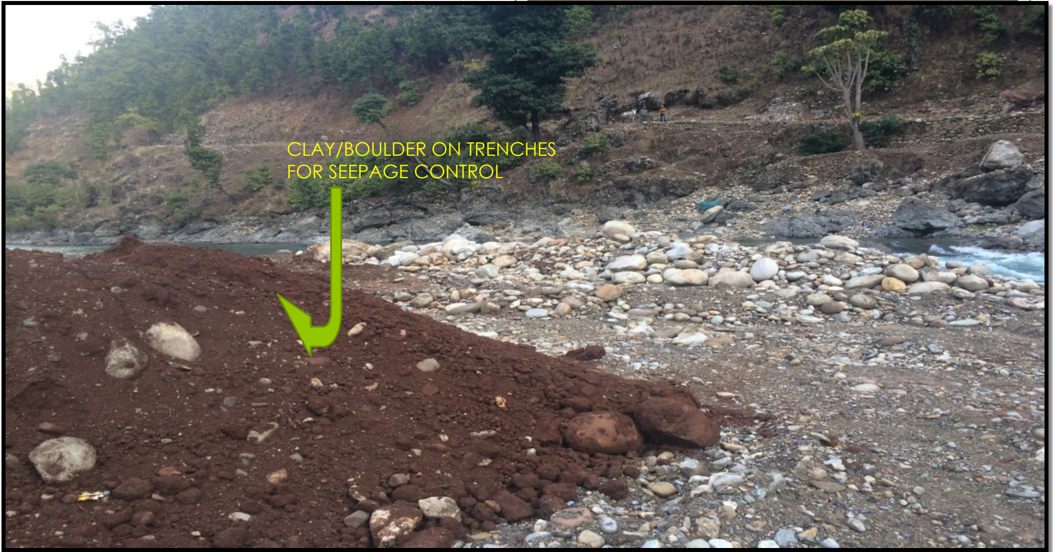
BHERI BRIDGE, RIMNA
