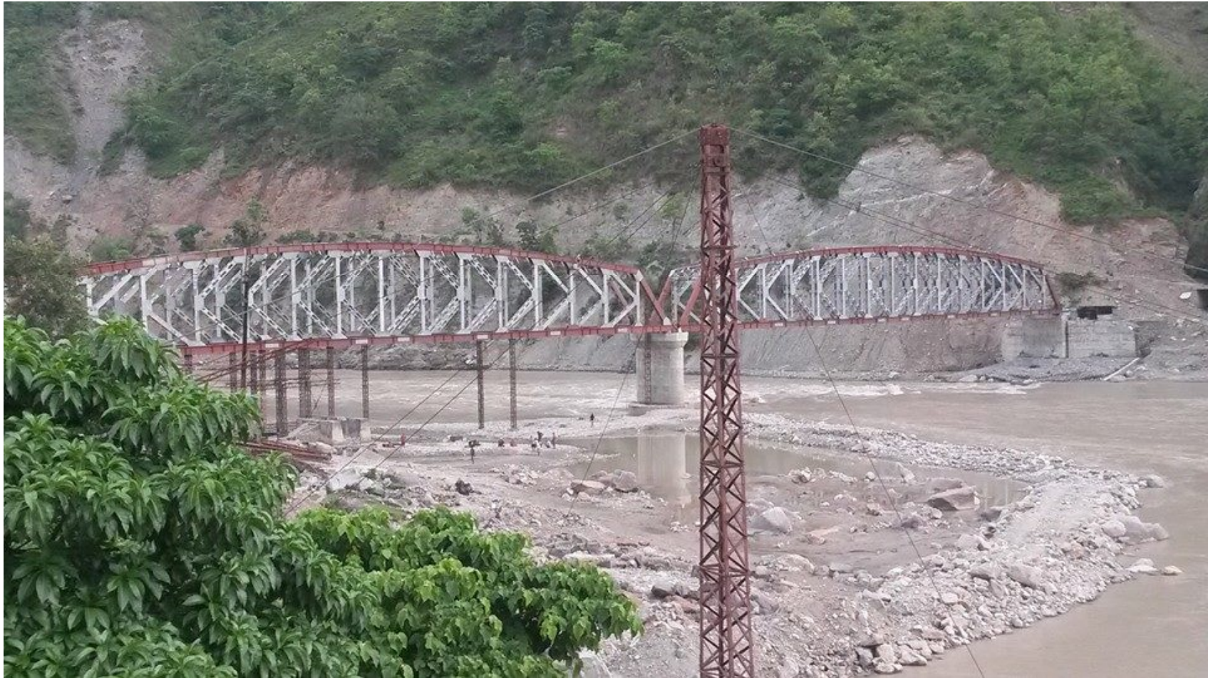
Bridge At Sunkoshi Bridge, Katari Okhaldhunga Road
