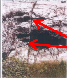
Plate 2: The excavated foundation pit of the right abutment in grey-green slate. Two prominent joints are seen to run NNE-SSW, almost parallel to the riverbank and extend beyond the anchorage block of the suspension bridge. View to NNE.
