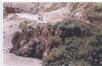
Plate 3: A close-up view of the right abutment. Note a rock cliff below the road with some overhangs and pool with eddies below the cliff. The water depth is more than 7 m. View to SW.
