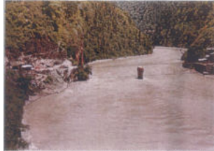
Plate 1: The Sunkoshi Bridge site north of Dolalghat. View to N. Note the steep river gorge and high currents.
