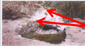
Plate 2: The excavated foundation pit of the right abutment in grey-green slate. Two prominent joints are seen to run NNE-SSW, almost parallel to the riverbank and extend beyond the anchorage block of the suspension bridge. View to NNE.
