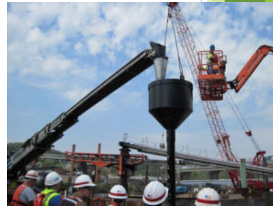
Method of underwater concreting— Tremie method (inside view)
