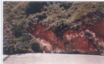
Plate 4: Scene of rock cliff upstream from the suspension bridge. Note some vertical joint faces with orange to brown colorations. A gabion wall (spur/dyke) is positioned at the grass spot below and upstream of the suspension bridge abutment to prevent scouring downstream. View to SW.
