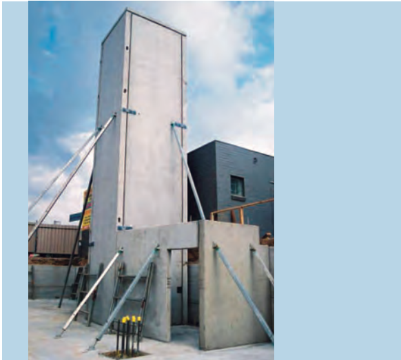
Precast wall panels The erection of precast concrete core walls for a lift shaft and stair core. Note the bracing of the panels with a minimum of two braces per panel and the precast panels would sit over projecting starter bars which fit into grout ducts in the precast walls, and which are later grouted.
