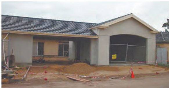
Precast walls for a garage and house extension
