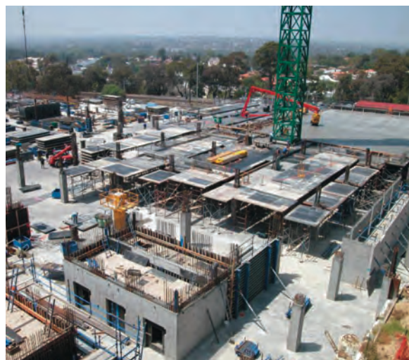
Insitu and precast concrete walls
