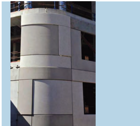
Precast cladding wall panels
