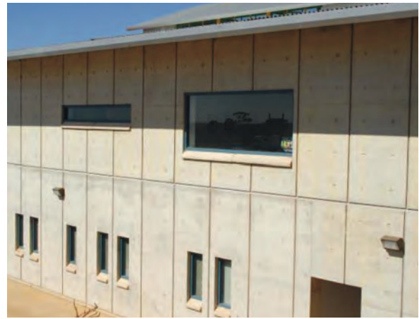
Insitu off form concrete walls Note the attention to the joint layout, construction joint locations (which will occur at the expressed joints) and the locations of the bolt holes or the form ties in this insitu wall to form a uniform pattern.
