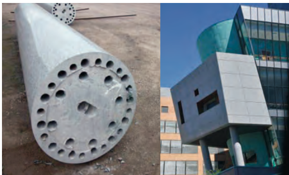
Polished round reinforced and post tensioned precast columns. These are unusual non-vertical columns, but illustrate how complex columns can be.
