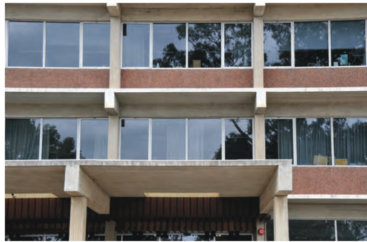
Figure 5.1 Long-term deflection of unsupported edge of insitu concrete slab
