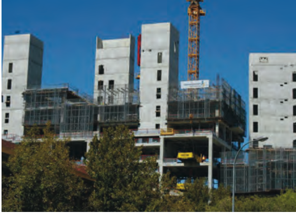
Insitu and precast concrete walls A series of insitu concrete core walls including both stair and lift shafts, constructed using climbing formwork before the floors below are cast.
