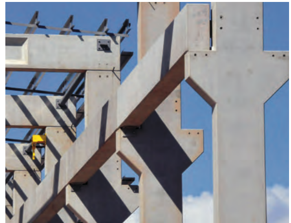
Figure 9.11 Double corbels on precast concrete columns
