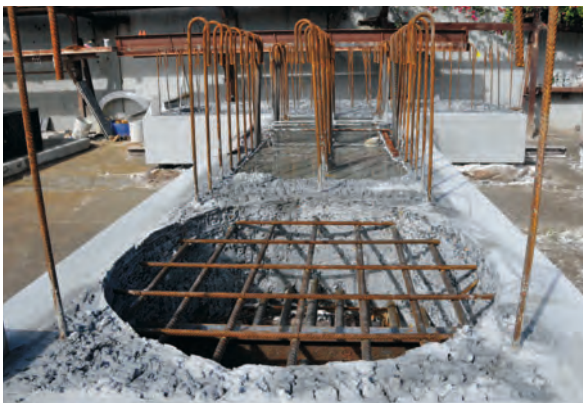
Figure 4.4 Precast pile cap with roughened surface
