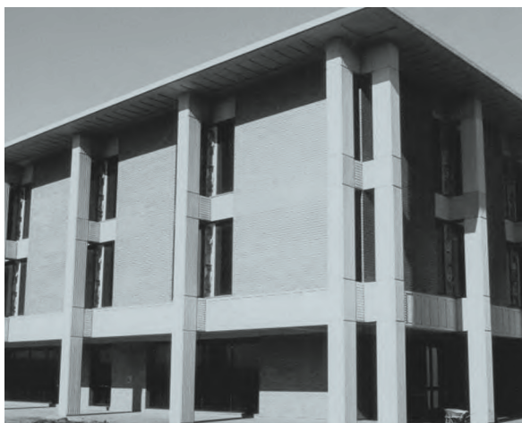
Figure 6.9 Columns requiring lateral shear reinforcement
