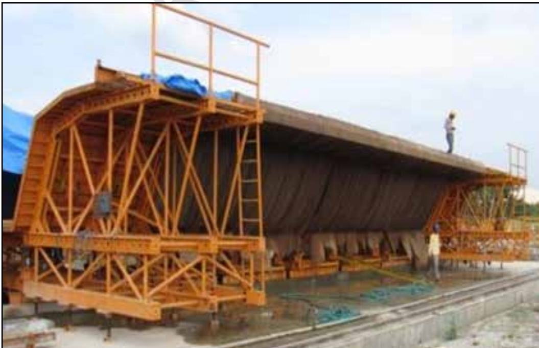
Figure-6.14: Typical Long-Line Production [1]
