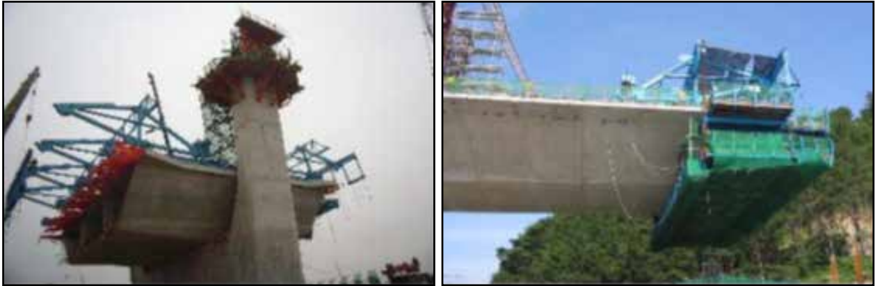
Figure-6.8: Erection of cast-in-place segments on scaffolding (Ah-am Bridge in S. Korea) [6]
