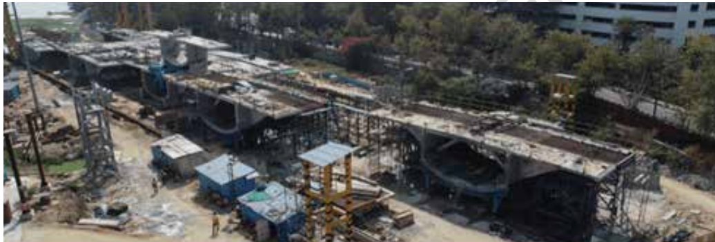
Figure-6.44: Casting yard for precast segments [9]
