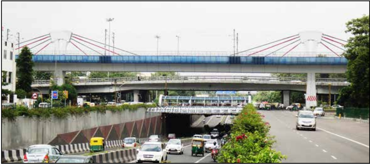
Fig 5.12 Extradosed Bridge at Moolchand, Delhi Note shape of Piers and multi-coloured stays
