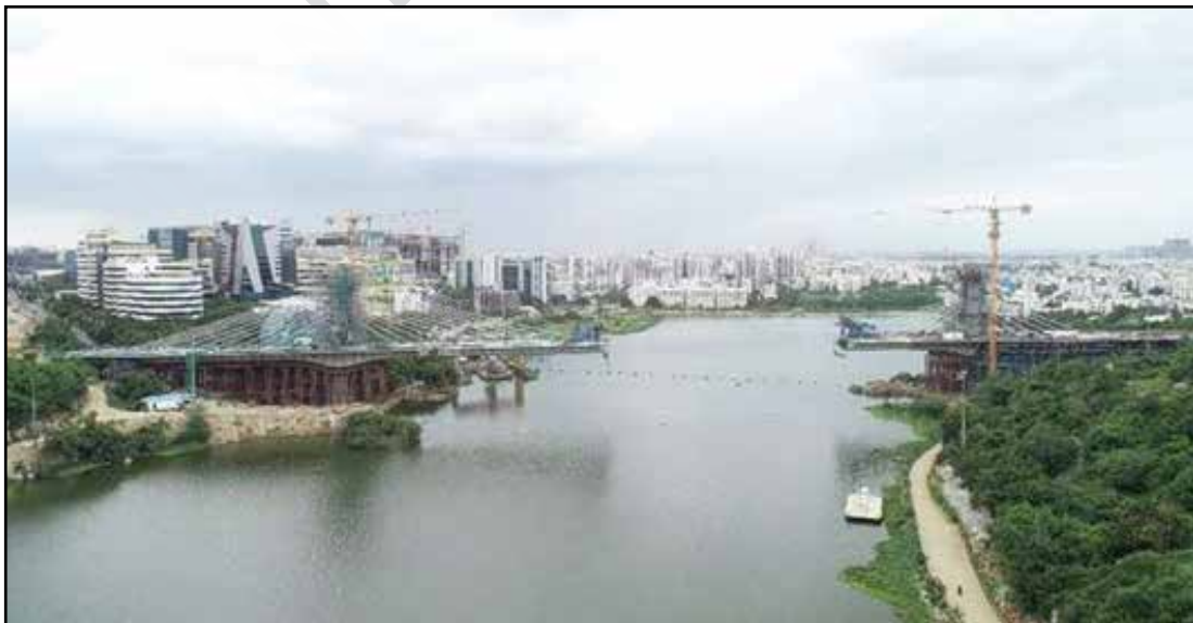
Figure-6.12: Construction of balanced cantilever construction for
