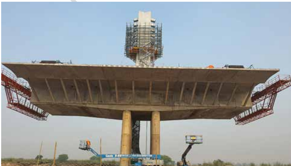
Fig 5.2 Reducing Pier Stiffness
