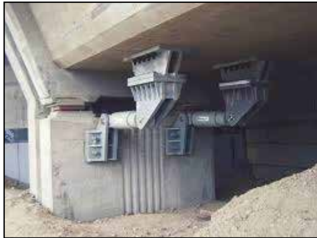
Fig 9.19 Shock Transmission Unit
