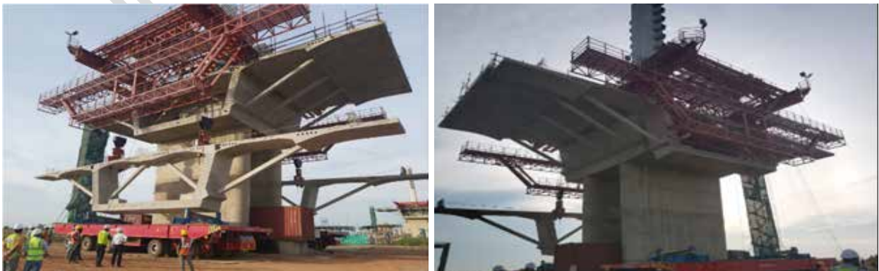
Figure-6.56: Erection of main span by free cantilever method [9]
