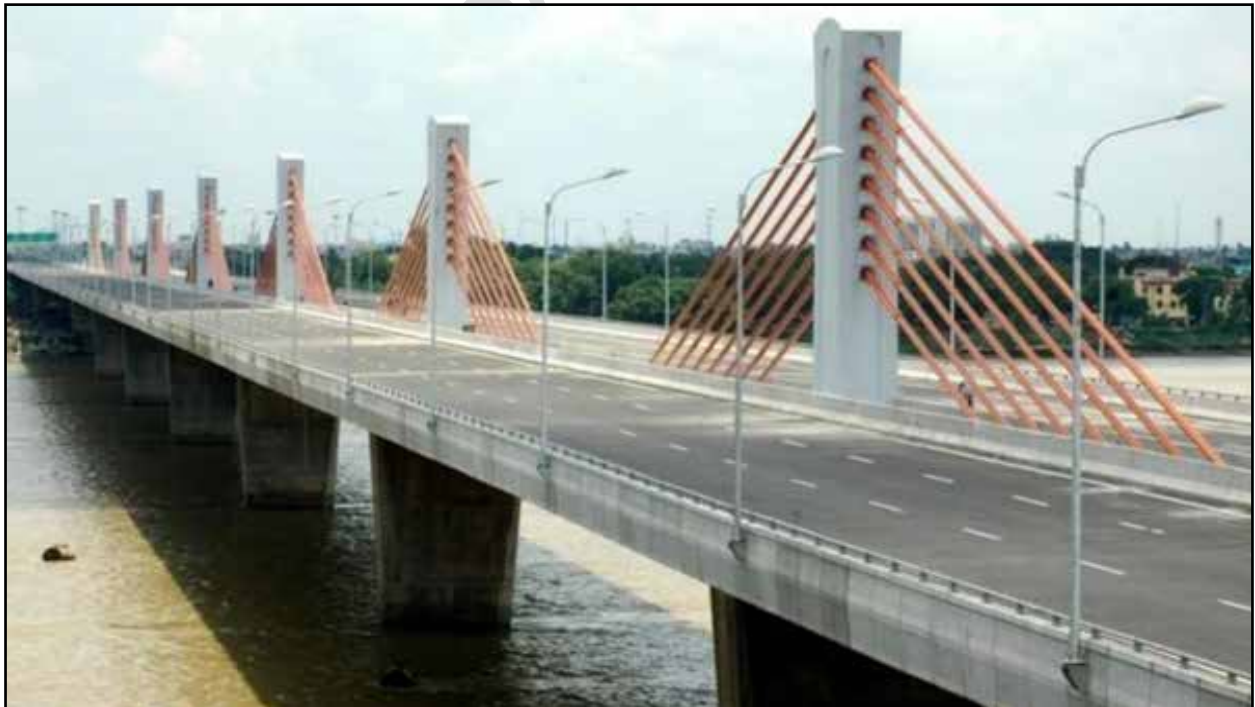
Figure-6.1: Second Vivekananda Bridge public over Hooghly River [9]
