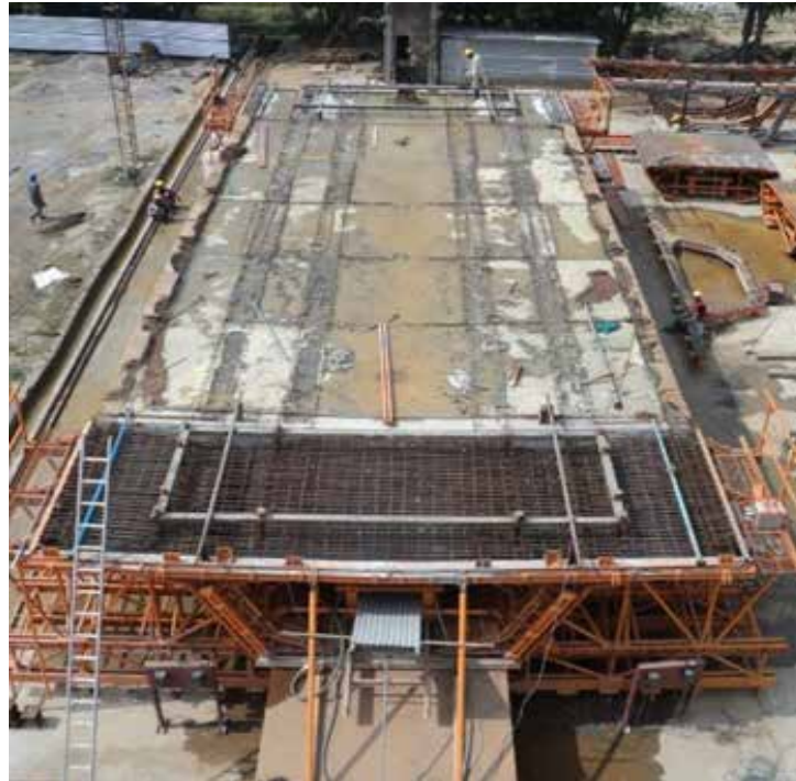
Figure-6.16: Long-Line method [9]
