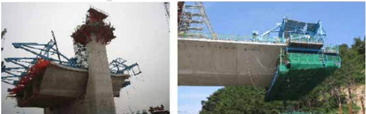
Figure-6.23: Form traveler erection arrangement [6]
