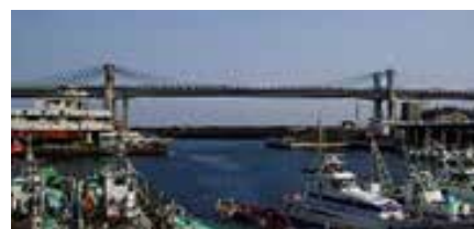
Fig. 2.2 :Odawara Blueway Bridge (Japan)
