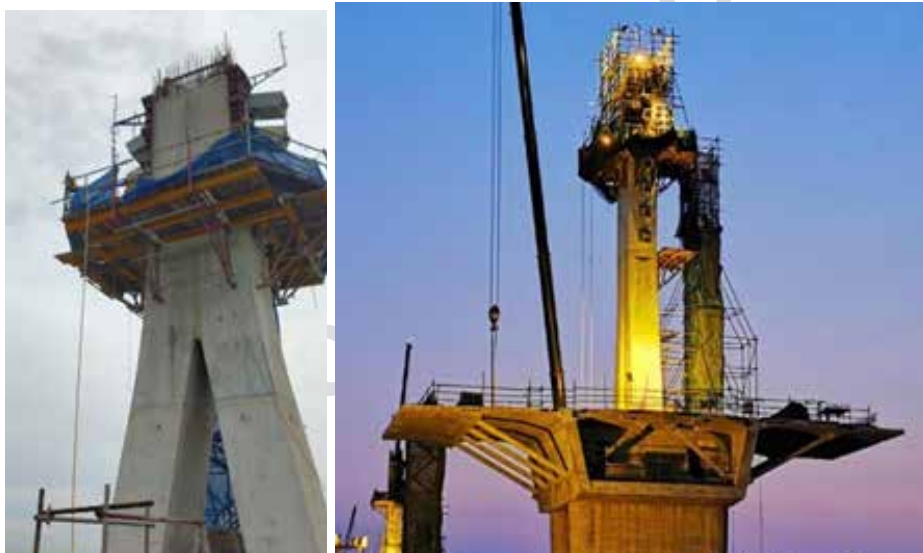
Figure-6.55: Upper Pylon Construction [9]
