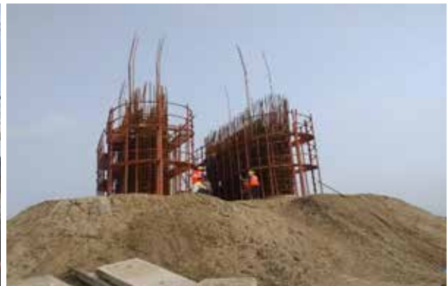
(ii) Lower pylon construction in Land mode
