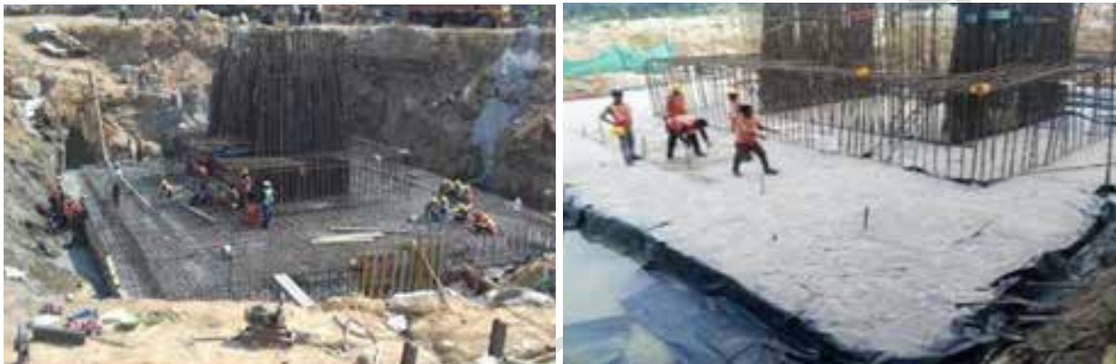
Figure-6.39: Construction of Foundation [9]
