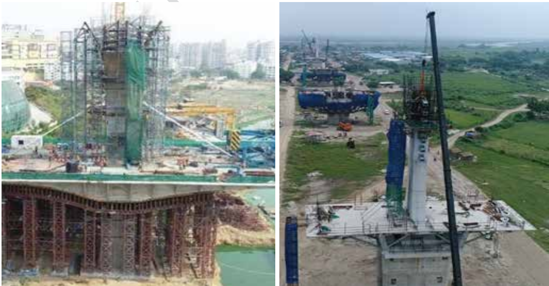
(i) Full Trestle Support (ii) Jump Formwork
