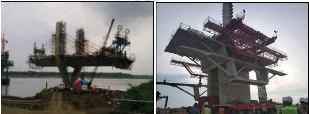
Figure-6.9: Balance Cantilever Erection of Precast Segment [9]
