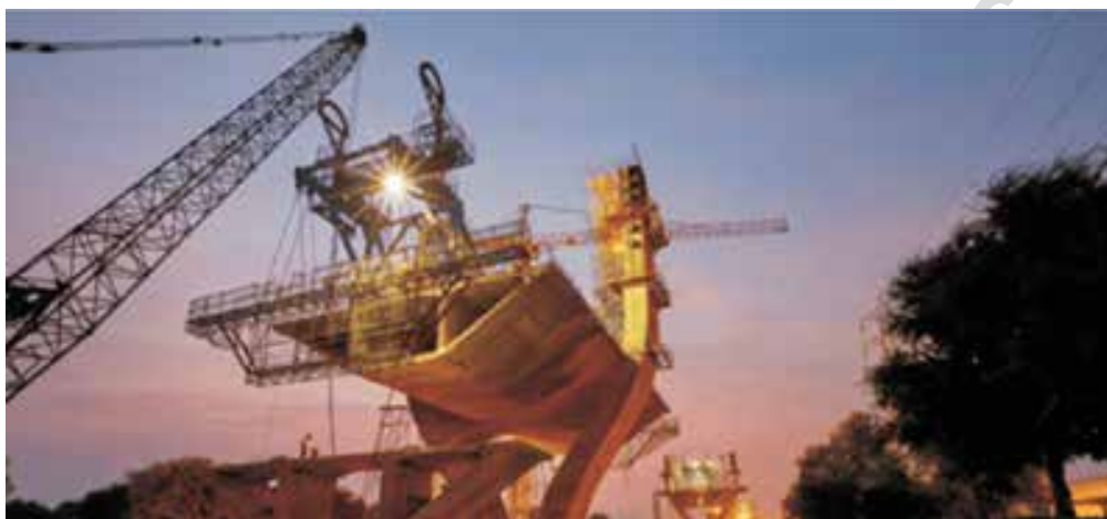
Figure-6.32: Bridge Builder arrangement on Pylon-span [9]
