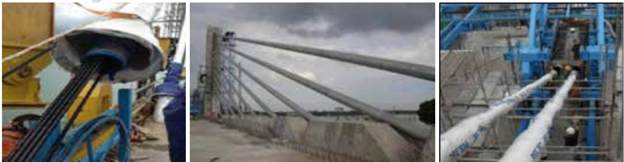
Figure-6.20: Cable Stay System [10]
