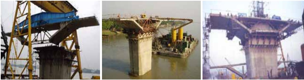
(i) Shifting Pier Table Segment (ii) Erected Pier table segments (iii) Finished Pier Table
