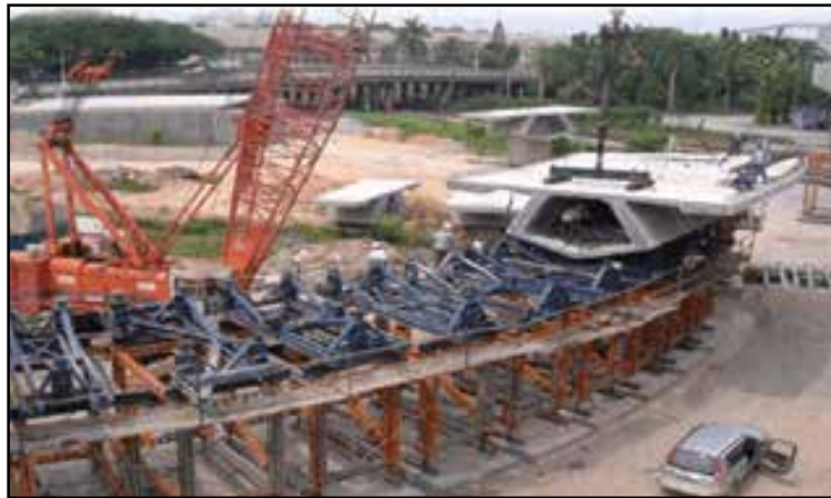
Figure-6.7: Erection of precast segments on scaffolding [5]
