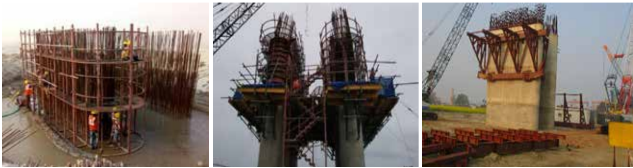
(i) Rebar assembly (ii) Installation of Form work
