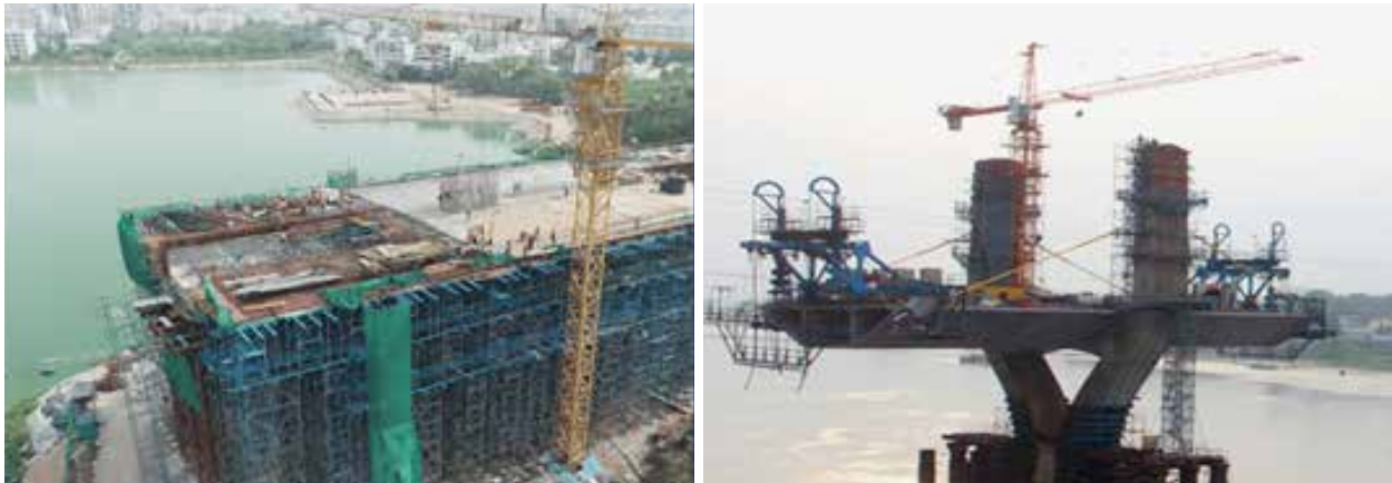
Figure-6.5: Tower Crane for Pylon Construction [9]
