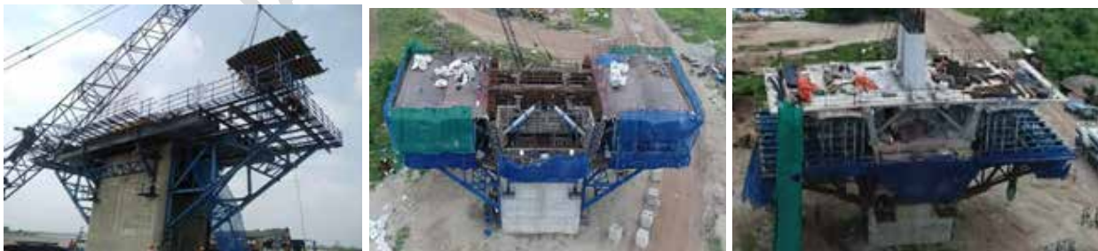
(i) Bracket Erection (ii) Installation of Form work (iii) Finished Pier Table
