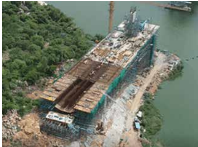
Figure-6.43: Construction of Deck back span [9]
