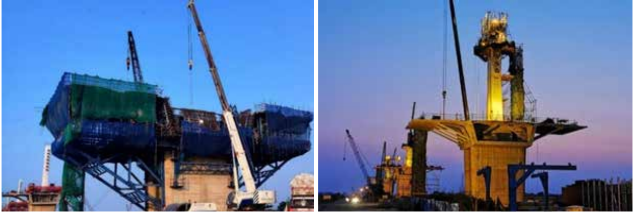
(i) Pier Table Shuttering (ii) Pier table concrete section
