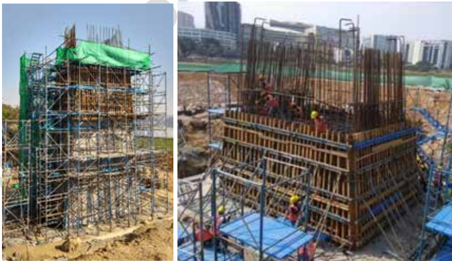
Figure-6.40: Construction of Lower pylon [9]
