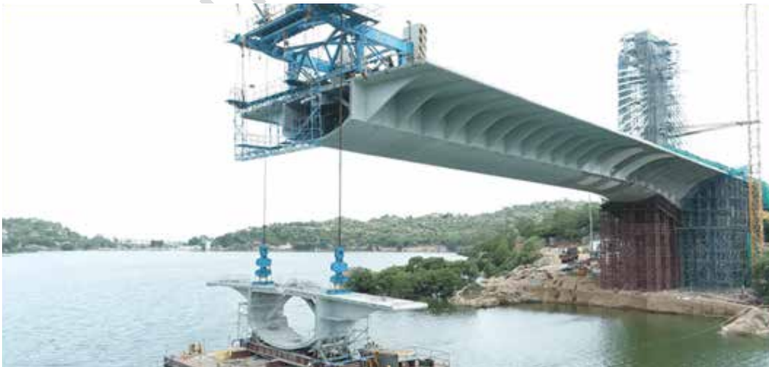
Figure-6.45: Erection of main span by free cantilever method [9]
