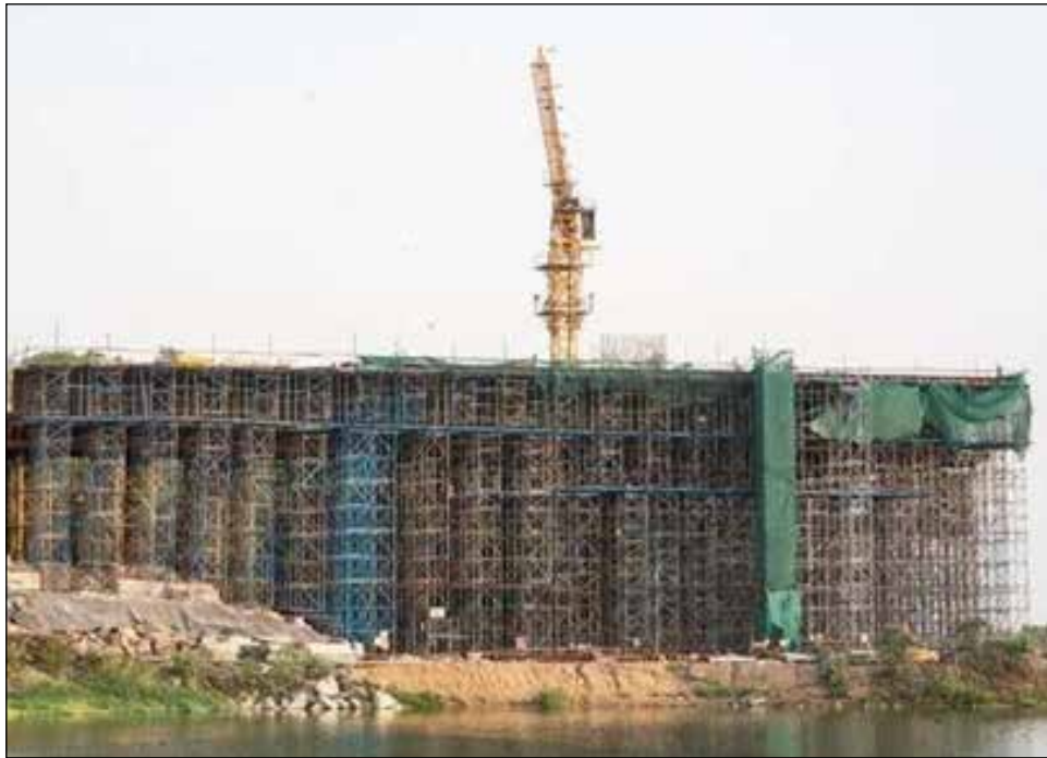
Figure-6.41: Construction of Pier table [9]
