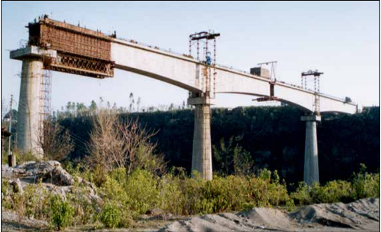
Fig 5.6. Completing Unbalanced Portion of End Span of Free Cantilevering in Jammu Udhampur Rail Link with Span Arrangement of 70+102+70=242\text{m} . Height at Piers= 70M
