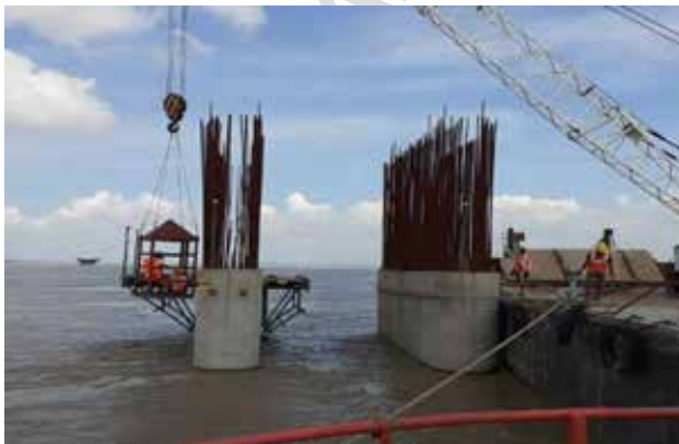
(i) Lower pylon construction in Water mode
