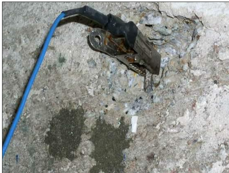
Figure 10.2: Connecting reinforcing steel with crocodile clip
