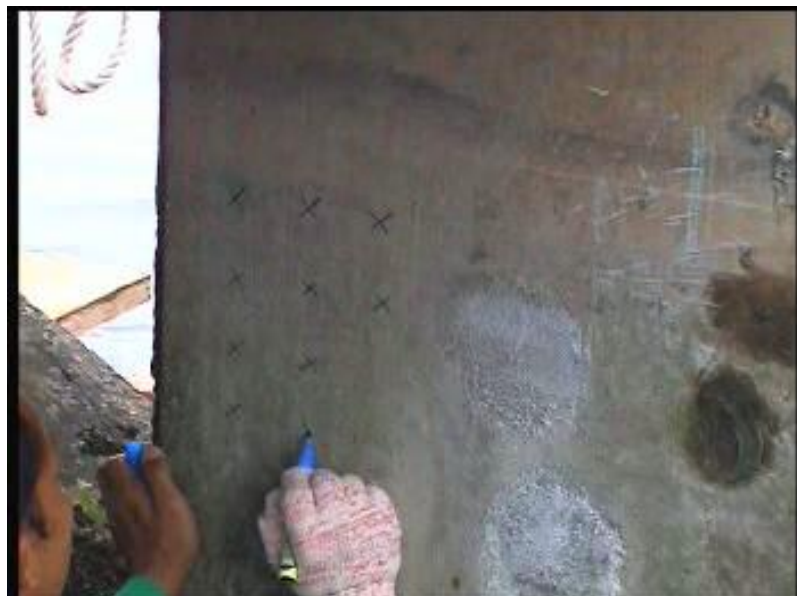
Figure 6.3: Marking test points according to grid
