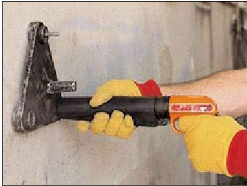
Figure 8.2: Positioning the driving unit with probe before fire into the concrete
