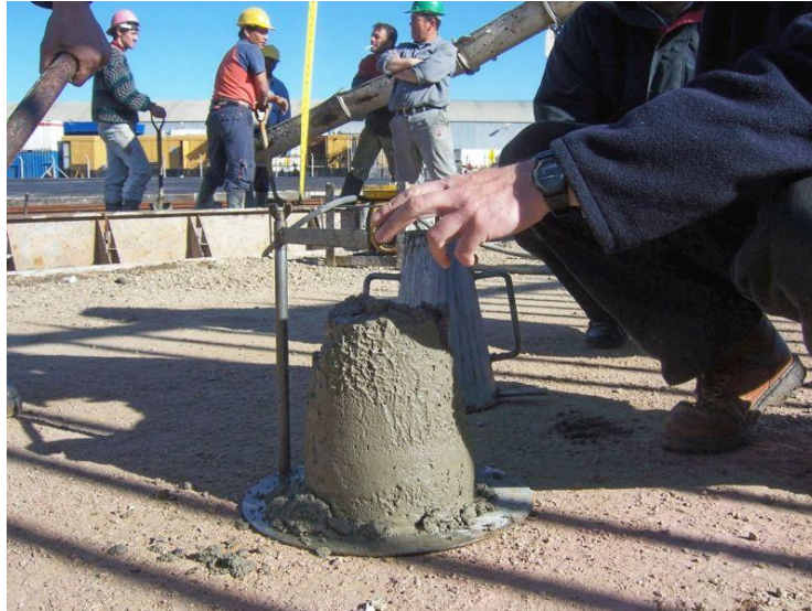
Figure 2.5 : Measured to determine slumps
