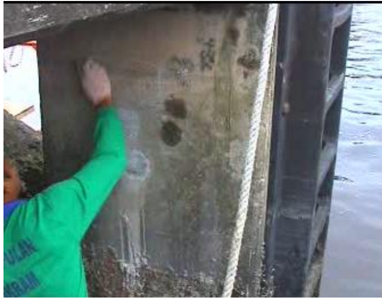
Figure 6.2: Brushing concrete surface to remove roughness and loose materials before test
