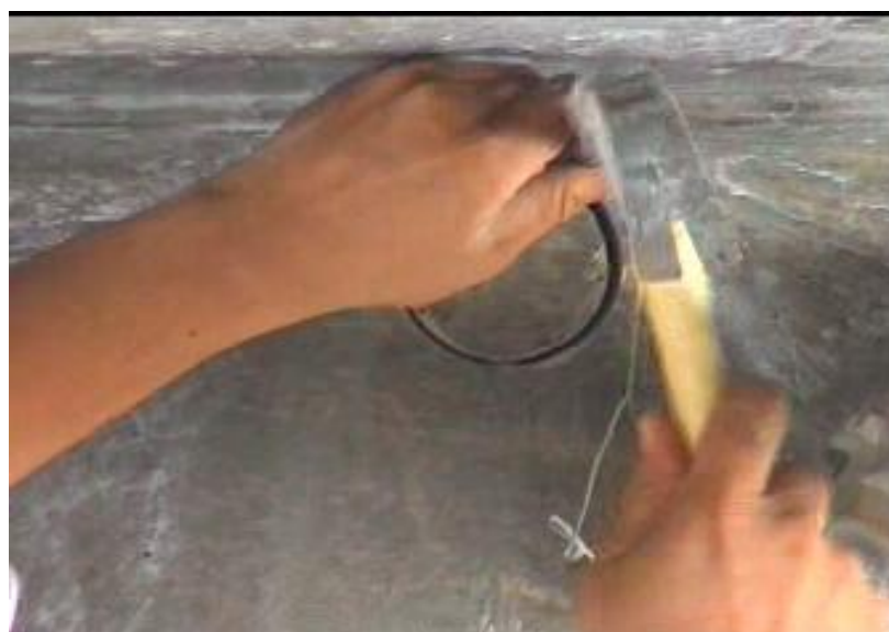
Figure 5.4: Extracting core from the structure
