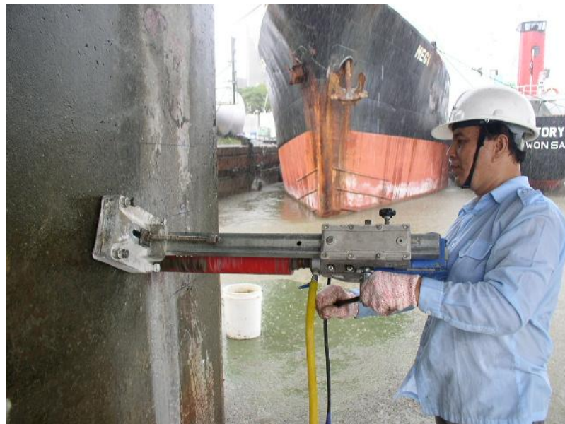
Figure 5.3: Coring process
