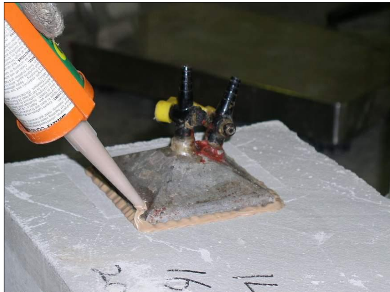
Figure 11.2: Fixing the cap onto concrete surface
