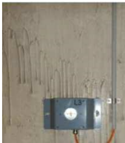
Picture 3: Example of fire emergency lighting
