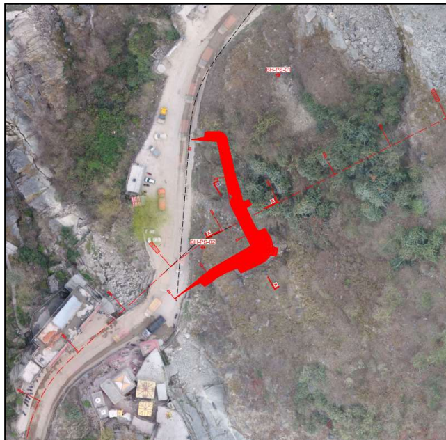
Figure 34 - South Portal Area
