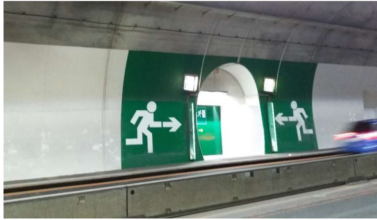
Figure 6: Example of emergency escape route with sliding fire resistant door and proper marking
