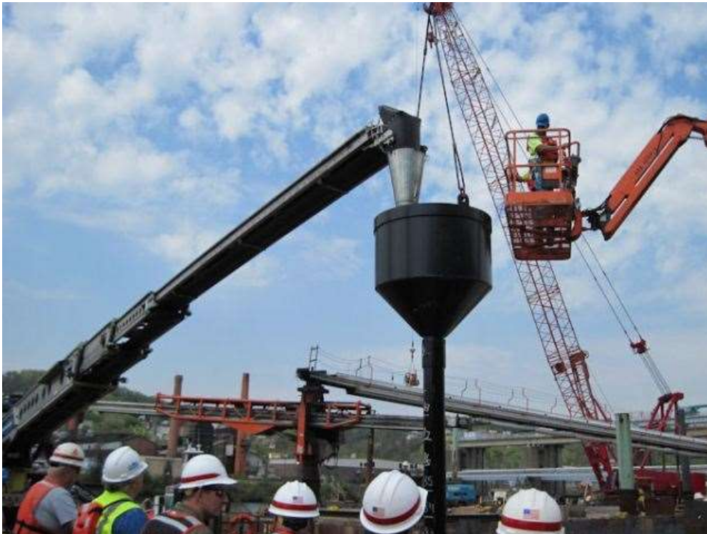
Figure 3.1 Tremie Concreting Method
