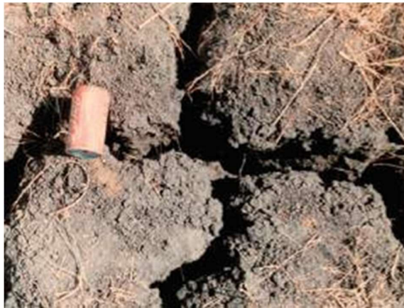
Figure D-2: Expansive soil exhibiting wide shrinkage cracks [11]
