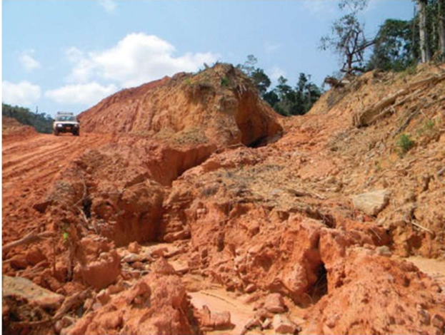
Figure D-10 Example of severe erosion in erodible/dispersive soils [11]
