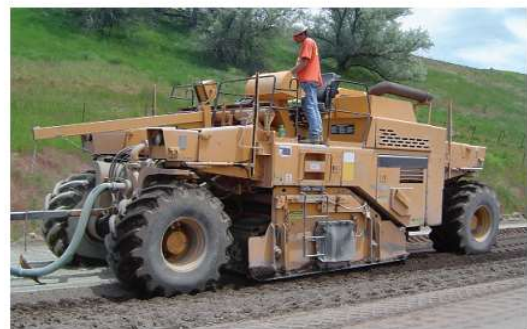
Mixing CTB in place using a single-shaft traveling mixer.
