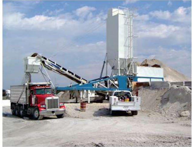
Mixing CTB in a continuous-flow-type pugmill.
