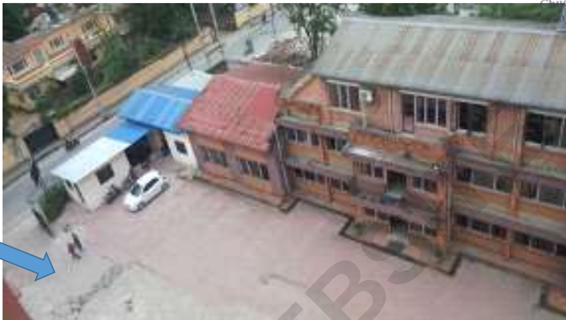
Photo 1: Entry point of proposed building
