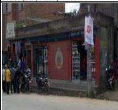
Structure No. 23: Sanu Shrestha, Mahadevsthan 1 Kha, Plot No. 336, Brick Masonry with RCC Roof, Full Impact, 0+200, Left Side
