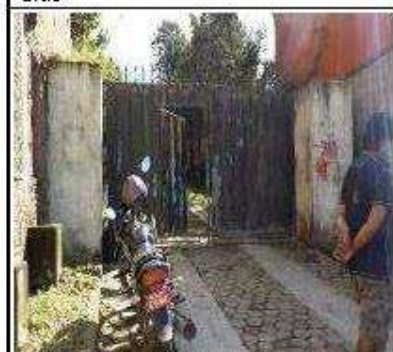
Structure No. 43: Sakunta Lal Hirachan, Mahadevsthan 1 Kha, Plot No. 288, Metallic Gate with Brick Masonry, Full Impact, 0+405, Left Side
