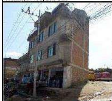
Structure No. 46: Rajib Maharjan, Mahadevsthan 1 Kha, Plot No. 371, RCC Frame Structure, Full Impact, 0+430, Left Side
