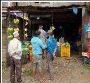
Structure No. 32: Nil Bahadur Maharjan, Mahadevsthan 1 Kha, Plot No. 364, CGI Sheet Structure, Full Impact, 0+248, Left Side
