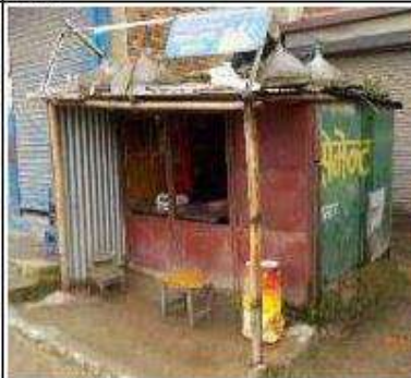
Structure No. 29: Gyani Maharjan, Mahadevsthan 1 Kha, Plot No. 261, 263, 342, CGI Sheet Structure, Full Impact, 0+240, Left Side
