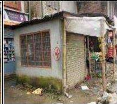
Structure No. 30: Gyani Maharjan, Mahadevsthan 1 Kha, Plot No. 261, 263, 342, Brick Masonry and CGI Sheet Roof, Full Impact, 0+245, Left Side
