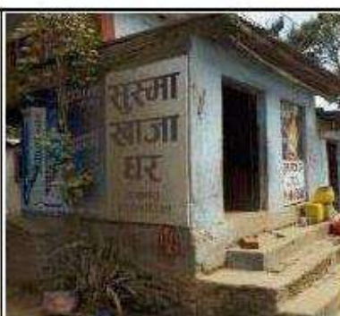
Structure No. 14: Kulchandra Silwal, Balambu 6 Kha, Plot No. 361, Brick Masonry with RCC Roof, Full Impact, 0+100, Right Side
