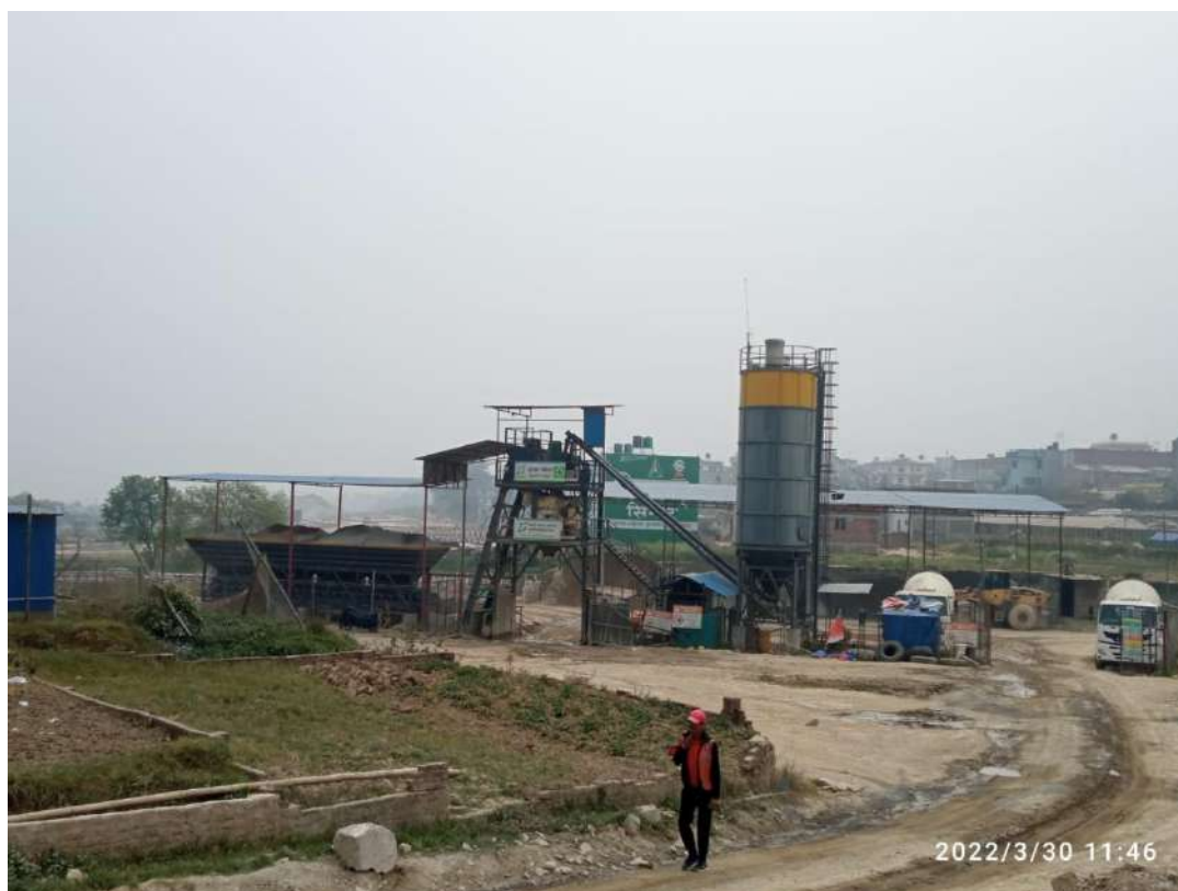
Figure 7-1: Batching Plant Site
