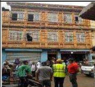
Structure No. 35: Kaji Maharjan, Mahadevsthan 1 Kha, Plot No. 365, RCC Frame Structure, Partial Impact, 0+255, Left Side
