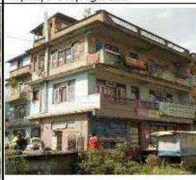
Structure No. 21: Hera Krishna Maharjan, Mahadevsthan 1 Kha, Plot No. 310, RCC Frame Structure, Partial Impact, 0+180, Left Side
