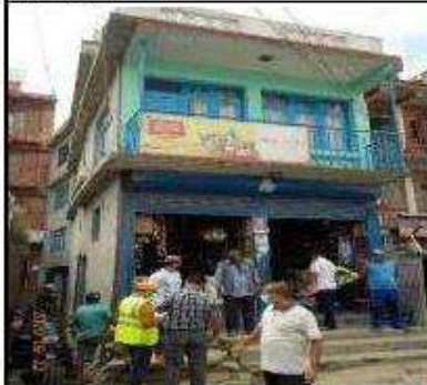
Structure No. 28: Aasha Lal Shrestha, Mahadevsthan 1 Kha, Plot No. 343, RCC Frame Structure, Partial Impact, 0+235, Left Side
