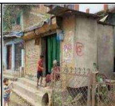
Structure No. 15: Prem Nath Silwal, Balambu 6 Kha, Plot No. 362, Brick Masonry with CGI Sheet Roof, Full Impact, 0+090, Right Side
