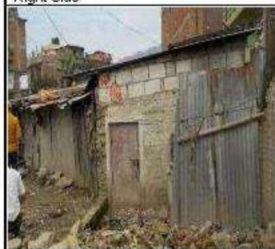
Structure No. 16: Jiwan Kumar Thapa, Balambu 6 Kha, Plot No. 190, Concrete Block with CGI Sheet Roof, Partial Impact, 0+055, Right Side
