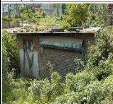
Structure No. 20: Hera Krishna Maharjan, Mahadevsthan 1 Kha, Plot No. 310, Brick Masonry with CGI Sheet Roof, Full Impact, 0+175, Left Side
