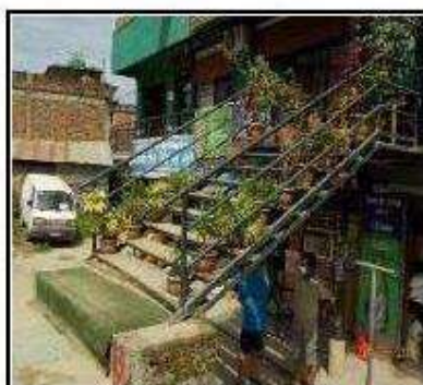
Structure No. 13: Puneshwari Nakami, Mahadevsthan 1 Ka, Plot No. 444, Steel Stair and Oil Tank, Full Impact, 0+170, Right Side
