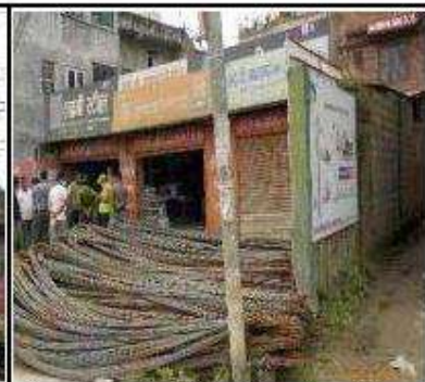
Structure No. 27: Nhuchhe Maya Shrestha, Mahadevsthan 1 Kha, Plot No. 345, 346, Concrete Block with CGI Sheet Roof, Partial Impact, 0+225, Left Side
