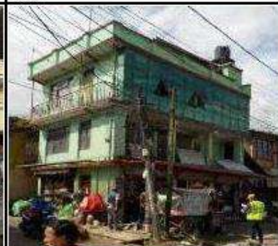
Structure No. 36: Mohan Devi Khadgi, Mahadevsthan 1 Kha, Plot No. 19, RCC Frame Structure, Full Impact, 0+270, Left Side
