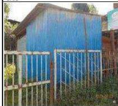
Structure No. 40: Sabina Shrestha, Mahadevsthan 1 Kha, Plot No. 355, CGI Sheet Structure, Full Impact, 0+375, Left Side
