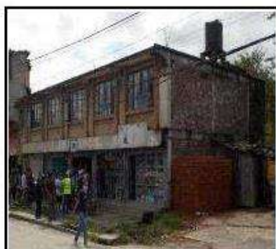
Structure No. 37: Kul Bahadur Maharjan, Mahadevsthan 1 Kha, Plot No. 281, RCC Frame Structure, Full Impact, 0+290, Left Side
