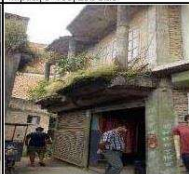
Structure No. 24: Kandhi Shrestha, Mahadevsthan 1 Kha, Plot No. 229, RCC Frame Structure, Partial Impact, 0+205, Left Side
