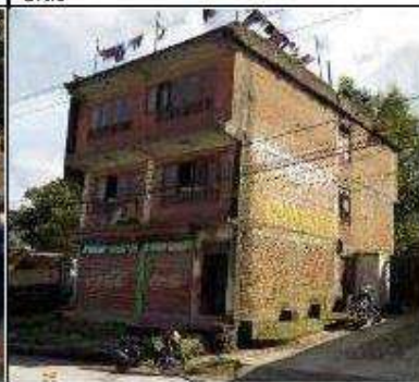
Structure No. 42: Dev Maya Maharjan, Mahadevsthan 1 Kha, Plot No. 287, RCC Frame Structure, Full Impact, 0+400, Left Side
