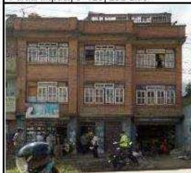
Structure No. 22: Hera Bahadur Maharjan, Mahadevsthan 1 Kha, Plot No. 337, RCC Frame Structure, Full Impact, 0+190, Left Side
