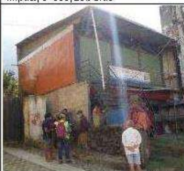
Structure No. 44: Apsara Maharjan, Mahadevsthan 1 Kha, Plot No. 289, Concrete Block and CGI Sheet Roof, Full Impact, 0+410, Left Side
