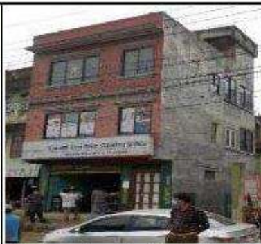
Structure No. 26: Bimal Shrestha, Mahadevsthan 1 Kha, Plot No. 242, RCC Frame Structure, Full Impact, 0+215, Left Side
