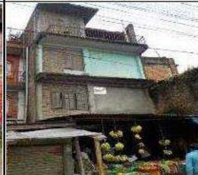
Structure No. 33: Nil Bahadur Maharjan, Mahadevsthan 1 Kha, Plot No. 364, RCC Frame Structure, Full Impact, 0+248, Left Side
