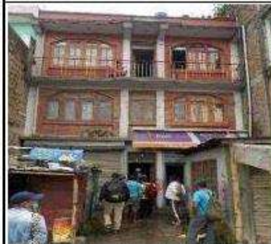
Structure No. 31: Gyani Maharjan, Mahadevsthan 1 Kha, Plot No. 261, 263, 342, RCC Frame Structure, Partial Impact, 0+240, Left Side
