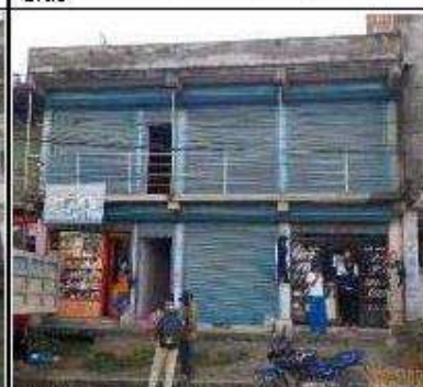
Structure No. 45: Maiya Maharjan, Mahadevsthan 1 Kha, Plot No. 372, RCC Frame Structure, Full Impact, 0+420, Left Side
