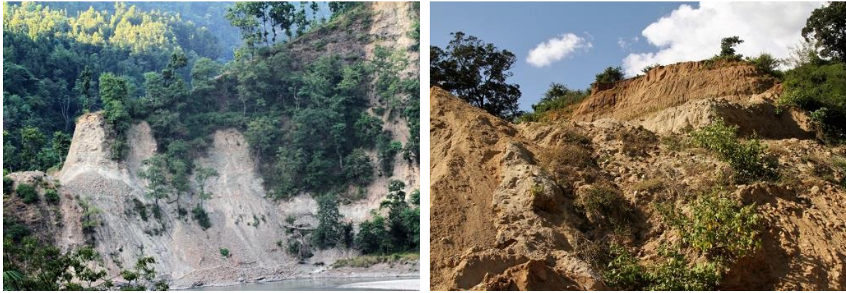
Figure 0-8: Landslide and instable slopes along NNM section.
