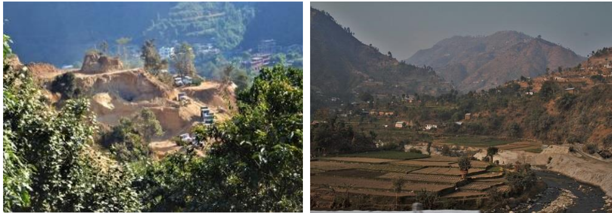
Figure0-5: Soil from project impacted area and water from Trishuli river will be used for construction.
