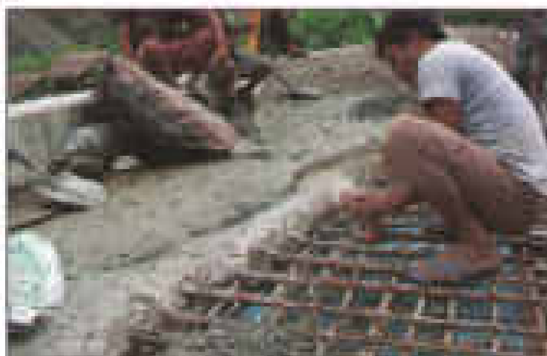
Fixing of reinforcement and concreting.
