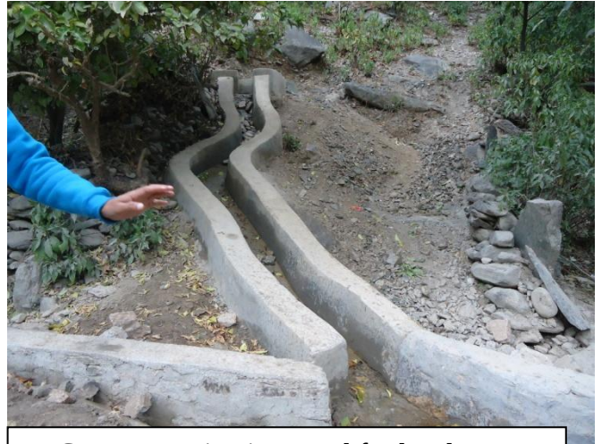
Construct Irrigation canal for locals as a example of good practice
