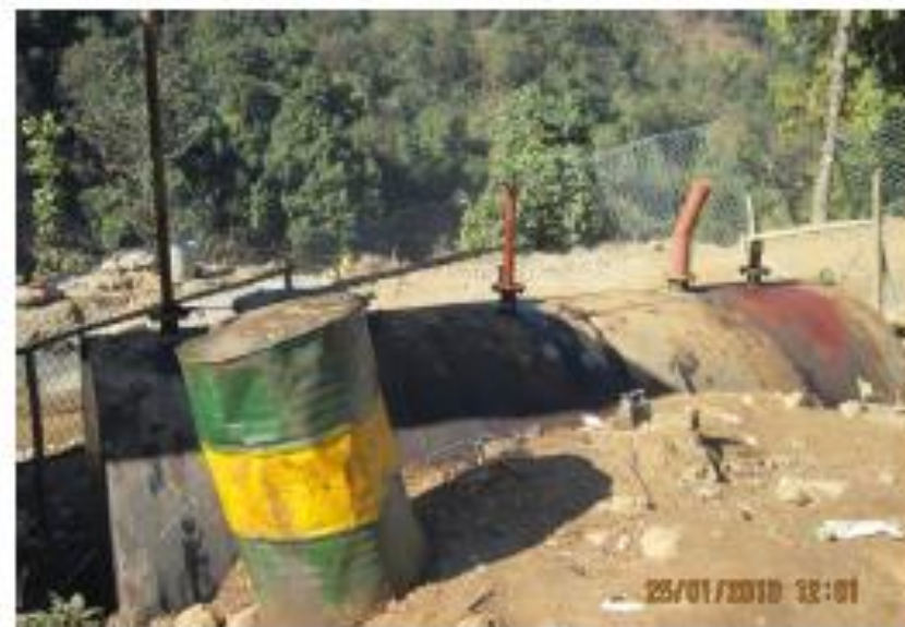
CJ4: Fuel stored in underground metal tank
