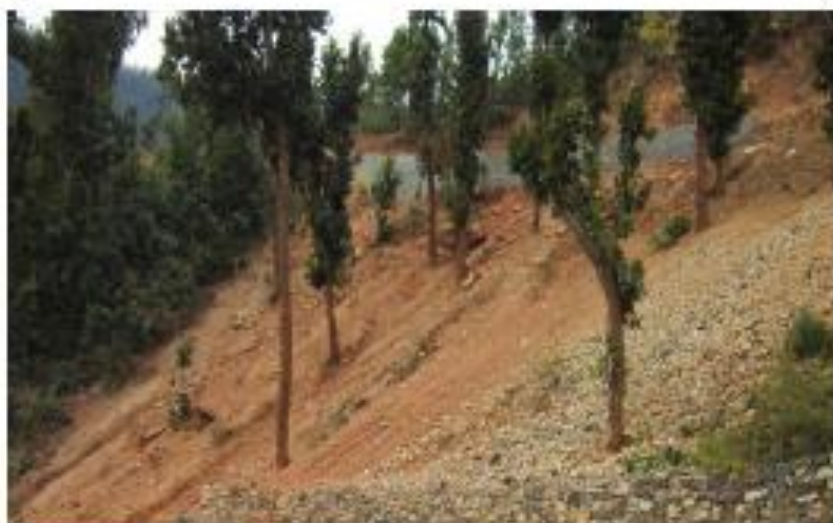
CJ5: Debris fallen from high above crossing the existing road at three different points
