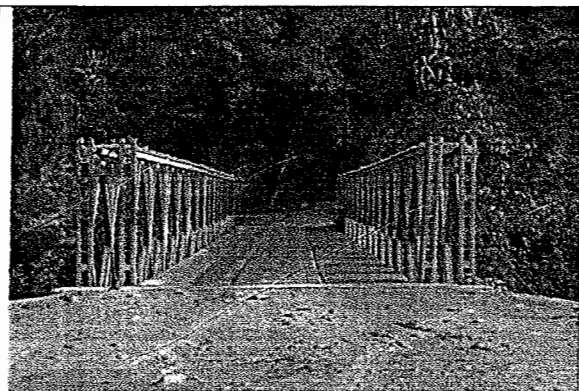
Photo 1: Existing Bailey Bridge over Kane Gadh Khola
