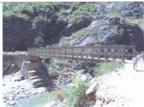
EXISTING TILA BRIDGE
