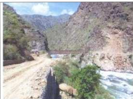
EXISTING TILA BRIDGE
