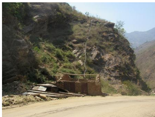
Private structures around the Bridge location
