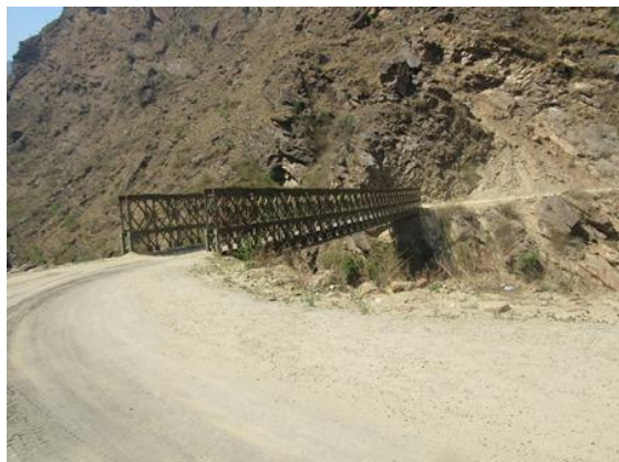
Existing Bailey bridge over Tila River
