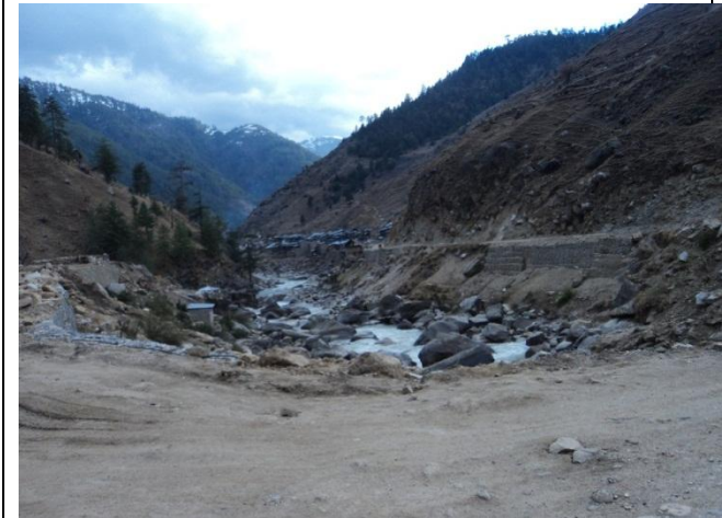
Photo 6: View of site for the construction of the bridge
