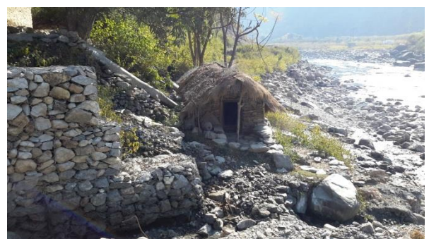
Figure 6.5: Water mill affected by the project.
