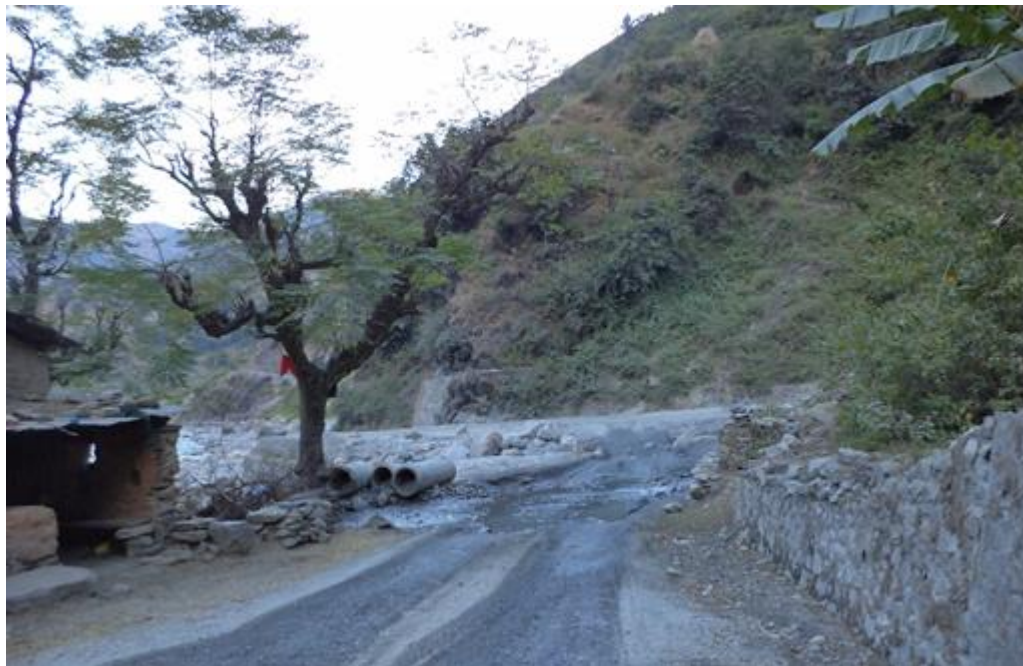
Figure 6.1: Photographs of proposed bridge location
