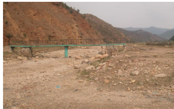
Figure 6-7: Bridge within Direct Impact area (30 m u/s from the proposed bridge location) of the Proposed Bridge
