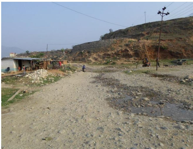
Electricity poles Likely to be Affected
