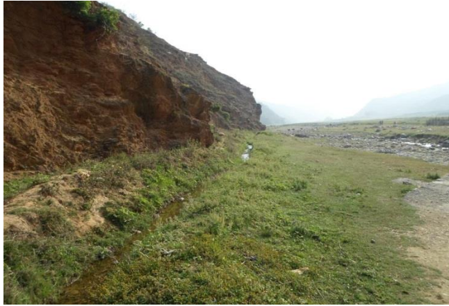
Irrigation Canal U/S of the Proposed Bridge Location
