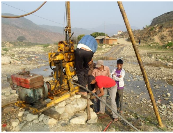
Photo 3: Water pump for water supply in the settlement
