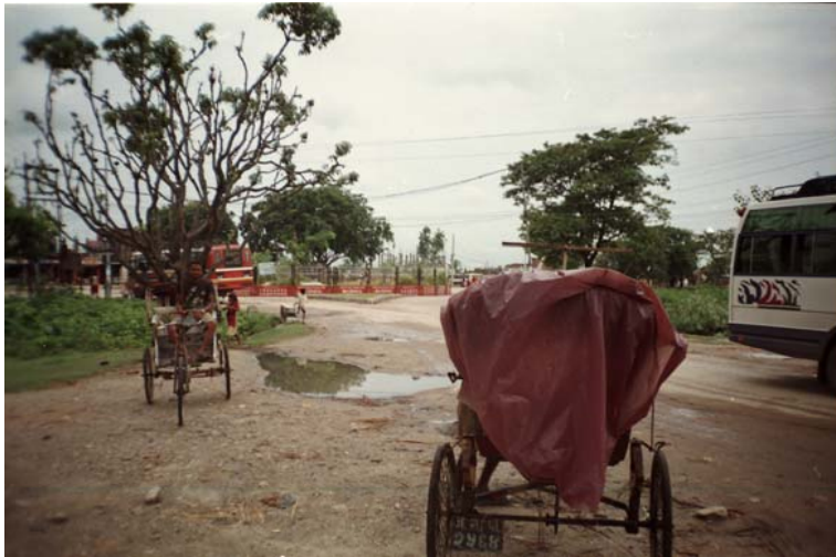
Photo 05: Road Condition at Janakpur
