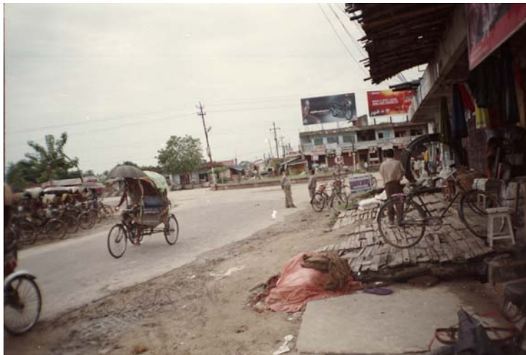
Photo 07: Road Condition at Janakpur
