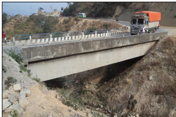
Figure 3: Sharp bends on the existing road at Khatripauwa
