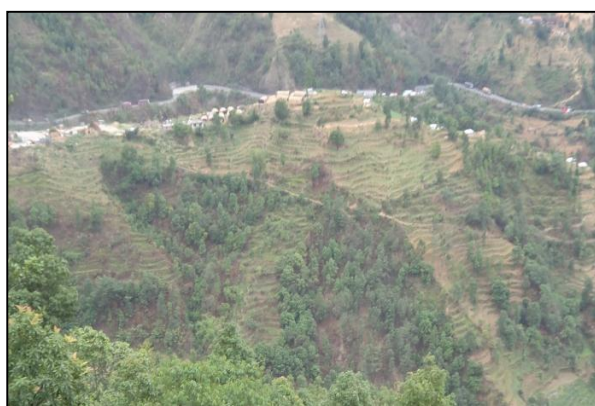
Sisne Khola Dharke road is aligned through old landslide at north of Chyaudanda
