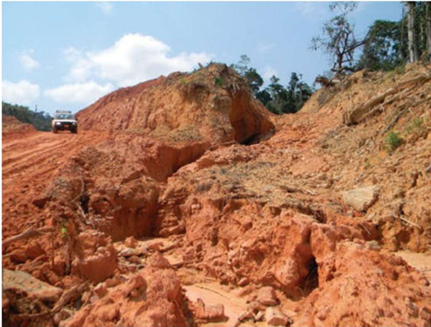
Figure D-10 Example of severe erosion in erodible/dispersive soils [11]
