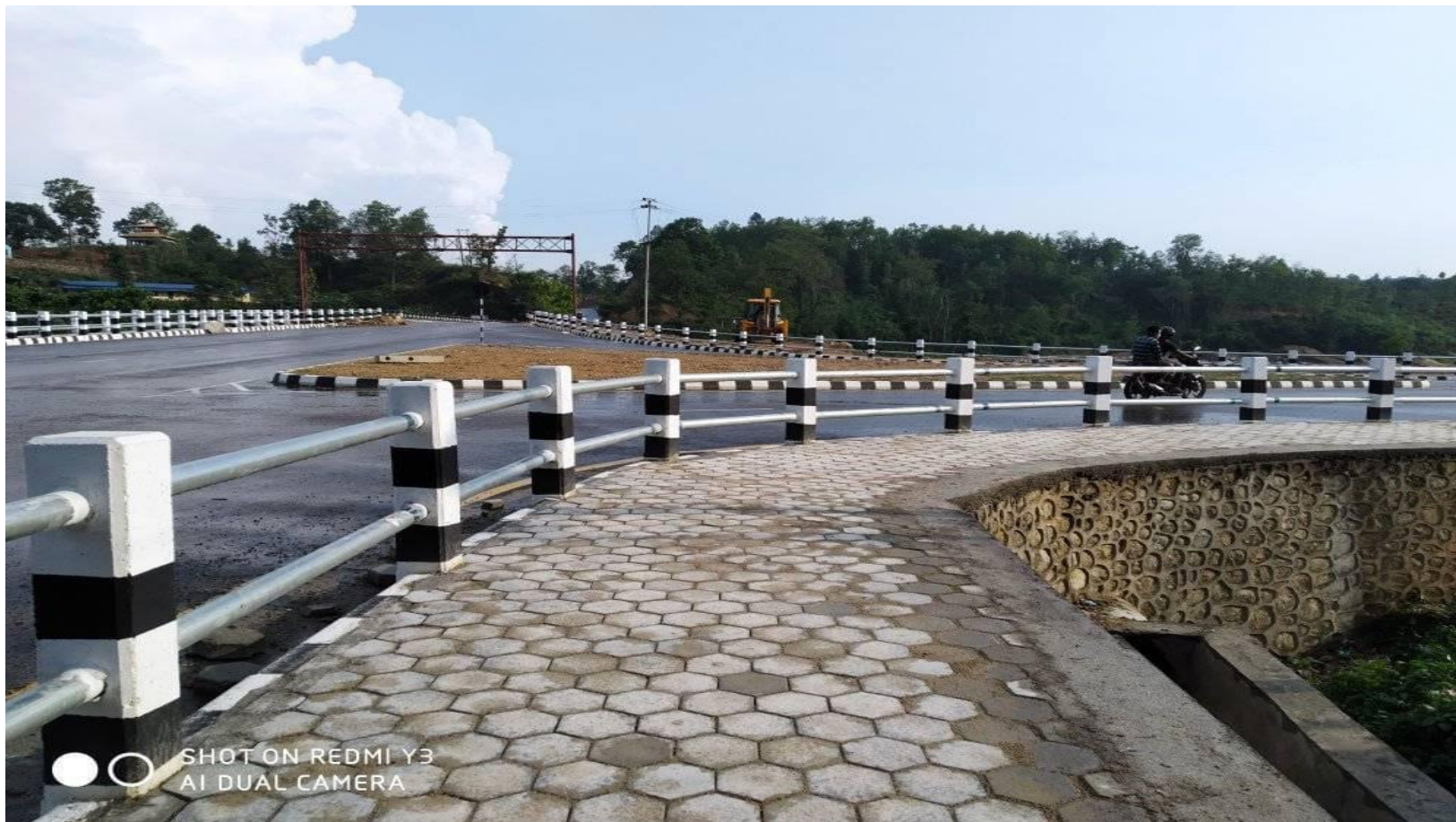
Intersection at Katari Bazar Chainage : 127+500
