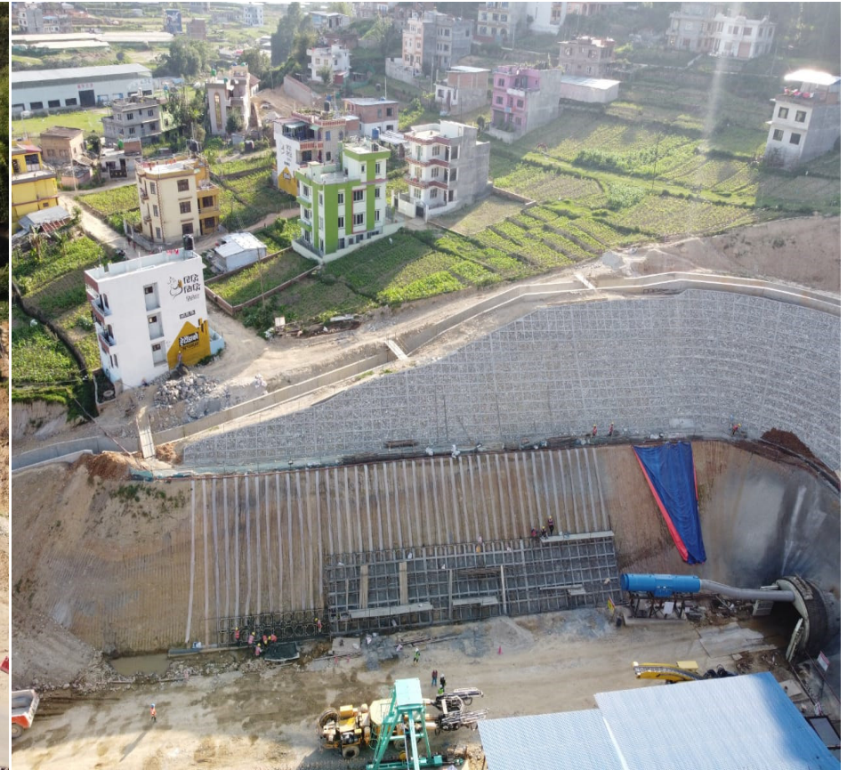
Photo 2: Crib Works at East Portal
