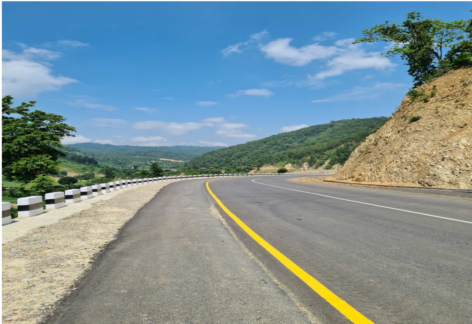
L-Beam Crash Barrier at chainage : 108+200 , Udayapur
