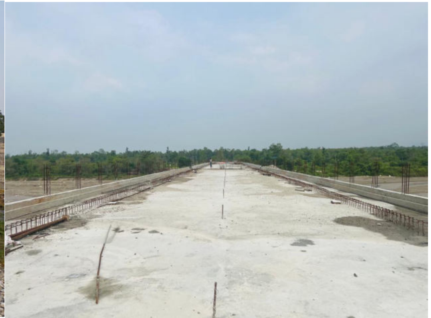
Completed Deck Slab of Ratuwa Khola Bridge
