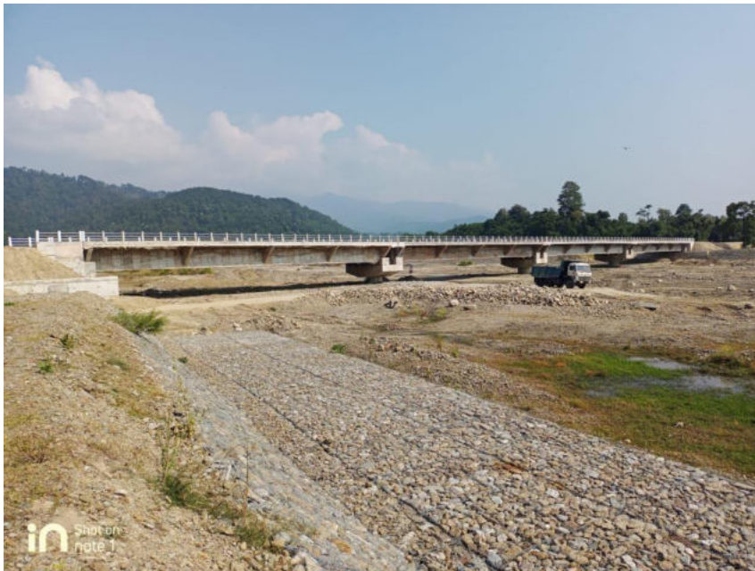
Completed Structure of Morangi Khola Bridge
