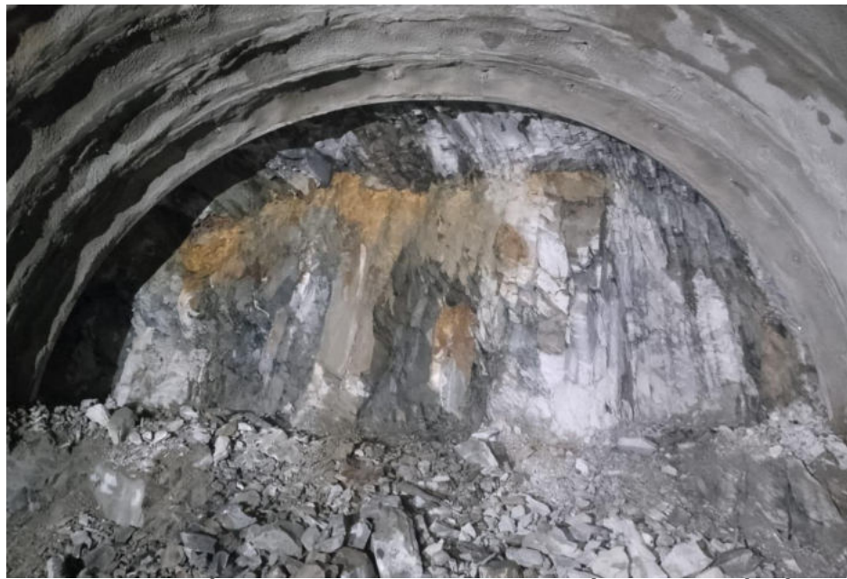
Blasting, excavation, mucking, steel rib installation and shotcreting
