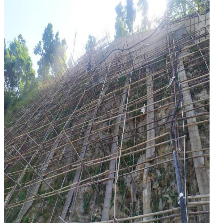
Shotcrete work, CH 2+160
