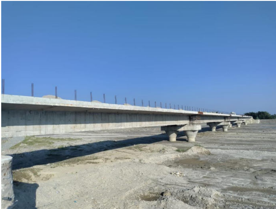
Completed Structure of Nusari Khola Bridge Morang
