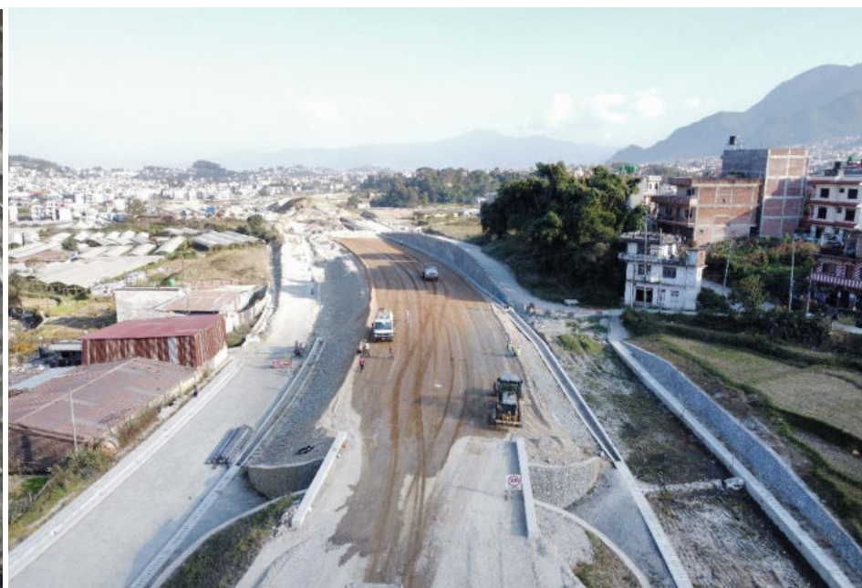
Approach road Construction
