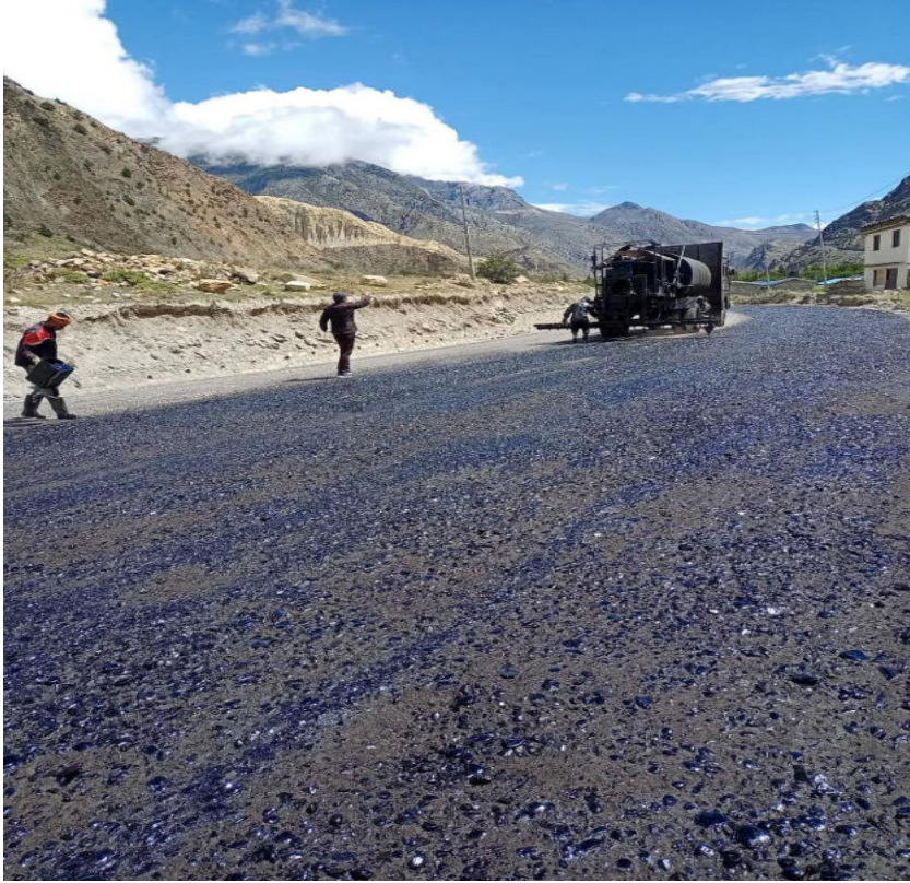
(Prime Coat, Near Marpha, Ch 35+150, घाँसा जोमसोम सडक खण्ड)
