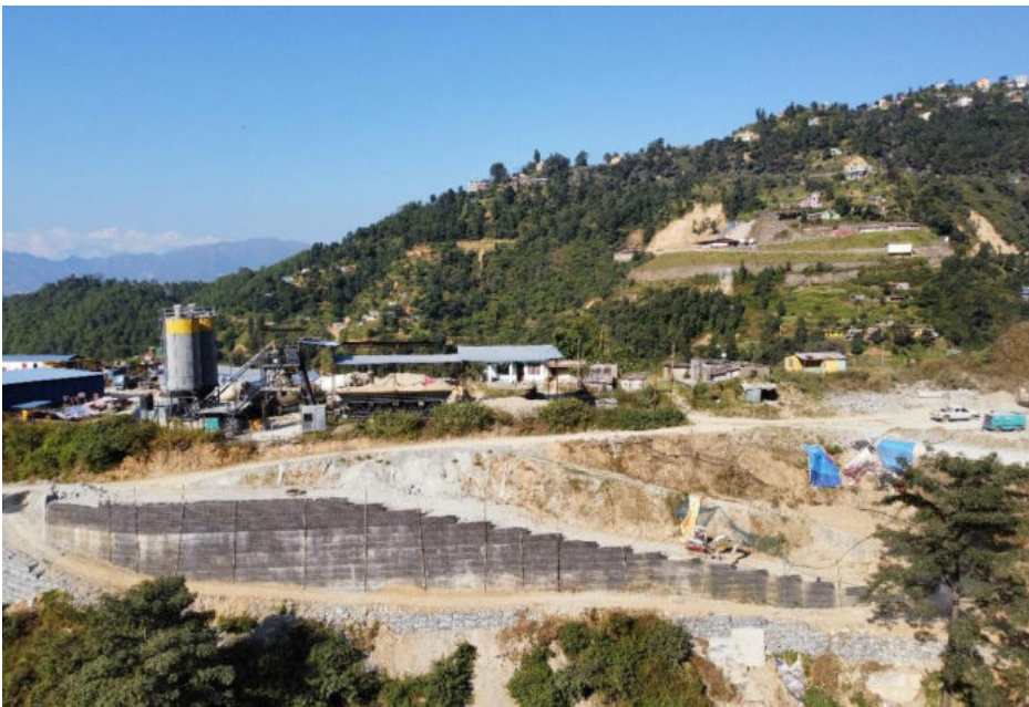
Reinforced Soil Wall Construction
