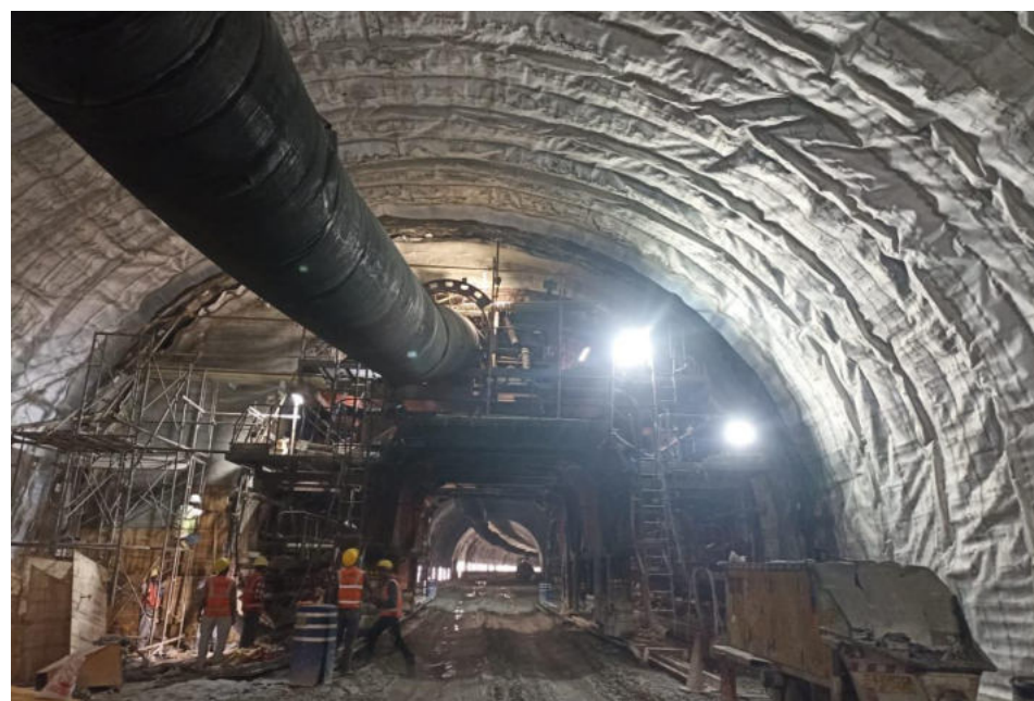
Tunnel Lining works
