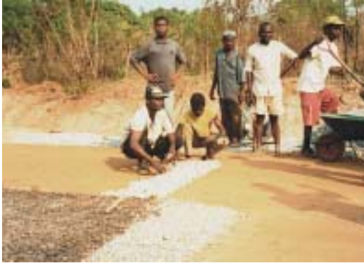
Plate 17 Largest aggregate placed by hand
