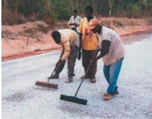
Plate 15 Sweeping excess chippings
