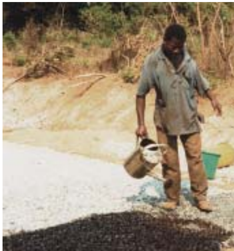
Plate 20 Application of emulsion binder
