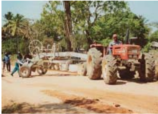
Plate 10 Tractor towed scarification
