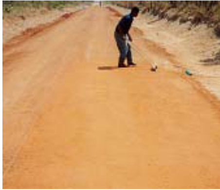
Plate 12 Brooming of surface
