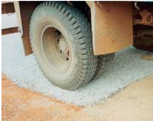
Plate 6 Lorry wheel compaction
