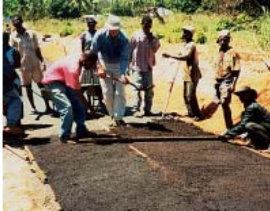
Plate 16 Placing of material between wooden batons
