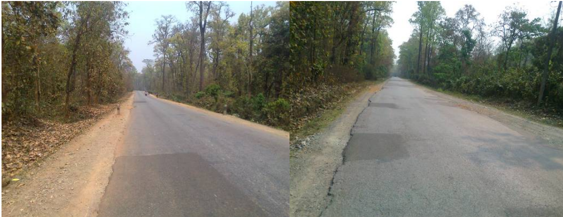
Wildlife crossing area at Ch 3+550
