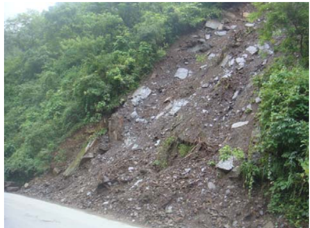
Landslide along the road.
