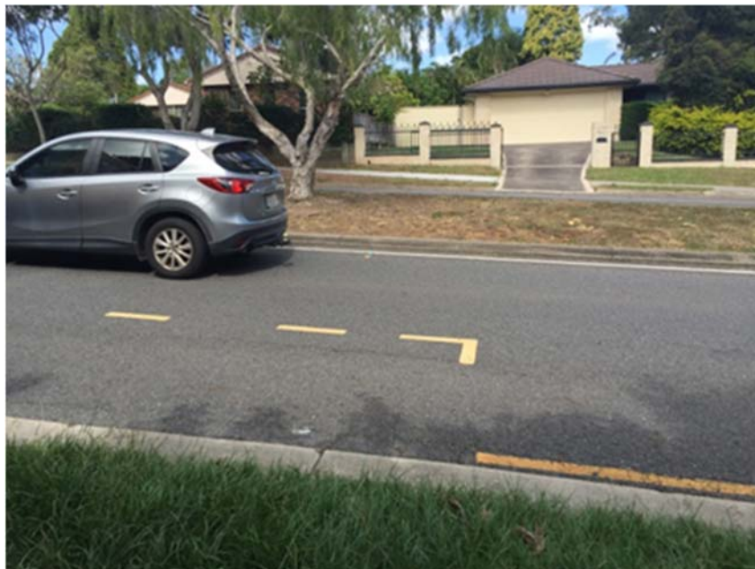
Figure 6.24: Yellow Bus Box at Bus Stops
