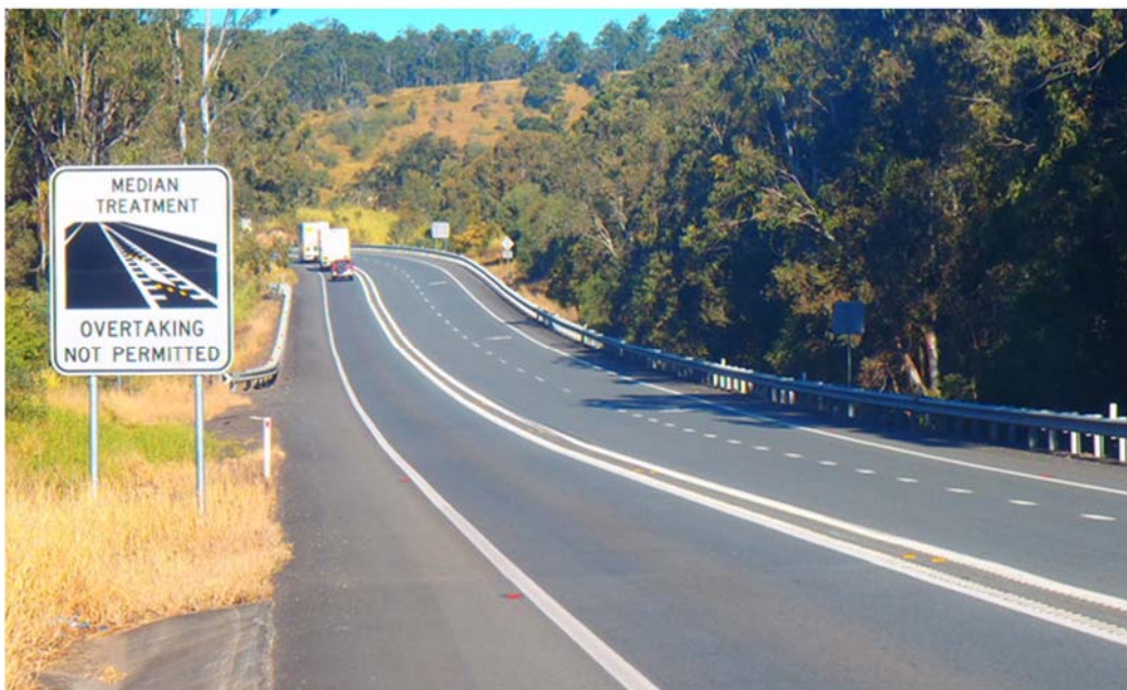
Figure 6.16: Illustration of Combination of WCLT and Passing Lane Treatment
