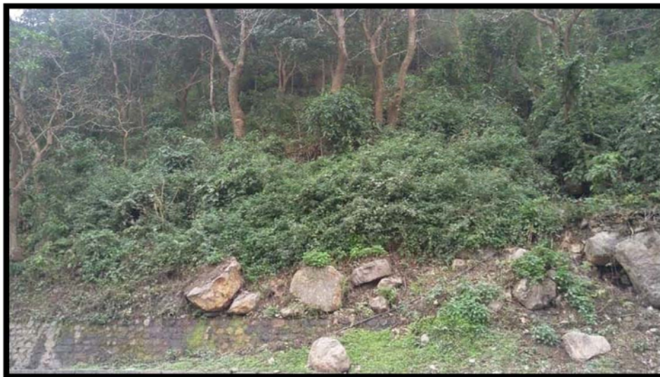
Photo 11: The colluvial cone along with the retaining wall and boulder in between Ch 8+850 to Ch 9+975
