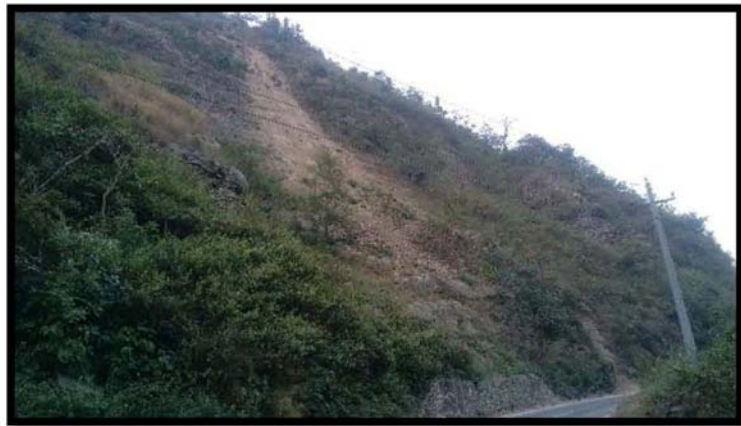
Photo 6: A minor recent rockfall at Ch 5+625 to Ch 5+650
