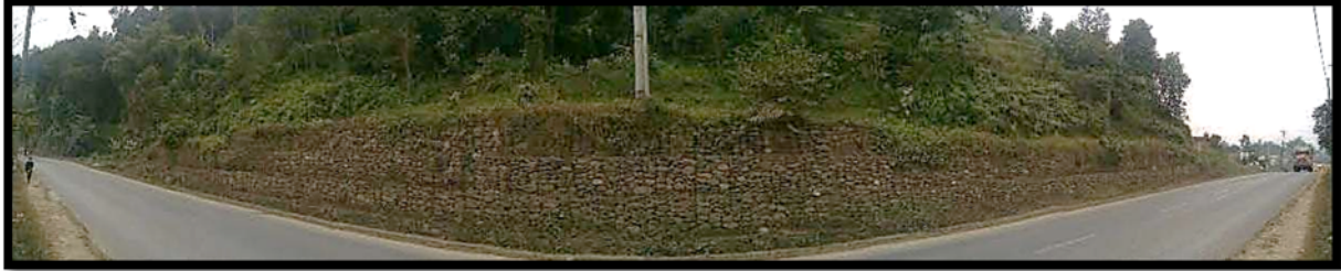
Photo 20: The gabion constructed to check the possible creeping of the thick residual soil near Thurpu
