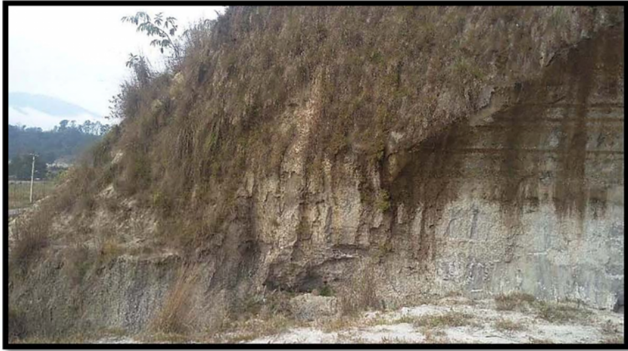
Photo 22: The hill lock consisting calcareous silty clay to clayey silt at Ch 59+675 59+700 to 60+900
