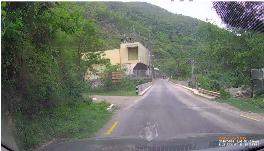
Photo 6.5: Delineation measures in the form Chevron Alignment Markers (CAMs) on the approach of the bridge is missing. Concrete posts or other simple delineation should be introduced on the near approach both sides to guide traffic to reduce the likelihood of vehicles hitting the bridge hand rails. Intersection approach and culvert head wall needs improvement. There is no terminal treatment on the W-Beam Guard Rail.
