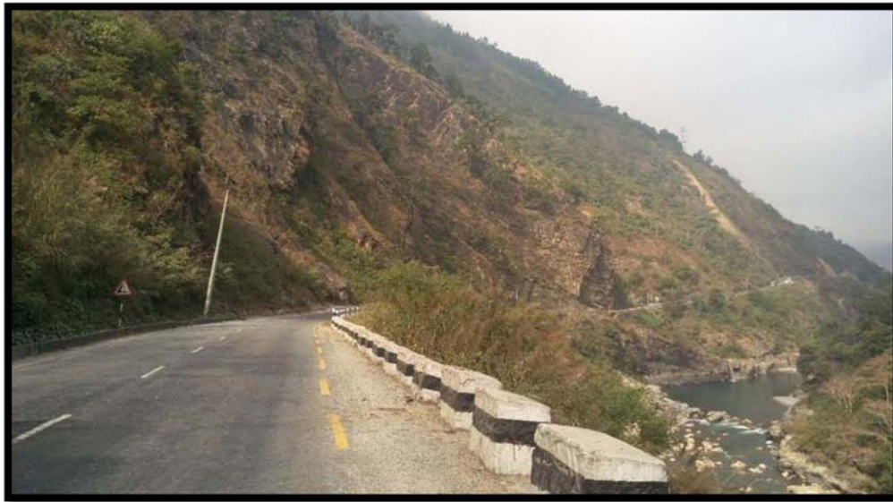
Photo 8: View between Ch 3+725 to Ch 5+875
