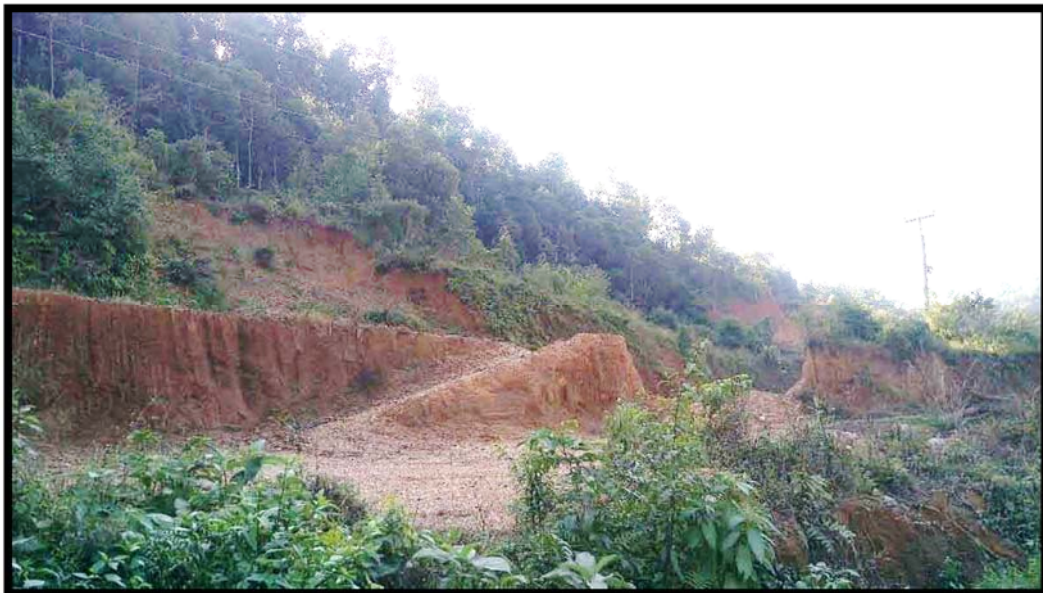
Photo 16: The exposed showing thick sequence of residual soil in between Ch 36+750 to 39+175 39+175 to 39+200
