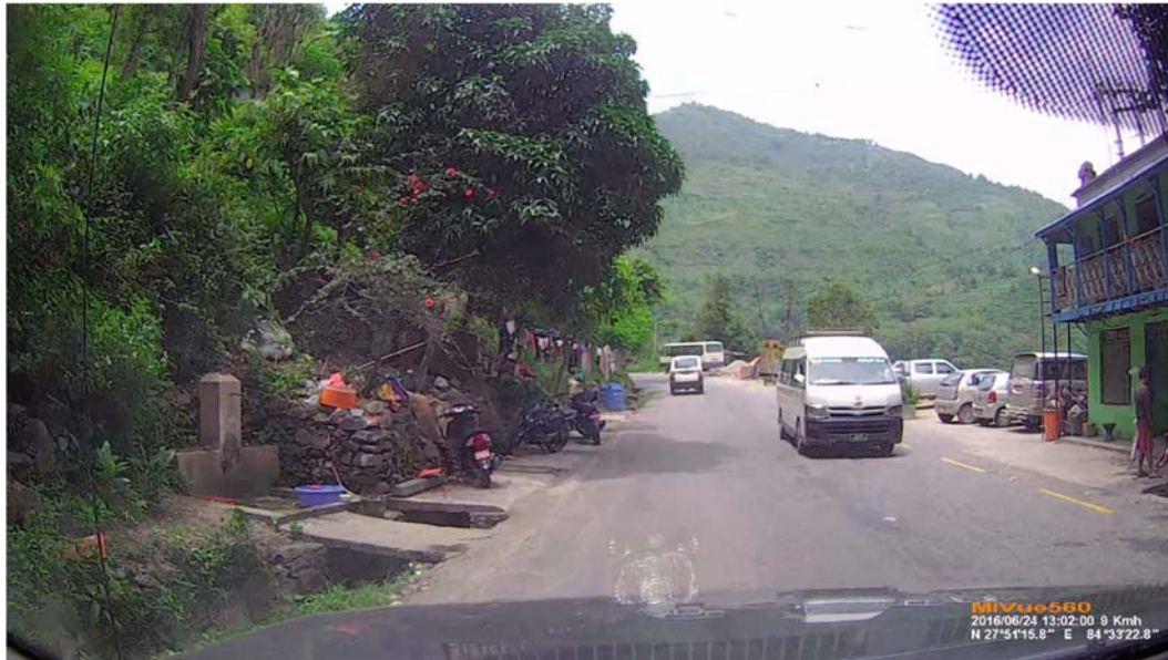
Photo 6.2: Road in Nepal is not just for transport. This is also a place for washing and cleaning. On the right steep fall calls for installing RCC crash barrier. Widening is possible by cutting hill side. On the right, side drains should be covered and water spout should be managed to satisfy both safety and drainage
