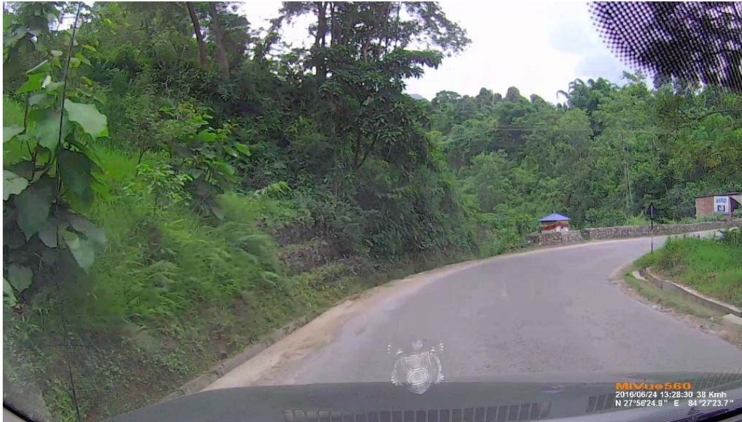
Photo 6.6: Another example of potential site for delineation measures on either side of the curve and either ends of high fills above waterway. When the road will be widened and culvert extended or replaced, its parapet wall must be raised to the standard height of RCC barrier with hazard markers on both ends.
