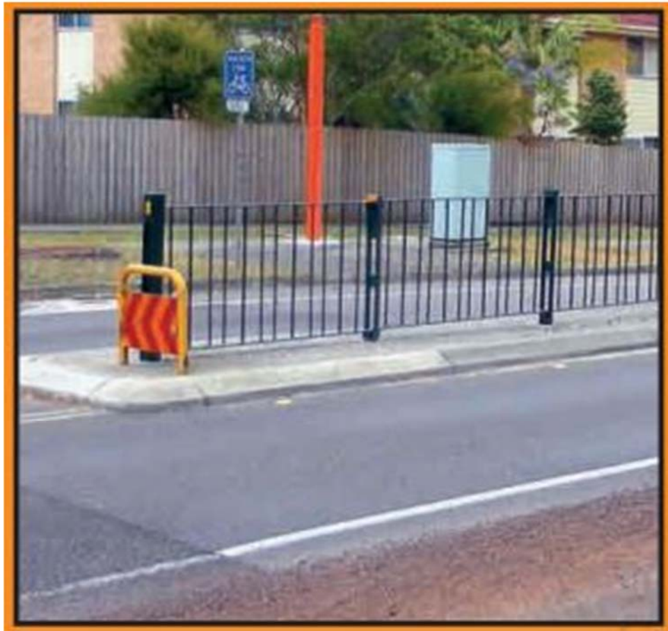
Figure 6.20: Vandal Proof Median Fencing
