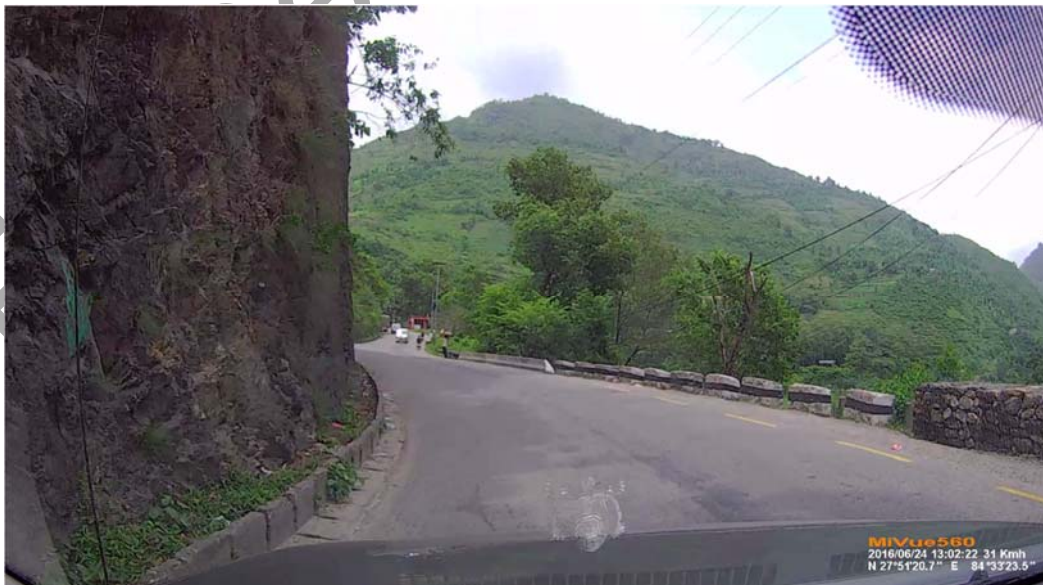
Photo 6.1: This could be typical candidate section for continuous RCC roadside crash barrier. Potential run off crash can trigger mass casualties due to large depth of drop on river side. Use of confidence block can guide the vehicles but cannot stop errant vehicles from Road widening is possible by cutting hill slope.
