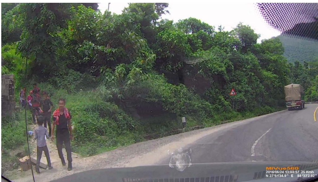
Photo 6.4: Multiple safety problems (a) Deep drain on left is road side hazard (b) Deep drop on the right is highly hazardous (c) Pedestrian Intrusion on road at blind spot (d) No center line marking on blind turn (e) Narrow shoulder
