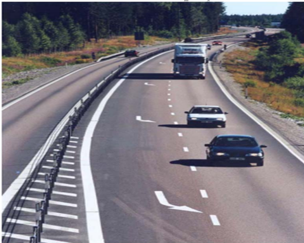
Figure 6.19: Example of 2+1 Treatment with Median Fencing
