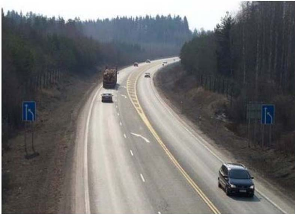
Figure 6.18: Example of 2+1 Treatment without Median Fencing
