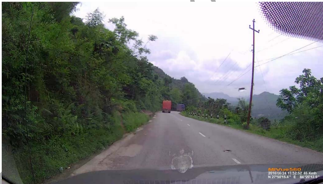
Photo 6.7: This is a typical section of PM Road where the fill slope can be made recoverable (1:4 or flatter). In this section, frangible delineation posts will be advantage to guide traffic along the bend. On the left, deep side drain is a safety concern.
