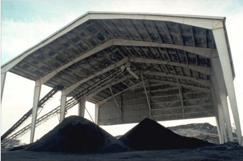
Figure 4.8 Covered aggregate stockpiles.
