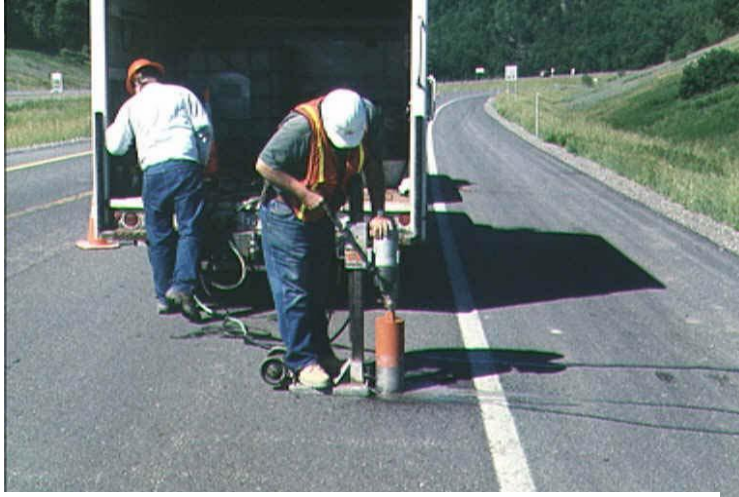
Figure 6.4 Coring hot mix asphalt
