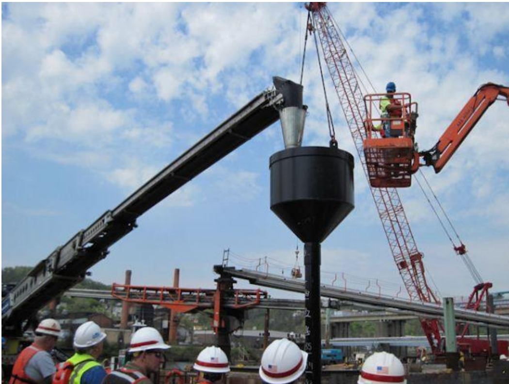
Figure 3.1 Tremie Concreting Method
