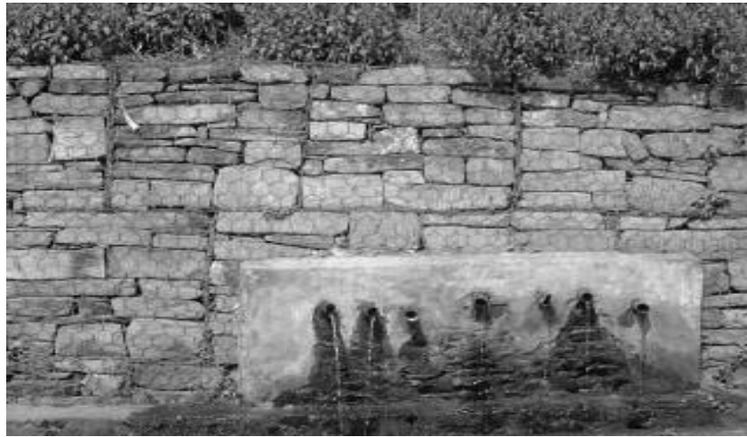
Figure 3.8: Horizontal Drilled Drain
