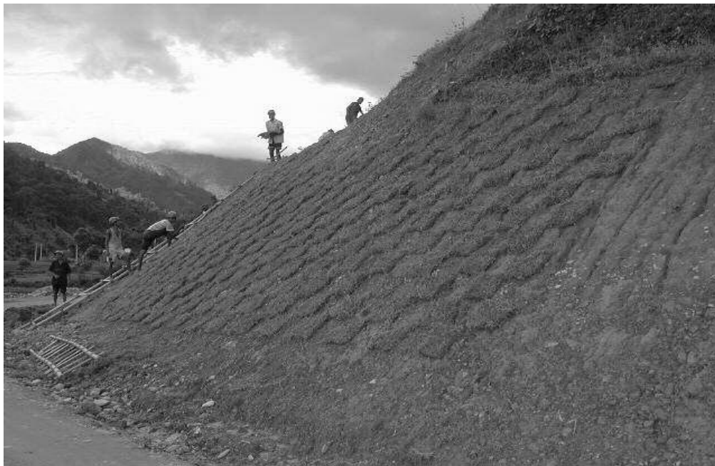
Figure 3.5: Example of Turfing in Cut Slope (Banepa- Sindhuli- BardibasRoad)
