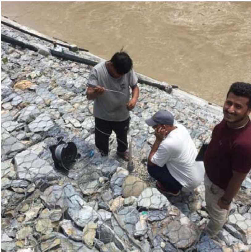
Piezometer test at Km 17 of Narayanghat Mugling Road
