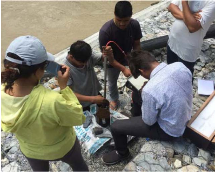
Inclinometer test at Km 17 of Narayanghat Mugling Road
