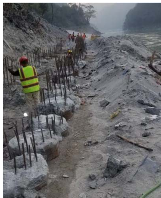
River training works at Km 17 of Narayanghat Mugling Road based on Piles
