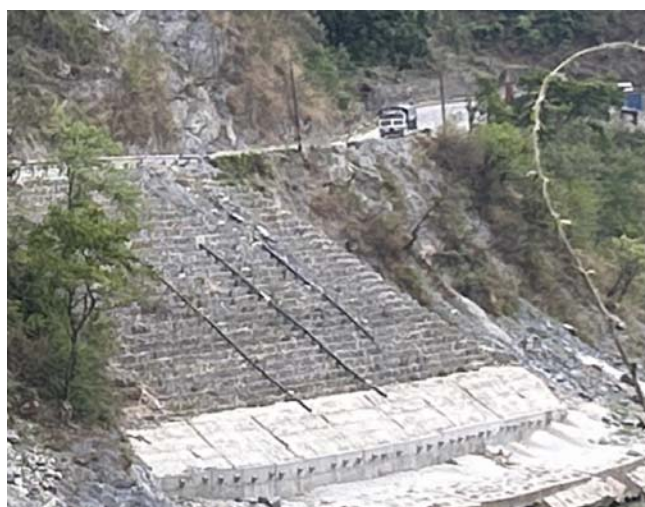
River training works at Km 17 of Narayanghat Mugling Road based on Piles
