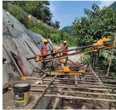
Example: Km 26 of NM road using Soil nails in retaining structures
