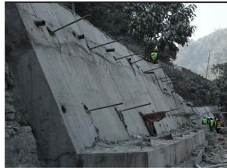
Example: Km 26 of NM road using Soil nails in retaining structures
