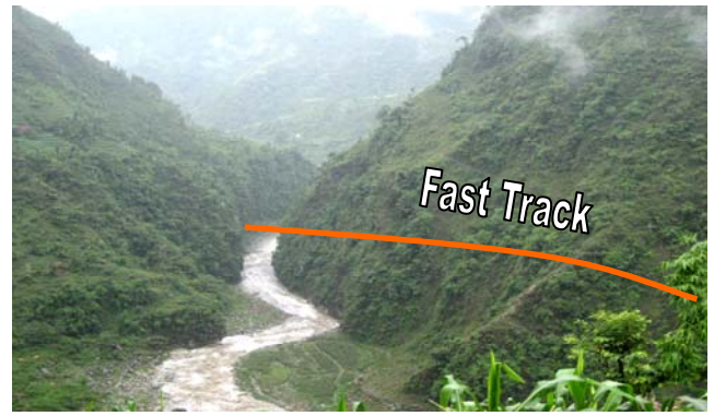
Photo: Road alignment passing through steep hill slope of Bagmati at Ch. 24+000.
