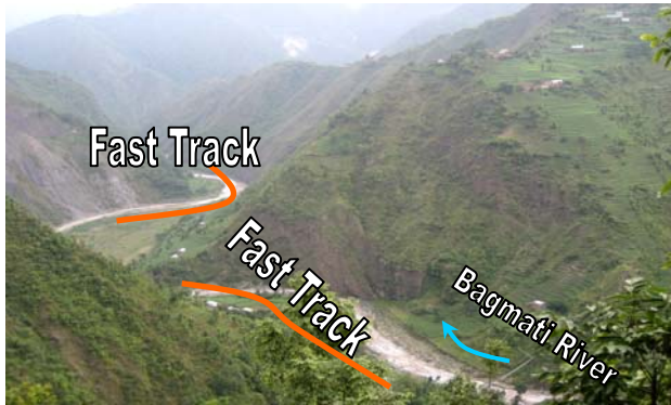
Photo : View of Bagmati Valley between Ch. 13+000 and Ch.15+000
