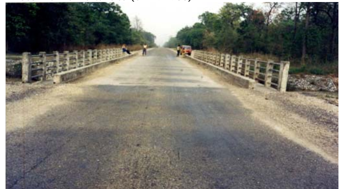
Photo: Existing Road Alignment of MRM. Nijgadh - Pathaiya Section
