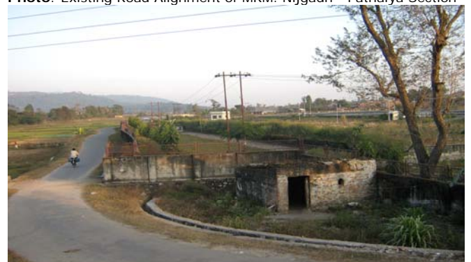
Photo: Part of the wastewater treatment plant where the Hetauda connector joins Tribhuvan Rajpath.
