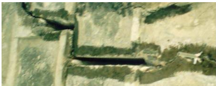
Photo 3, View of Cracks at the arch slab from below
