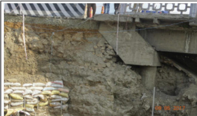
(c) Existing Bridge foundation exposed
