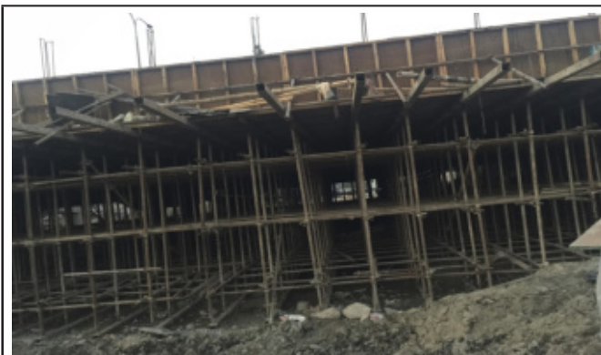
(e) Scaffolding work for deck construction
