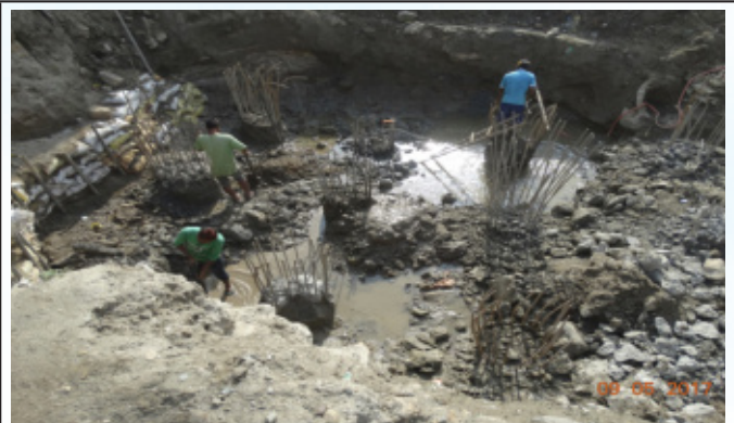
(b) Construction of pile foundation
