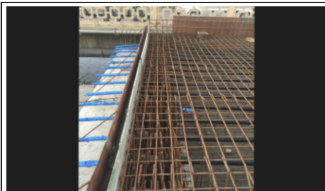
(g) Dead-end anchorage details
