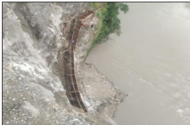
Fig. 16: Preparation for wall base with dowel bars
