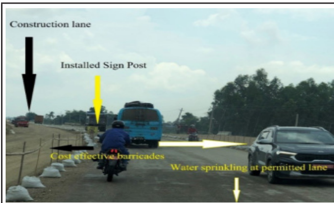
(c) Barricades for road safety and dust control at KK road
