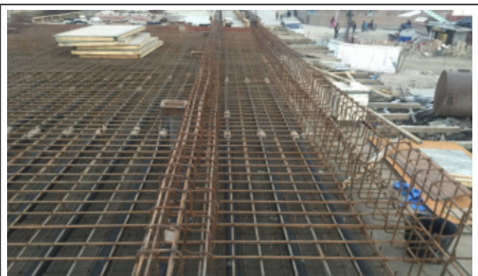
(f) Reinforcement placing and duct profiling
