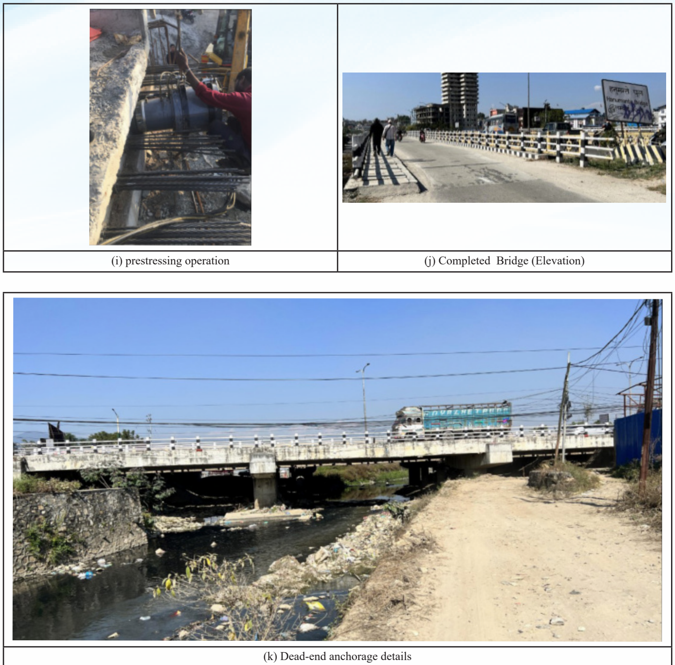
Fig.3- Photographs of construction sequence of Bridge
