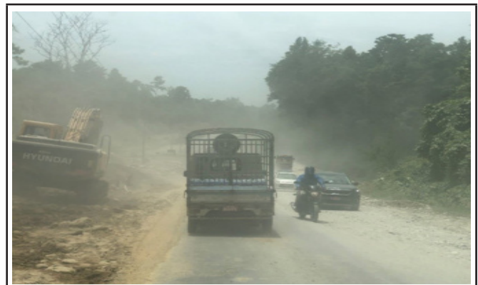
(d) Upgrading of side lane without barricading at NB road
