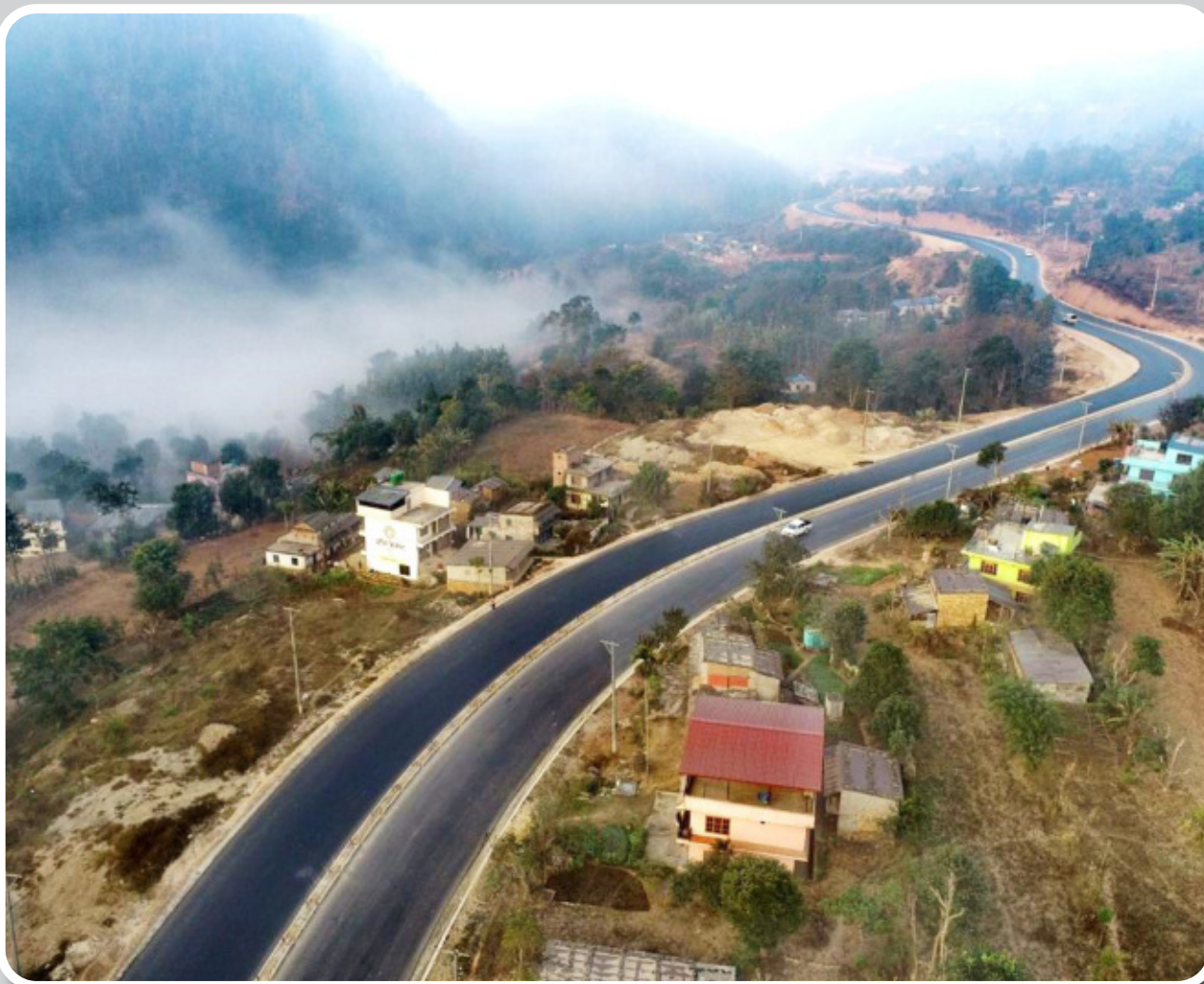
On-going construction Work along Mugling-Pokhara Road
