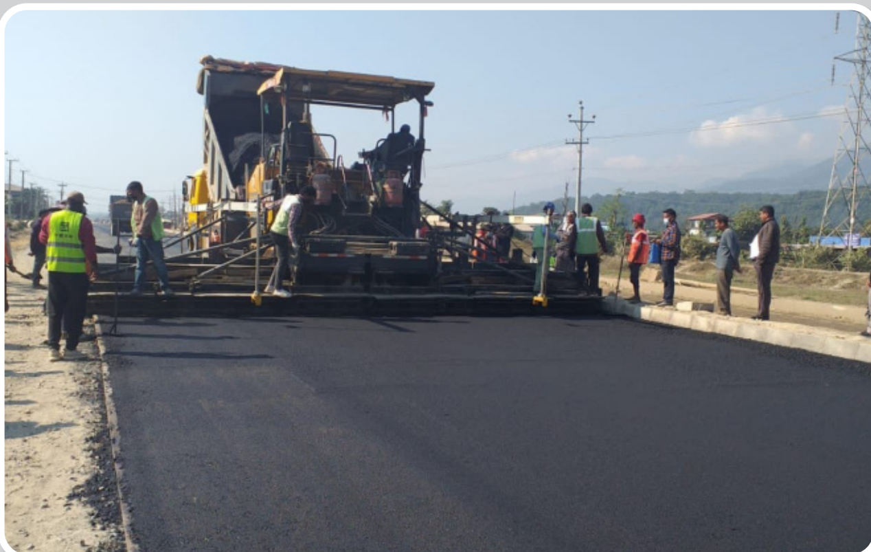
On-going construction Work along Narayanghat-Butwal Road
