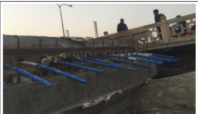
(h) Deck concreting and prestressing cable placement
