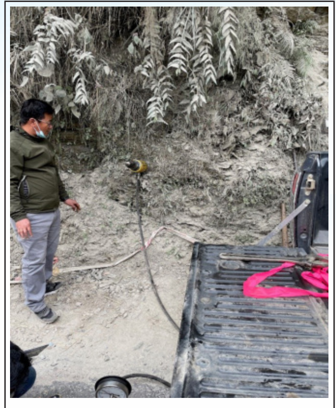
Fig. 10: Pull-out test of grouted rock anchors at the field.
