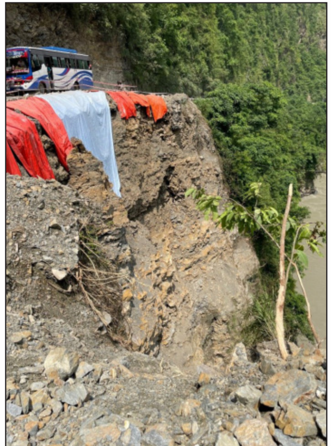
Fig. 3: Rock type, exposure, failed slope of damaged Road section of Mugling-Aabukhaireni section of Road (Km 86+050)
