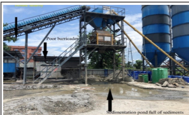
(g) Batching plant with sedimentation pond at NB road
