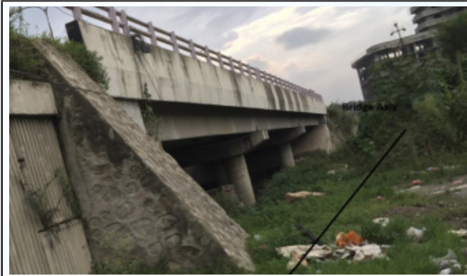
(a) Bridge site before construction begins
