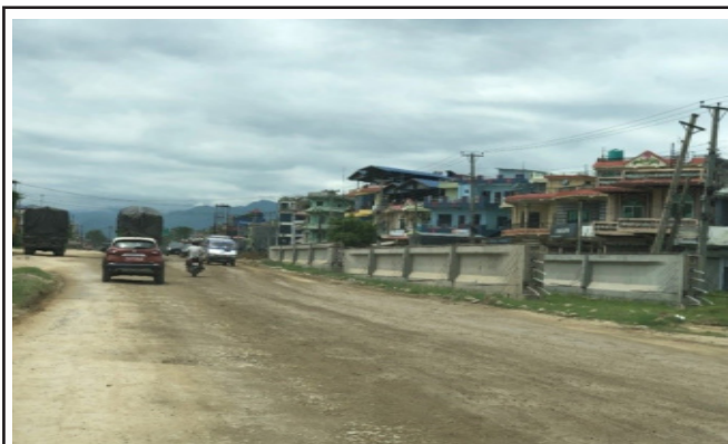
(e) Water Sprinkling at settlement area at NB road section
