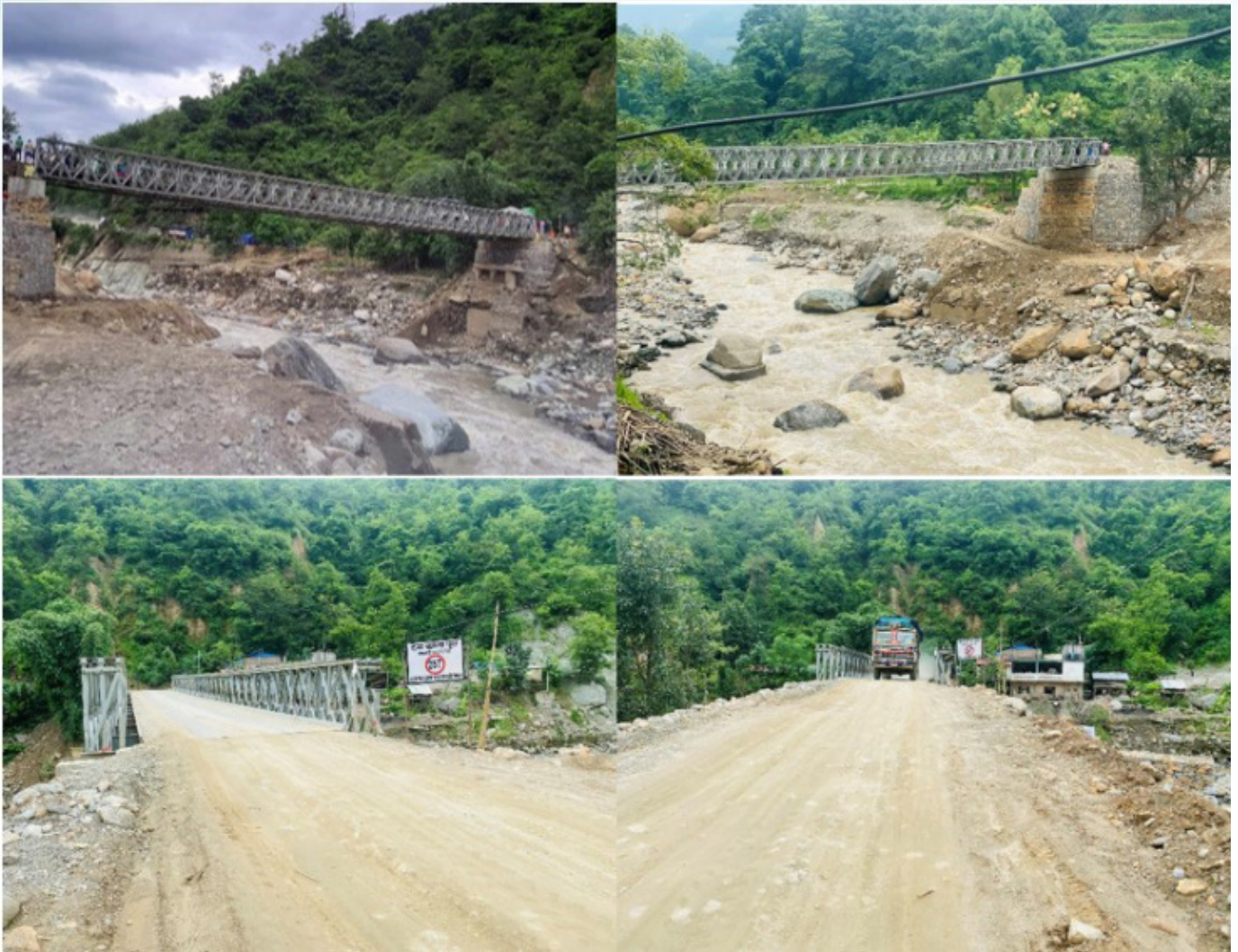
Fig. 8: Some pictures of the bridge site are included, showing the site before the damage, after it was damaged, and during the installation of the modular bridge.
