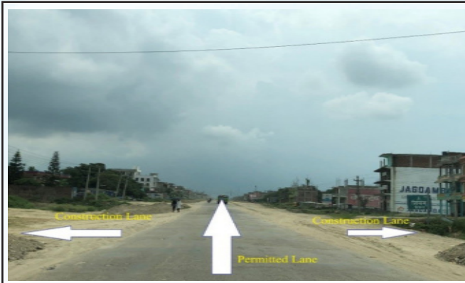
(a) Lane Management at KK Road
