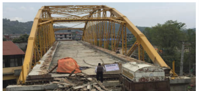
(h) Deck concreting
