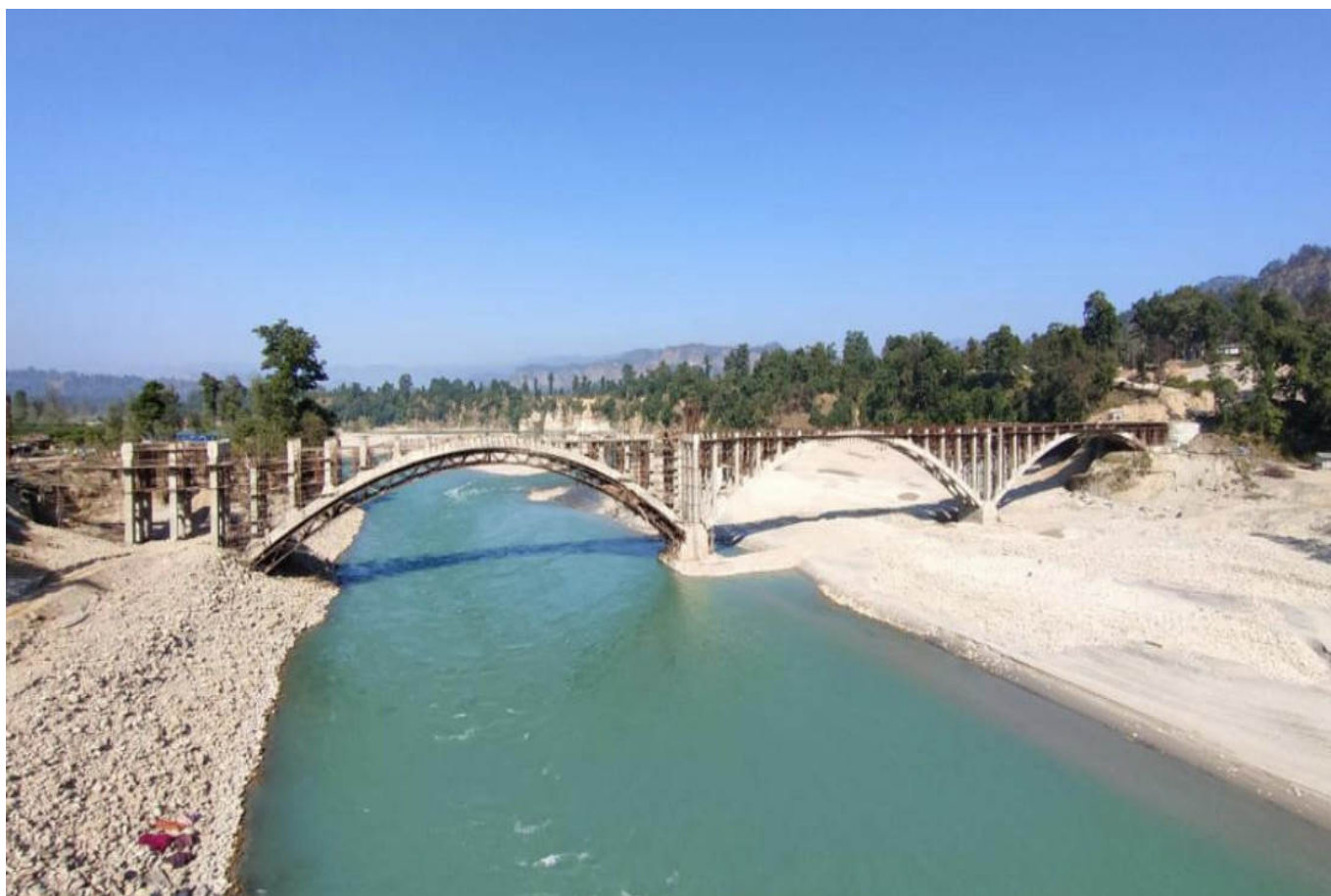
Karnali Arch Bridge, Kachalighat, Kuine (Under Construction)
