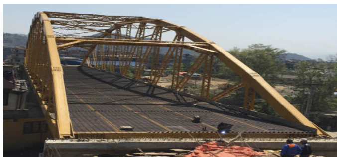
(g) Deck reinforcement
