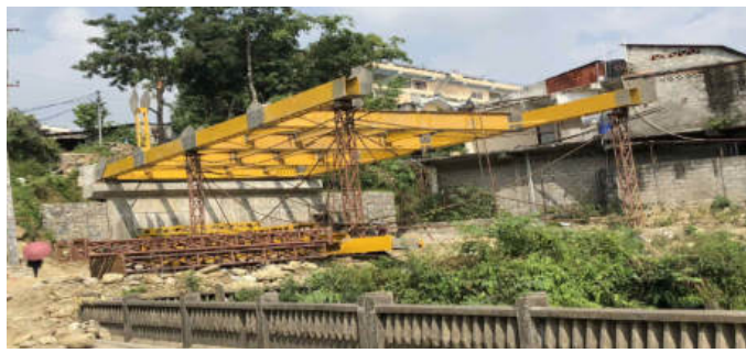
(c) Truss erection- Bottom chord, cross girder and stringer
