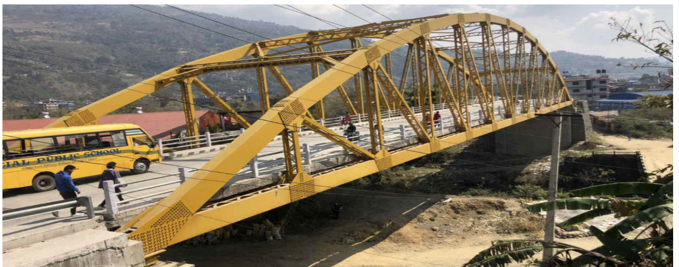
(i) Completed Bridge
