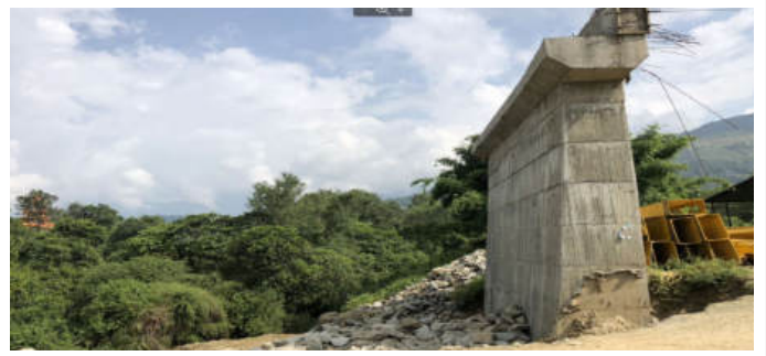
(b) Construction of abutment
