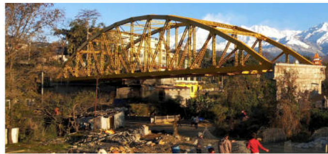
(e) Truss erection-remaining portion
