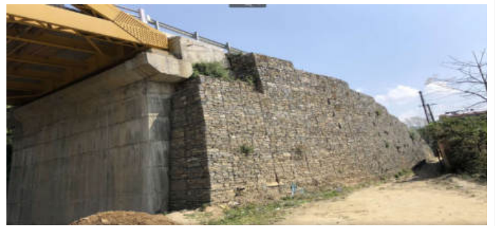
(f) Construction of wall (12.7 m)
