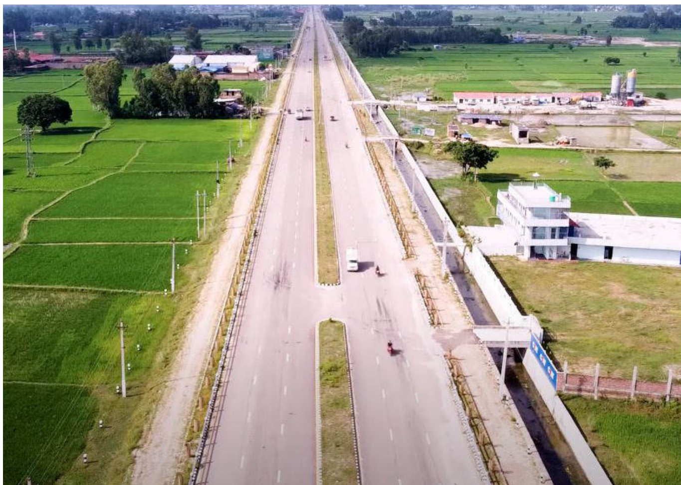
Dhalkebar-Janakpur Six Lane Road, Dhanusha Ch: 22+080 to 24+720 (Mahendranagar-Dhalkebar section)
