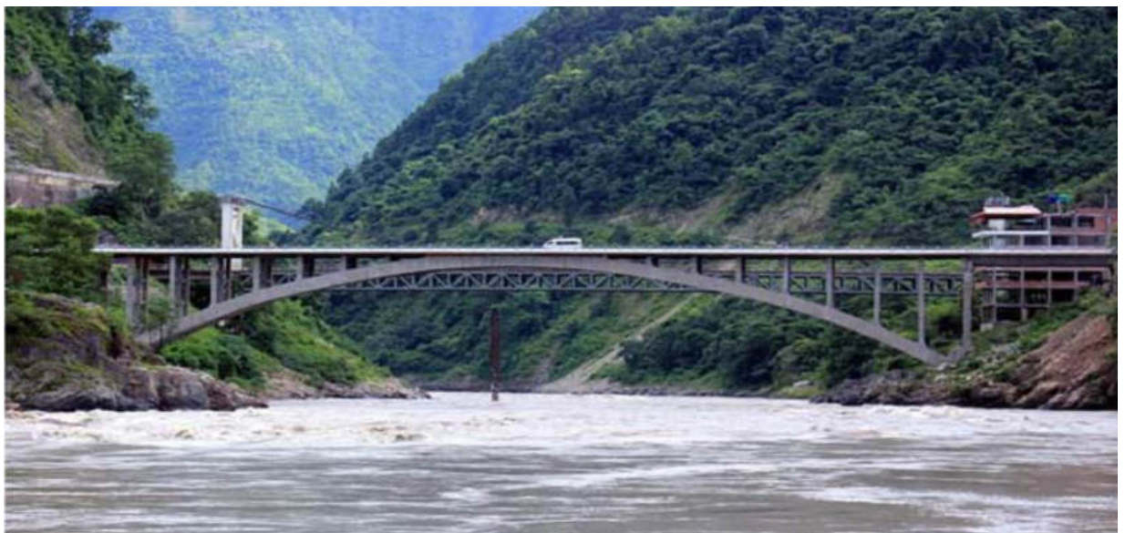
Fig.4 (b) - Construction photograph of Bridge Site
