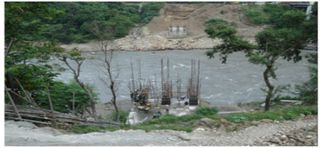
(b) Construction of Arch block/foundation
