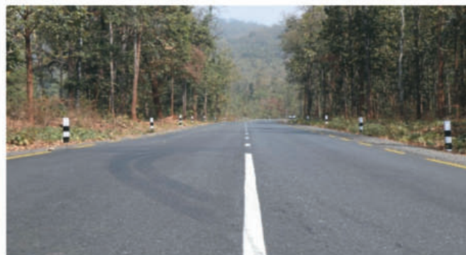
Road Alignment chainage 93+500, Madan-Bhandari Rajmarg, Udayapur
