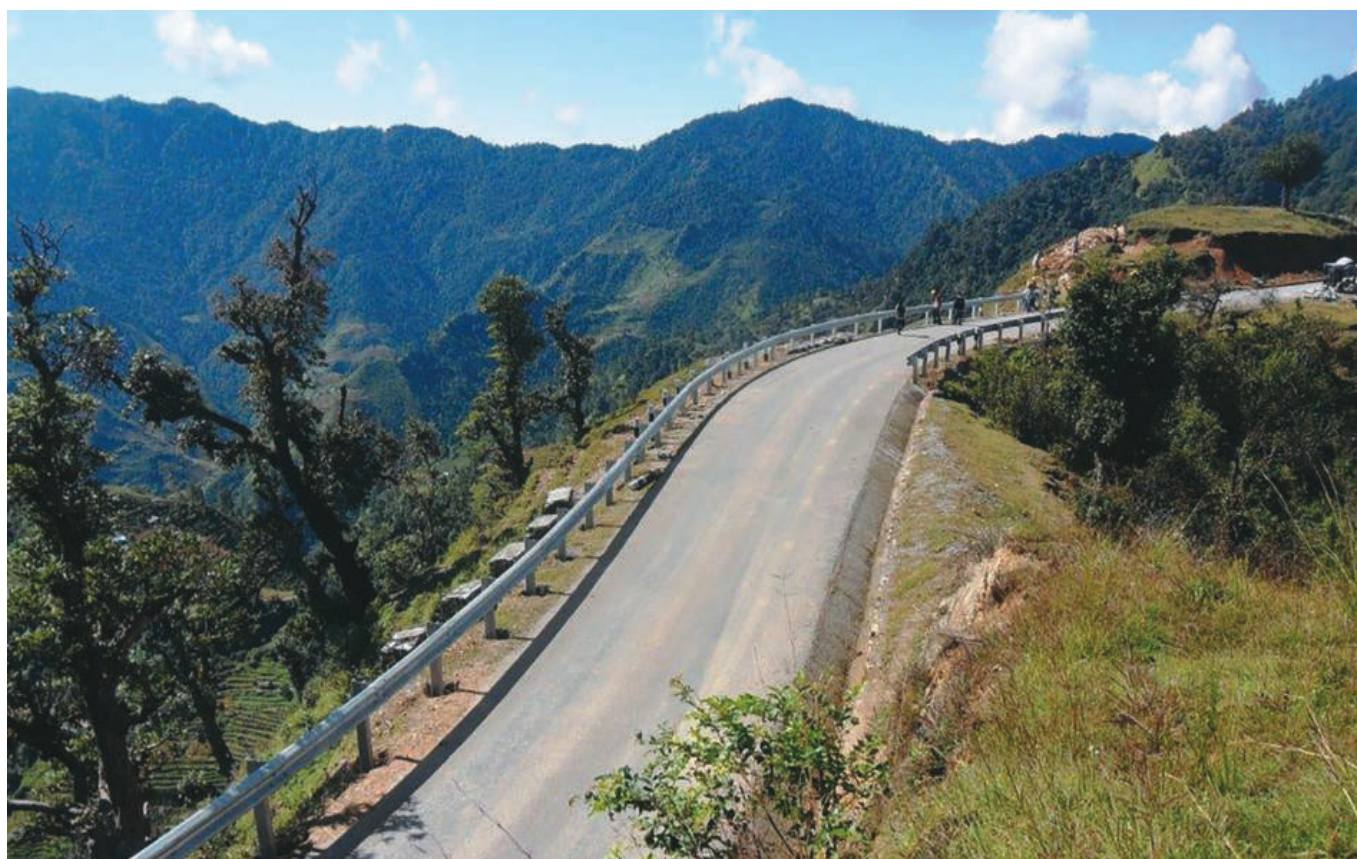
Road Safety Barrier (W-Beam type) at Khodpe Bajhang Road.
