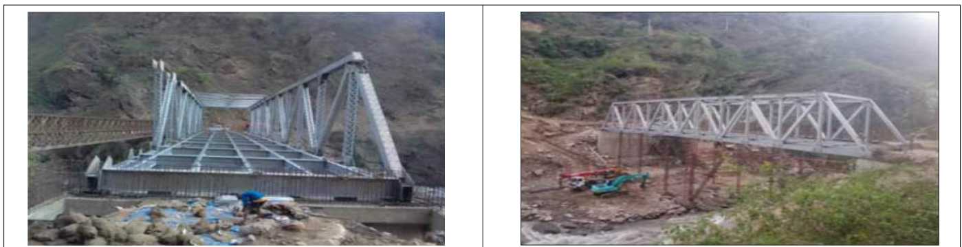
Fig 4: Superstructure construction photographs
