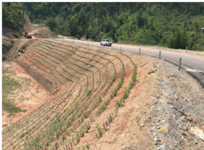
Bio-Engineering (Madan-Bhandari Rajmarg, Bhiman-Sindhuli Road Section)
