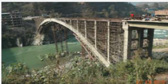
(g) Construction of arch deck slab
