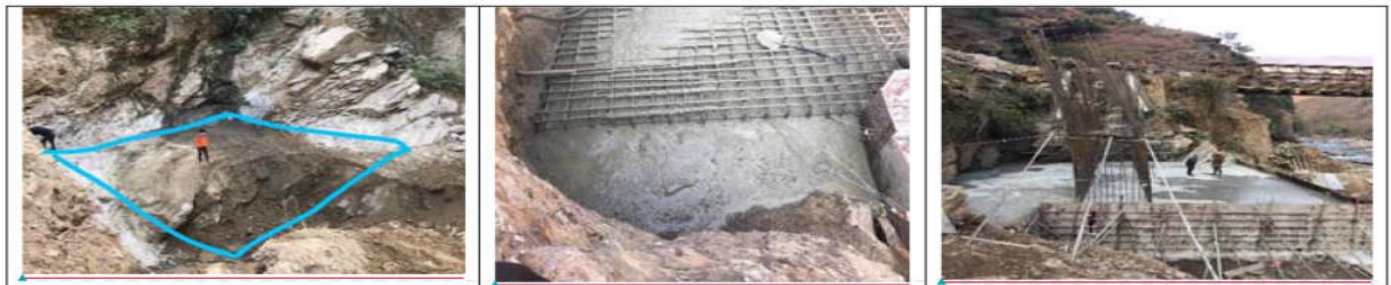
Fig 3: Foundation construction photographs
