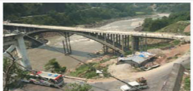
(h) Completed bridge
