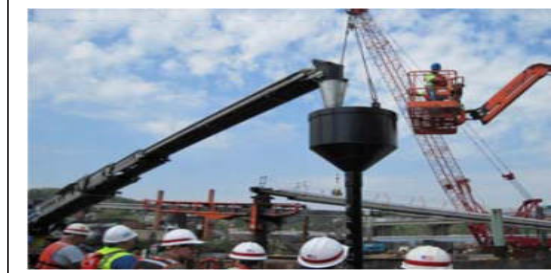
Fig.7-Typical field arrangement of Tremie Concreting of Pile
