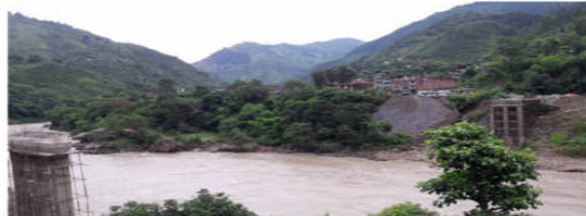
(c) Construction of side spans
