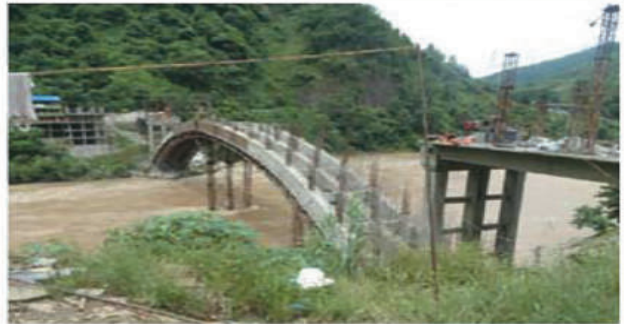
(f) Construction of arch rib and spandrel column
