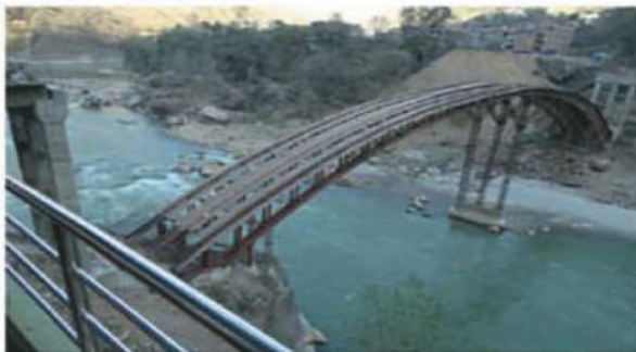
(e) Construction of temporary work for arch erection
