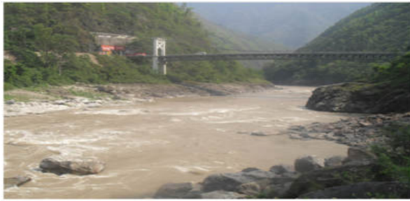
(a) Bridge site
