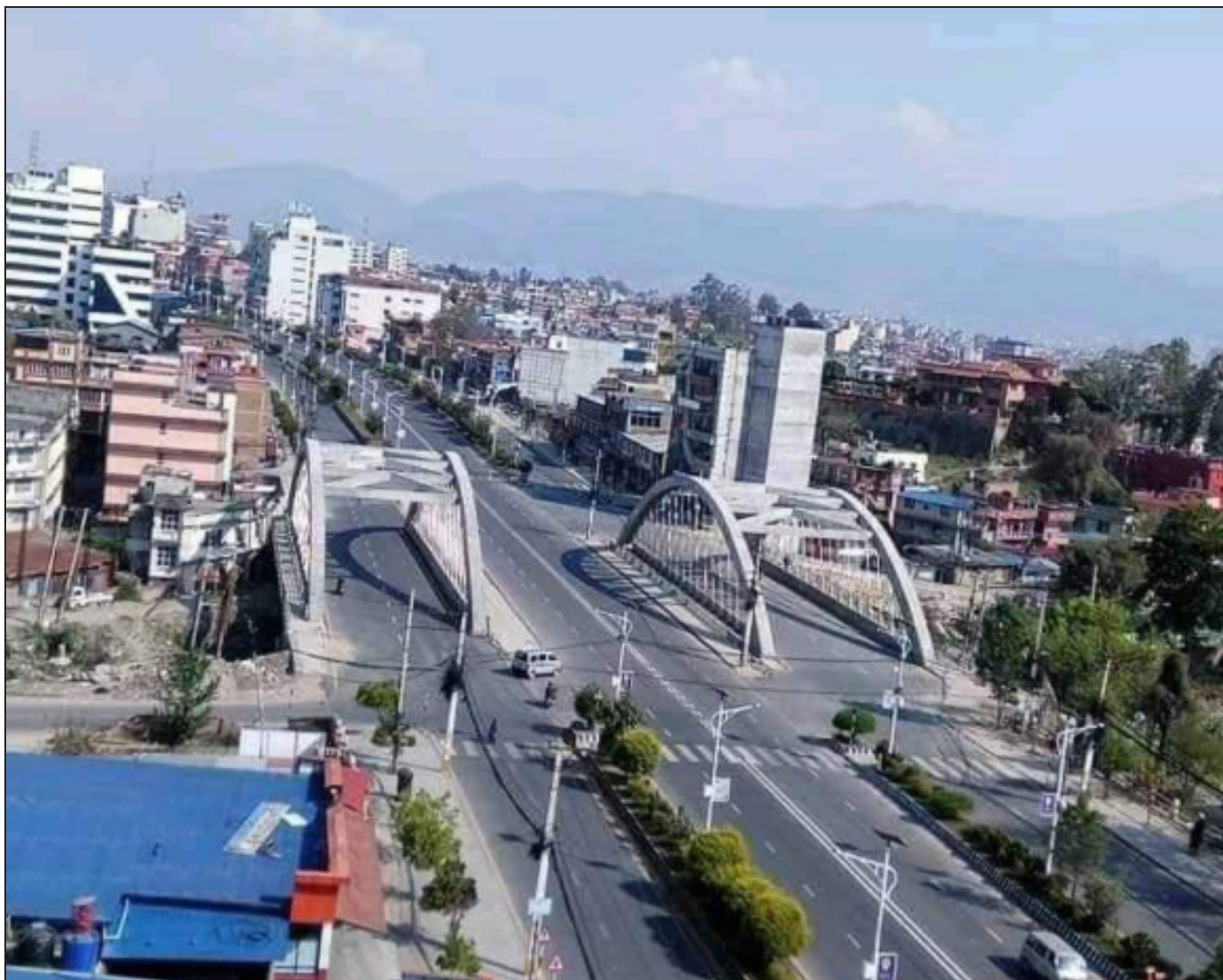
Dhobikhola Network Arch Bridge, Kathmandu (50m span)
