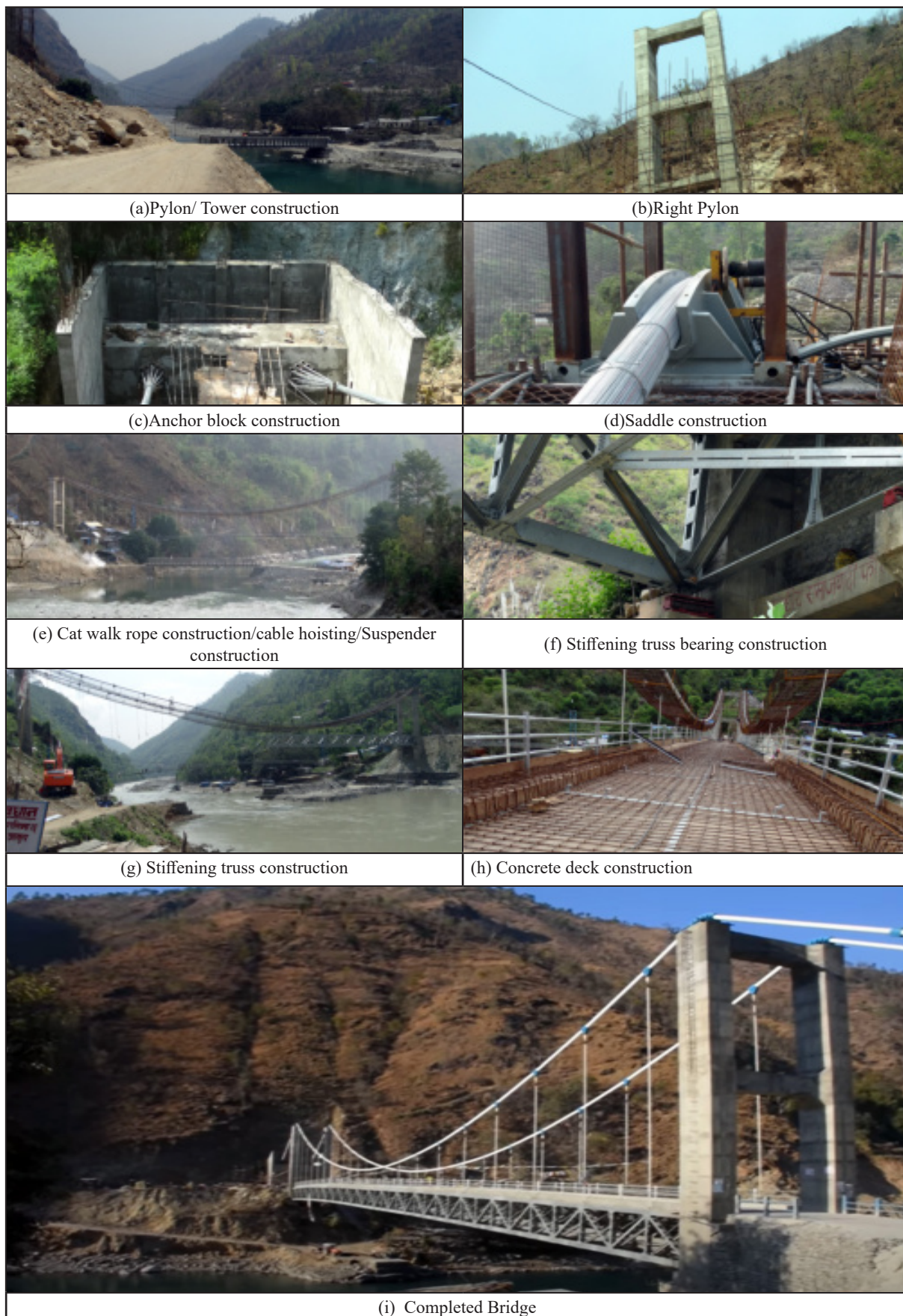
Fig.4- Bridge Construction Sequence
