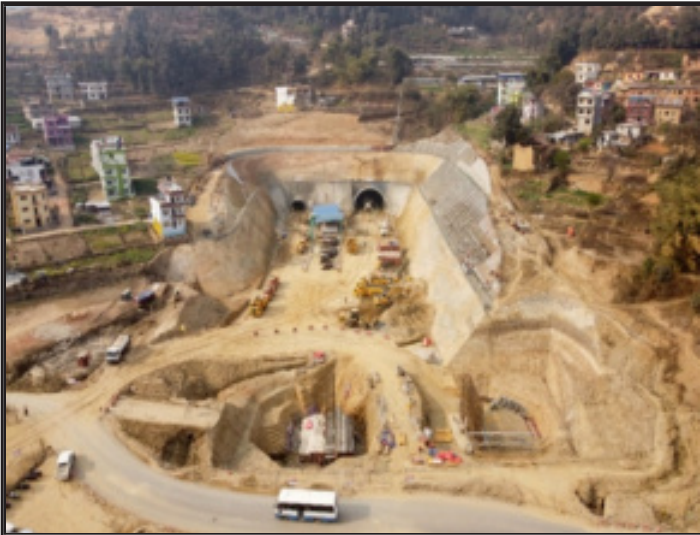
(a) Main Tunnel, East
