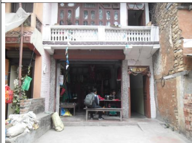
ID-41:Affected Structure of Guna Raj Tripathi (55+355)
