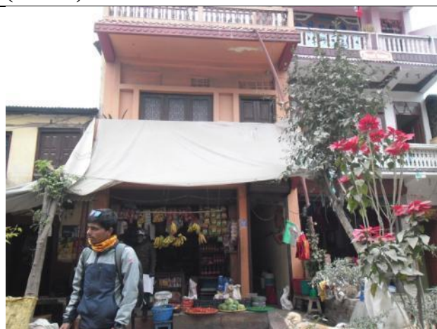
ID-42:Affected Structure of Sita Devi KC (55360)
