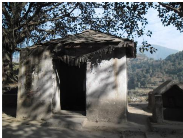
Project Affected Shivaparbati Temple at Koirale (12+300)
