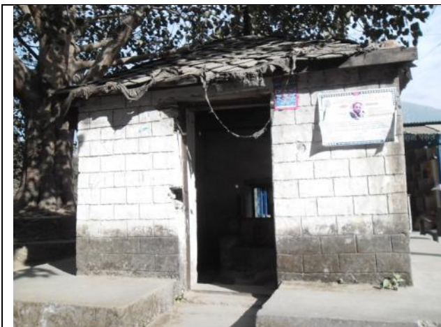
Project Affected Radhakrishna Temple at Koirale (12+300)
