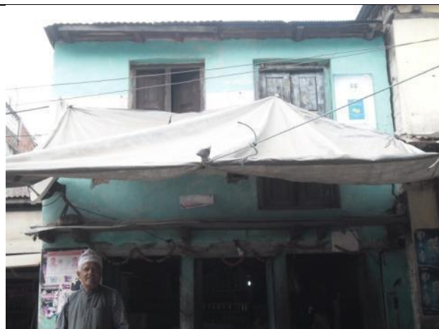
ID-44:Affected Structure of Ram Chandra Tripathi (55+370)
