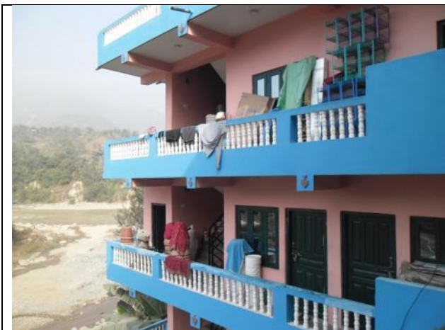
ID-48:Affected Structure of Gobinda Bhadur Baniya (55+395)
