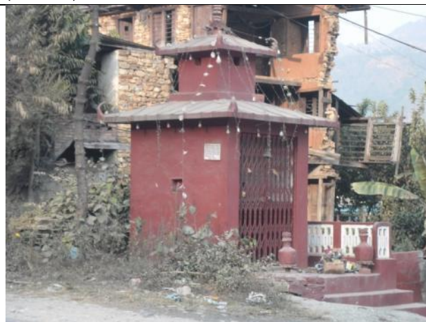
Project Affected Temple at Malekhu (44+050)
