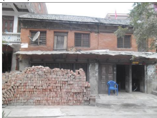
ID-40:Affected Structure of Puran Kumar Lohani (55+350)
