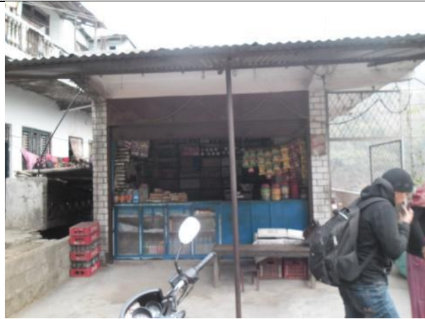
ID-25:Affected Structure of Subba Ramtel (25+000)
