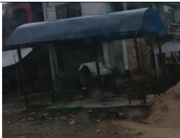
Project affected waiting shed at Maheshdobhan (25+000)
