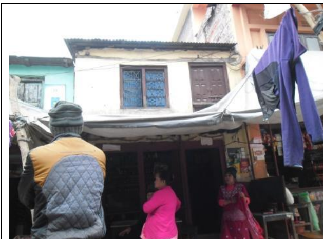
ID-43:Affected Structure of Suk Maya Magar (55+365)
