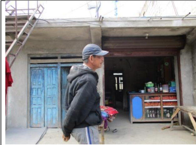
ID-60:Affected Structure of Hom Bahadur Magar (61+900)
