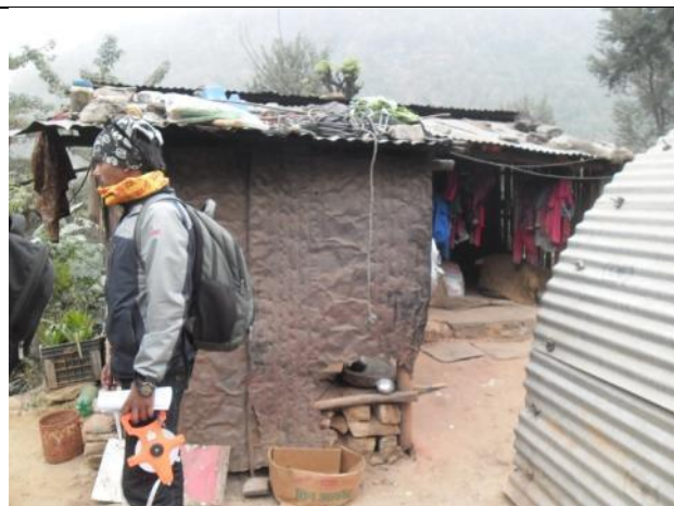
ID-38:Affected Structure of Bal Bahadur Praja (50+100)
