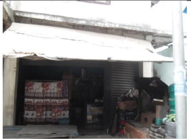
ID-26:Affected Structure of Devi Bahadur Malla (25+000)
