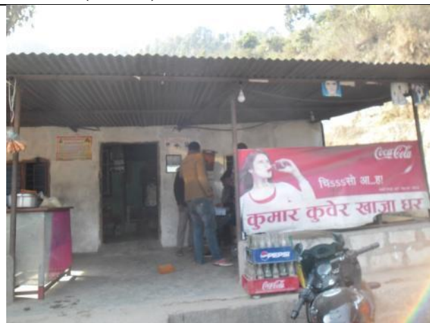
ID-17: Affected Structure of Keshav Lamichhane (19+550)
