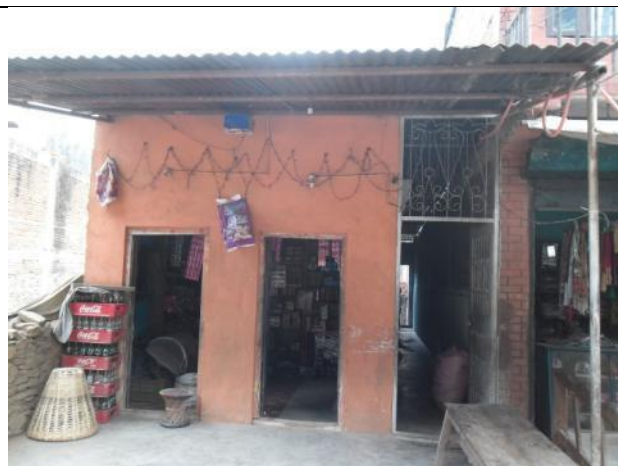
ID-28:Affected Structure of Shiva Ramtel (25+000)
