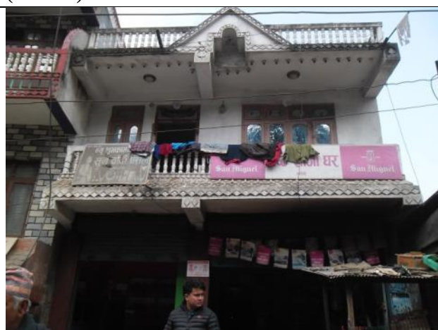
ID-46:Affected Structure of Bishnu Shrestha (55+380)
