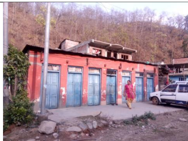
ID-18: Affected Structure of Nyarayan Dahal (23+250)
