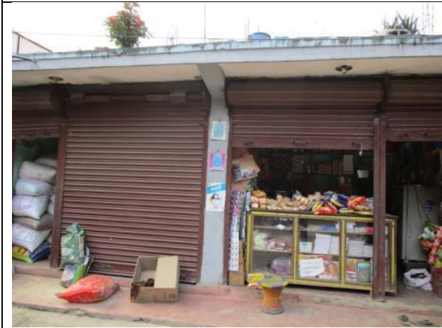
ID-62:Affected Structure of Krishna Prasad Dallakoti (61+900)
