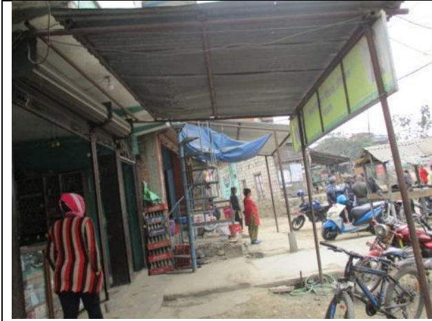
ID-77:Affected Structure of Raj Kumar Gurung (73+580)
