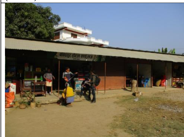
ID-56:Affected Structure of Krishna Prasad Thapaliya (58+400)
