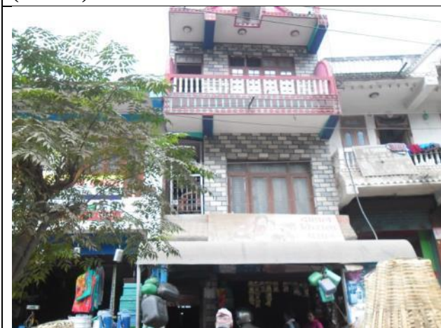
ID-47:Affected Structure of Dipendra Dahal (55+385)
