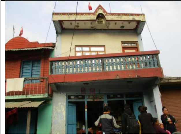
ID-64:Affected Structure of Gyan Bahadur Shrestha (62+000)
