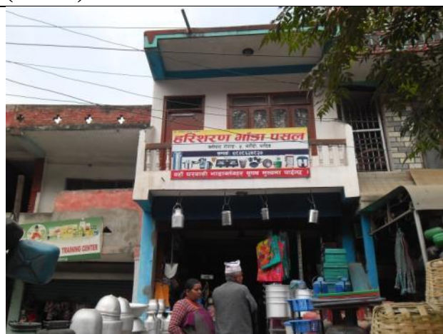
ID-48:Affected Structure of Gobinda Bhadur Baniya (55+390)
