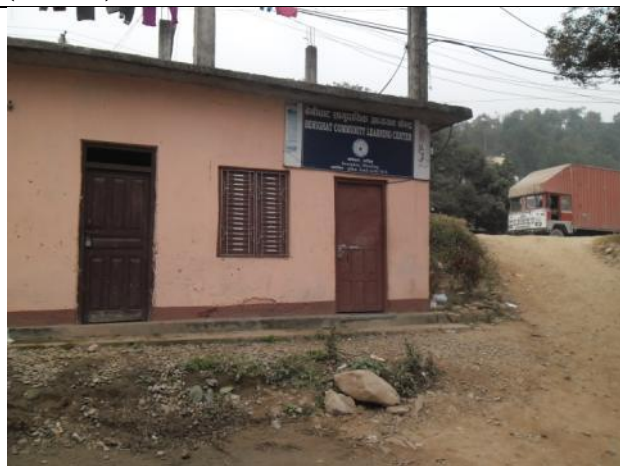
Project Affected Community Building at Benighat (50+900)
