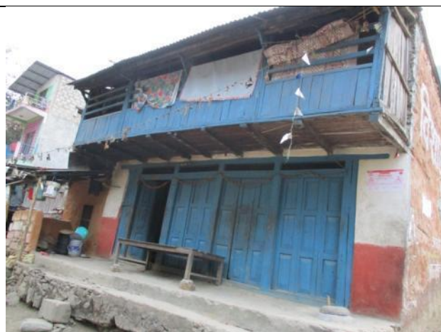
ID-73:Affected Structure of Insan Gurung (62+100)
