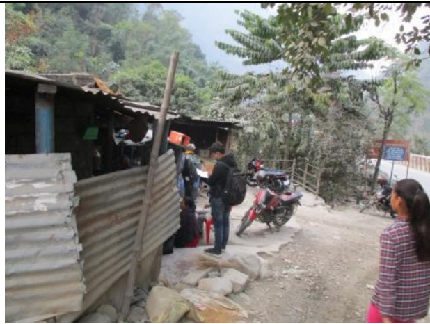
ID-73:Affected Structure of Insan Gurung (62+100)
