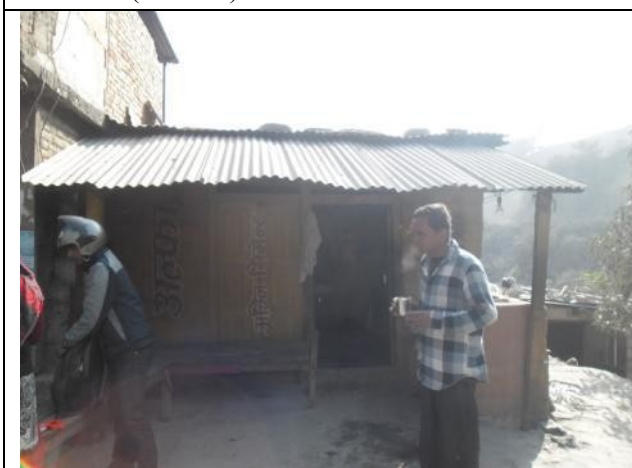
ID-29: Affected Structure of Gopal Bahadur Adhikari (26+000)
