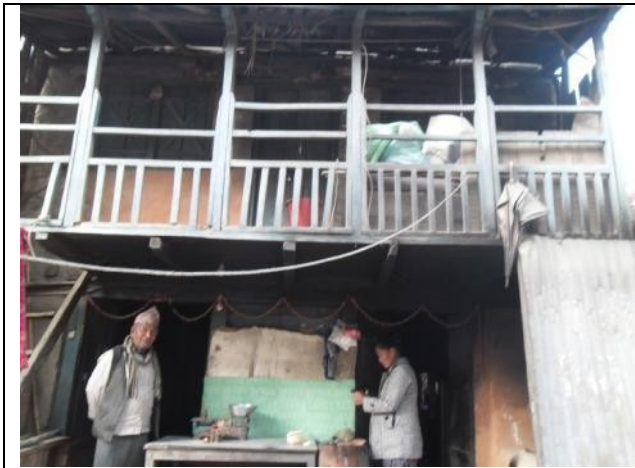
ID-21:Affected Structure of Bir Bhadur Tamang (25+000)
