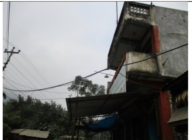
ID-76:Affected Structure of Talsa Bhujel (73+570)
