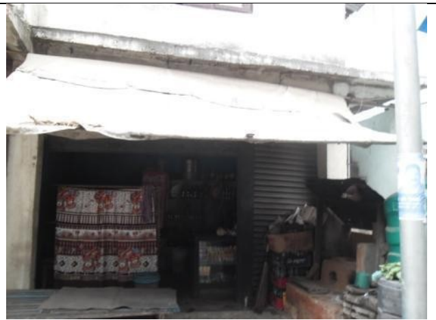
ID-26:Affected Structure of Devi Bahadur Malla (25+000)
