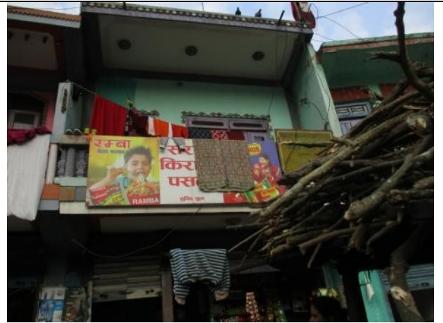
ID-67: Affected Structure of Mahendra Puri (62+050)
