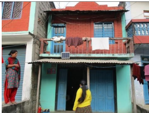
ID-65:Affected Structure of Dil Maya Ghale (62+050)
