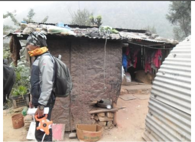
ID-38:Affected Structure of Bal Bahadur Praja (50+100)
