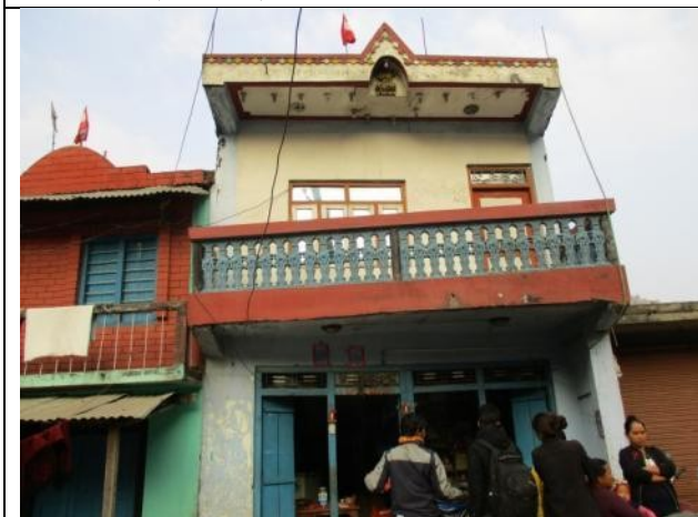
ID-64:Affected Structure of Gyan Bahadur Shrestha (62+000)
