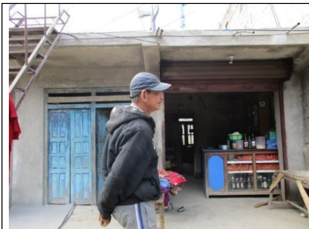
ID-60:Affected Structure of Hom Bahadur Magar (61+900)
