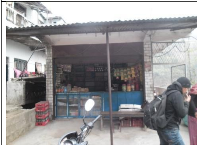
ID-25:Affected Structure of Subba Ramtel (25+000)
