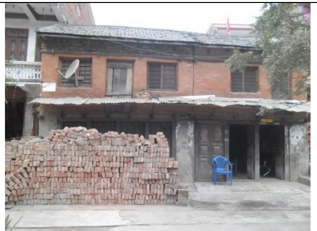
ID-40:Affected Structure of Puran Kumar Lohani (55+350)
