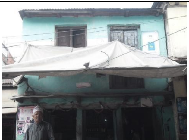
ID-44:Affected Structure of Ram Chandra Tripathi (55+370)
