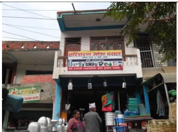
ID-48:Affected Structure of Gobinda Bhadr Baniya (55+390)
