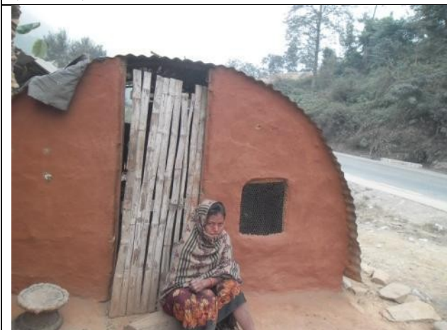
ID-36:Affected Structure of Sete Praja Chepang (50+100)
