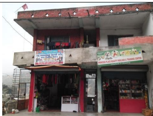
ID-49: Affected Structure of Tulasi Prasad Sual (55+400)
