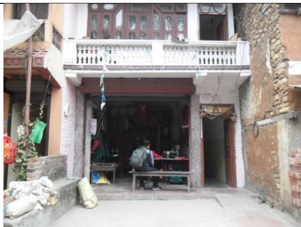
ID-41:Affected Structure of Guna Raj Tripathi (55+355)
