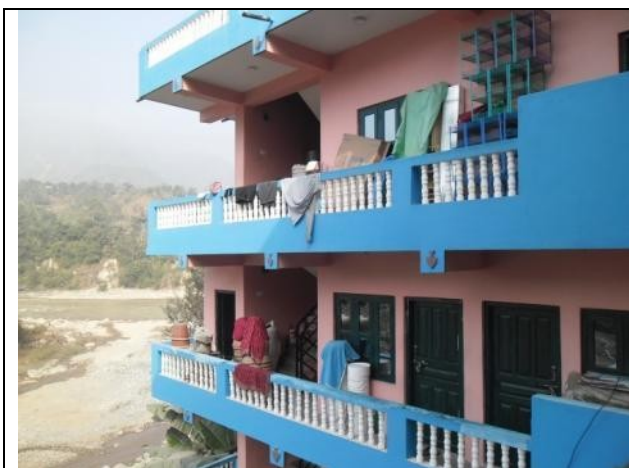
ID-48: Affected Structure of Gobinda Bhadur Baniya (55+395)
