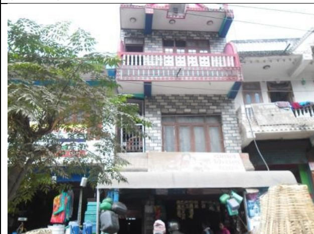
ID-47:Affected Structure of Dipendra Dahal (55+385)
