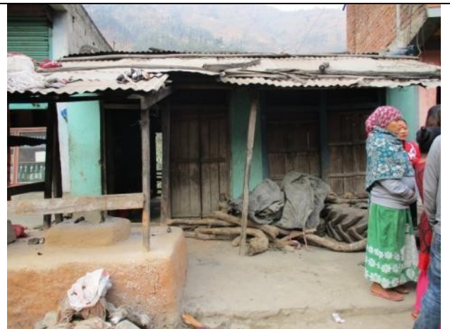
ID-69: Affected Structure of Dil Maya Chepang (62+100)
