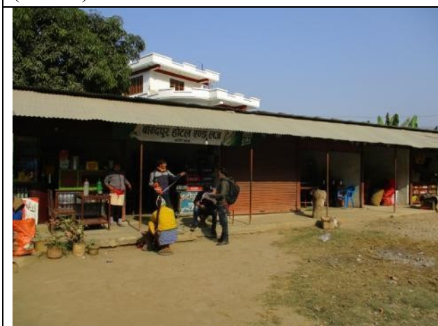
ID-56: Affected Structure of Krishna Prasad Thapaliya (58+400)
