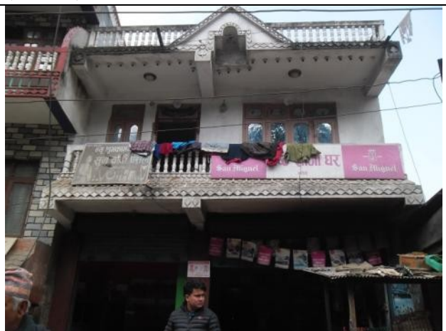
ID-46:Affected Structure of Bishnu Shrestha (55+380)
