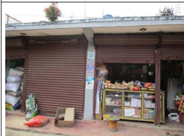
ID-62:Affected Structure of Krishna Prasad Dallakoti (61+900)
