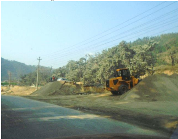
Crusher plant established close to highway at Galchi
