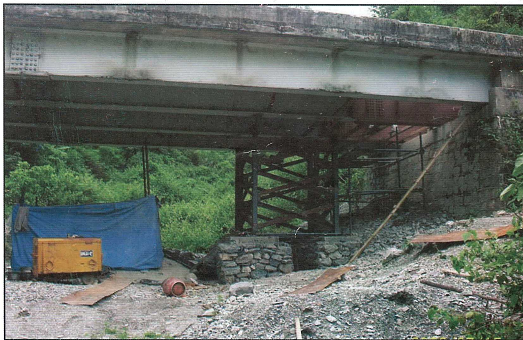
Staging for repair works
