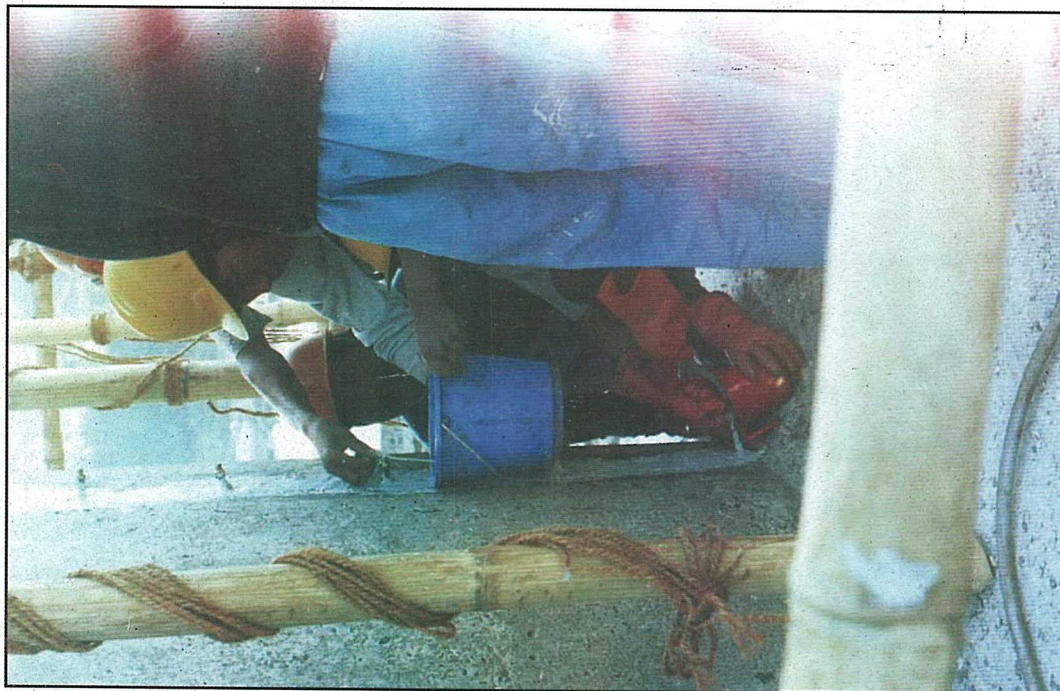
Photo 9: Crack Sealing on the Pier of Tamor Bridge : The scaffolding and sealing work
