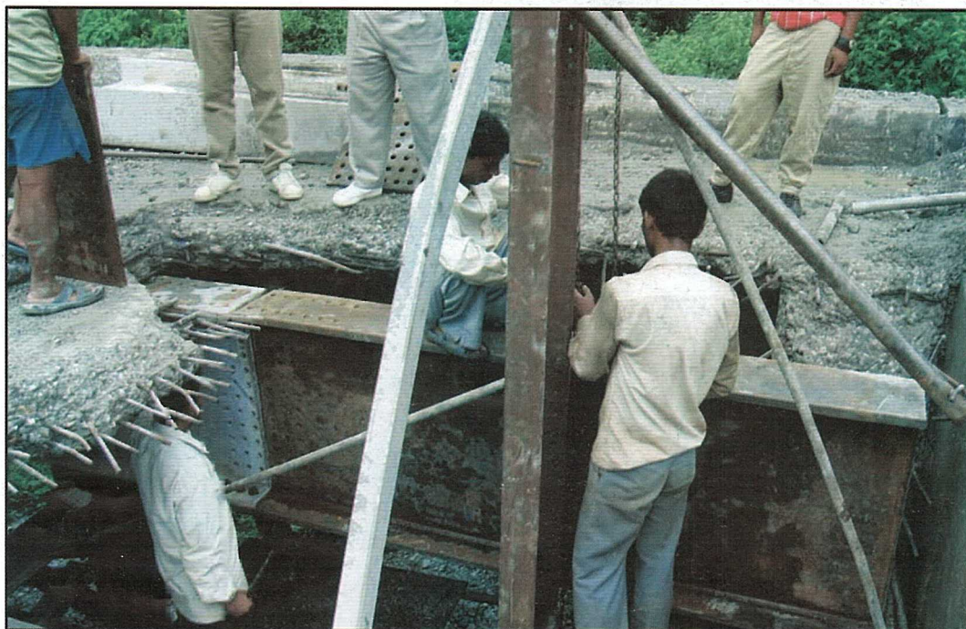
Lowering and Position of new girder section
