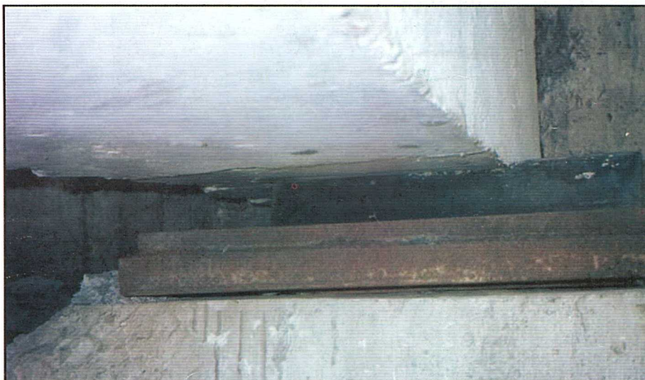
Photo 5-8: Some Minor Works needed at Expansion joint and bearings
