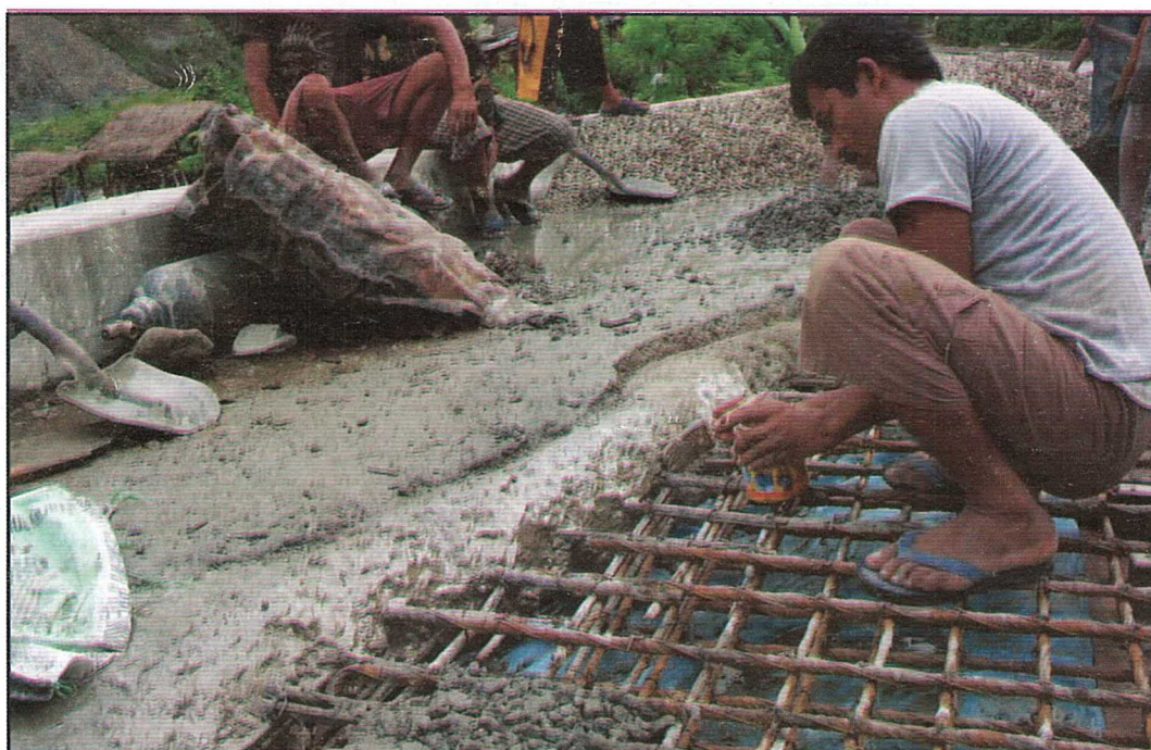
Fixing of reinforcement and concreting
