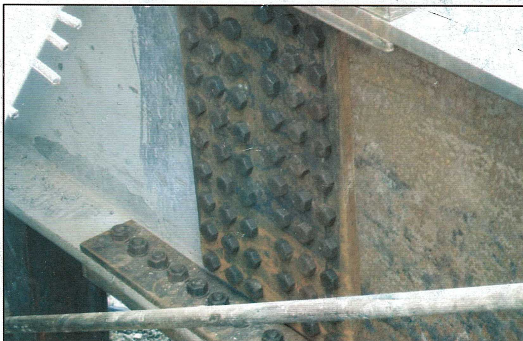
Fixing the new girder section with old girder
