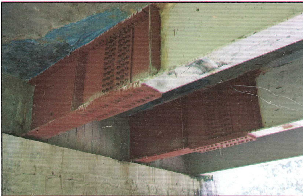
Two out of three girders are repaired
