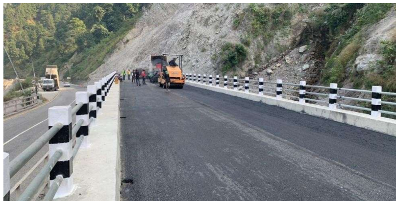
Figure 4 – Namsi Bridge, Chitwan
